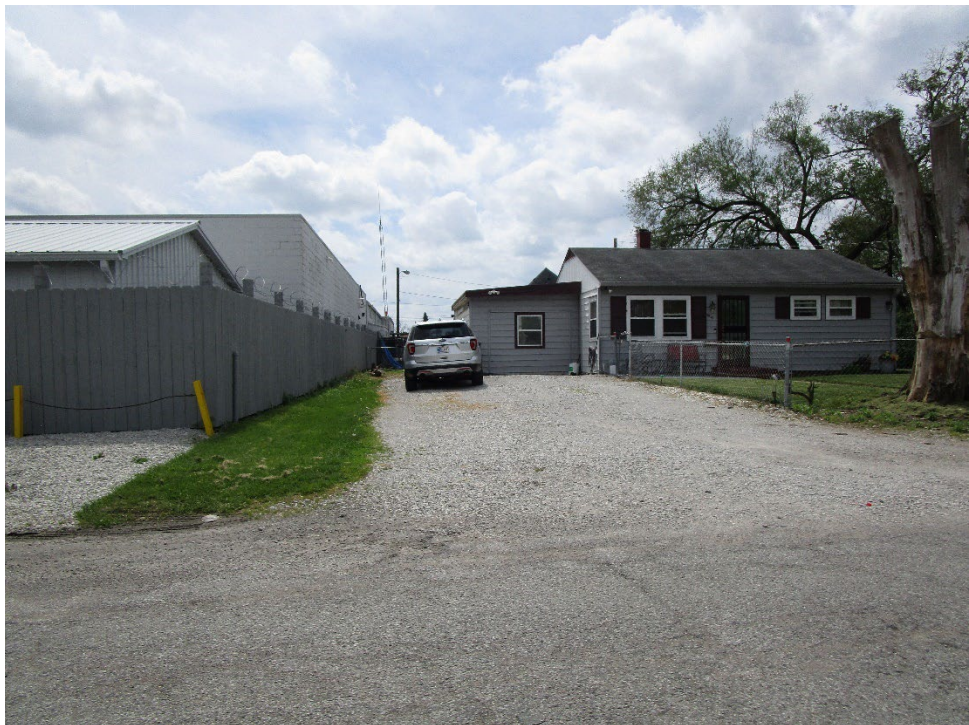
View of site and adjacent residence looking south across West 17th Street
