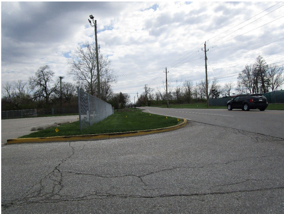
View looking south along South Franklin Road
