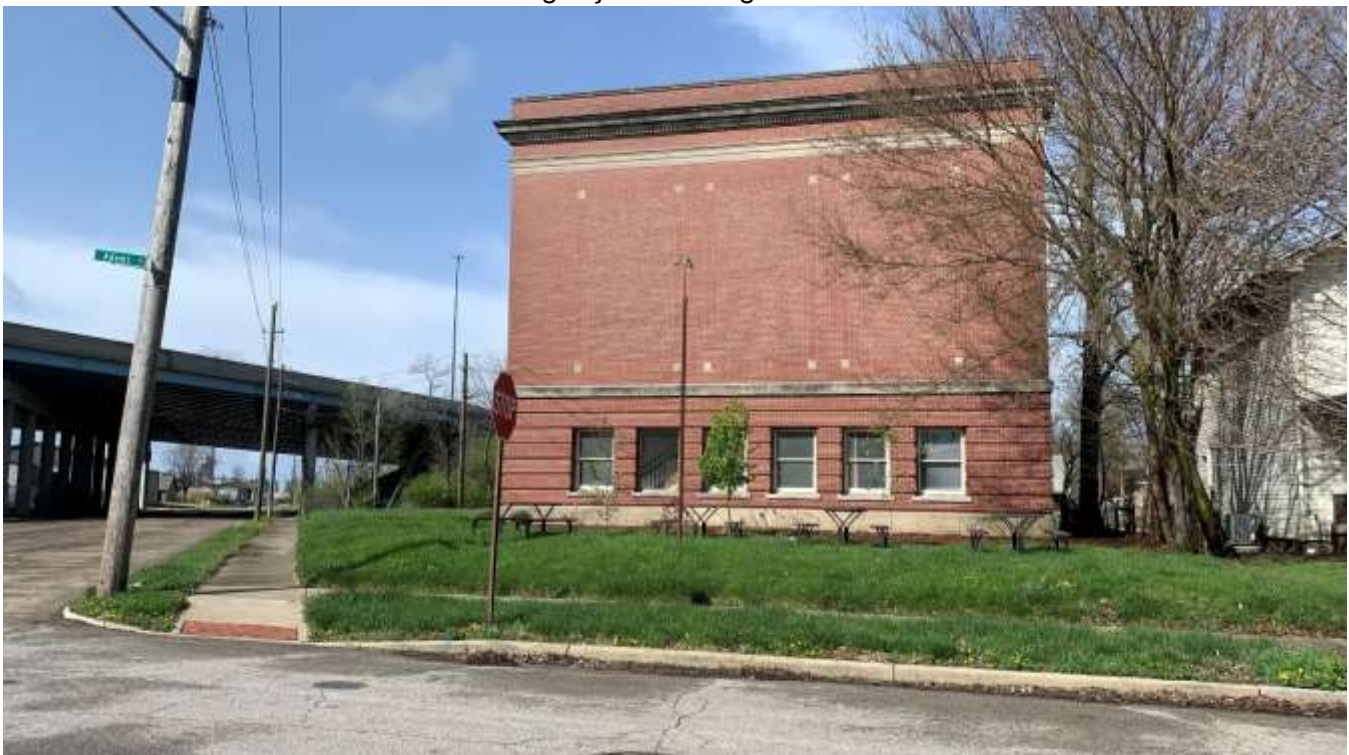
Photo of the eastern building façade looking southwest along Roosevelt Avenue.
