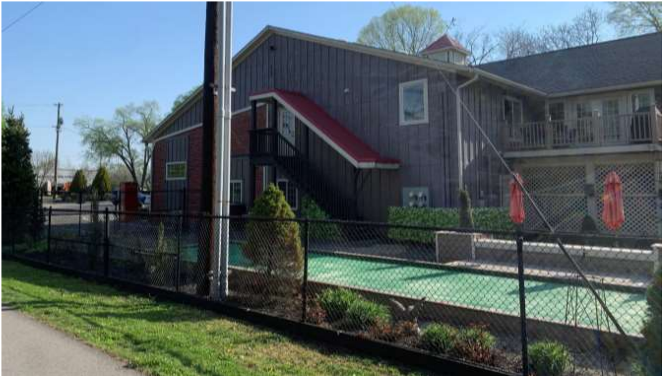
Photo of the west building façade and entrance to one of the units upstairs.
