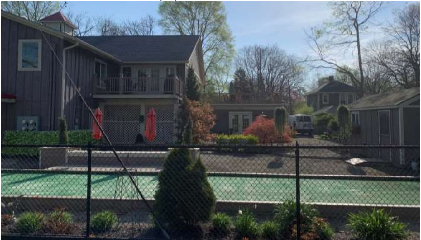
Photo of the rear yard and other units at the rear.
