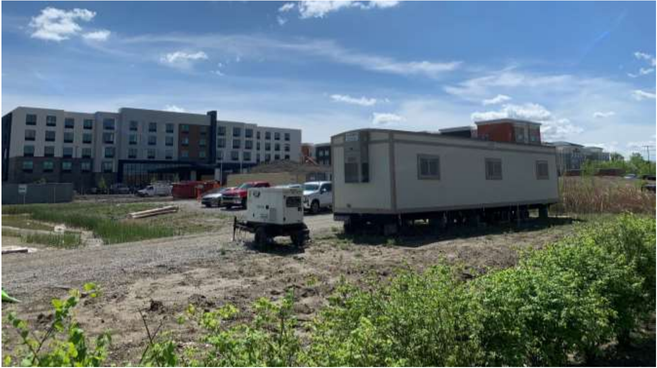
Photo of the subject site looking southeast.
