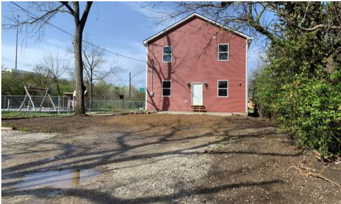
Photo of the rear yard of 2255 North LaSalle Street.
