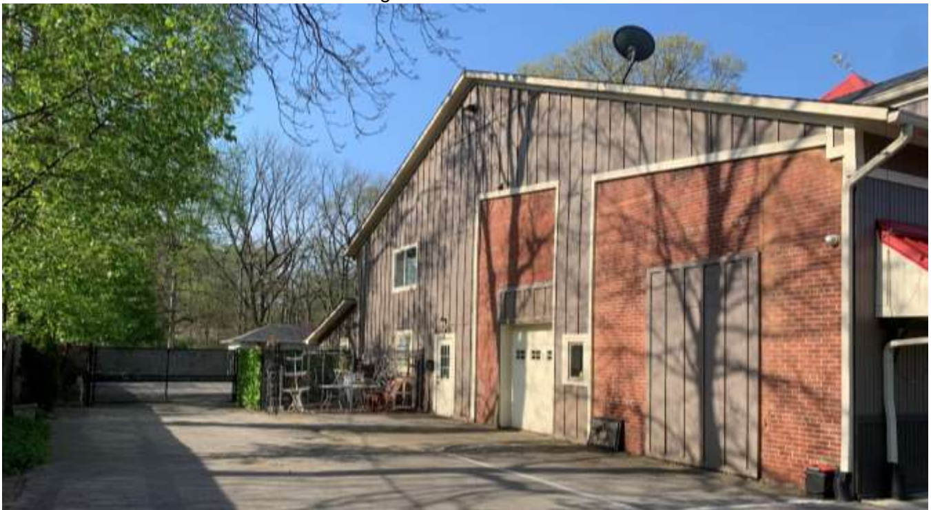
Photo of the east building façade.
