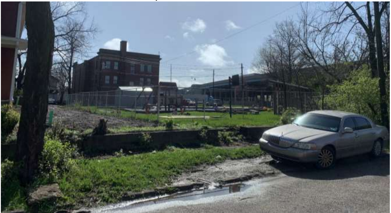
Photo of the subject site at 3350 Roosevelt Avenue with a playground.
