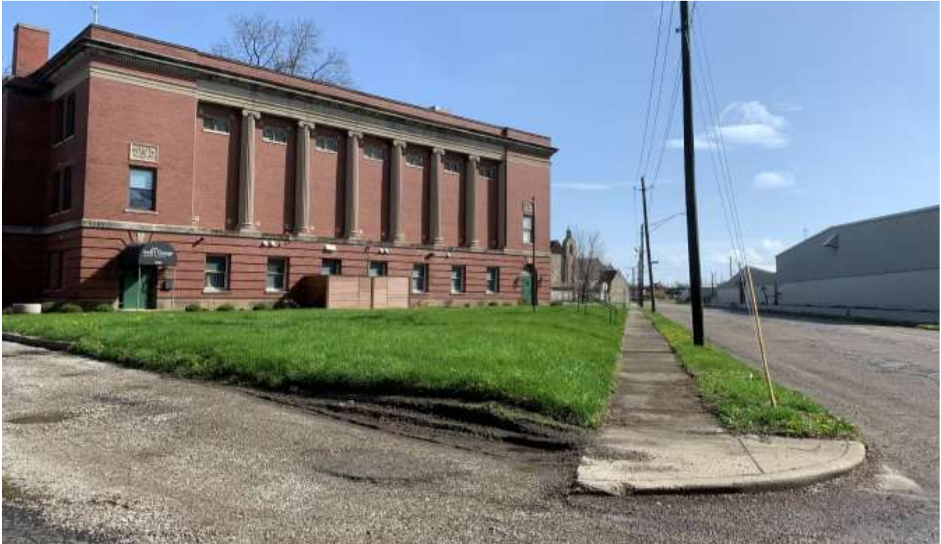
Photo of the southern building façade looking northeast on Roosevelt Avenue.
