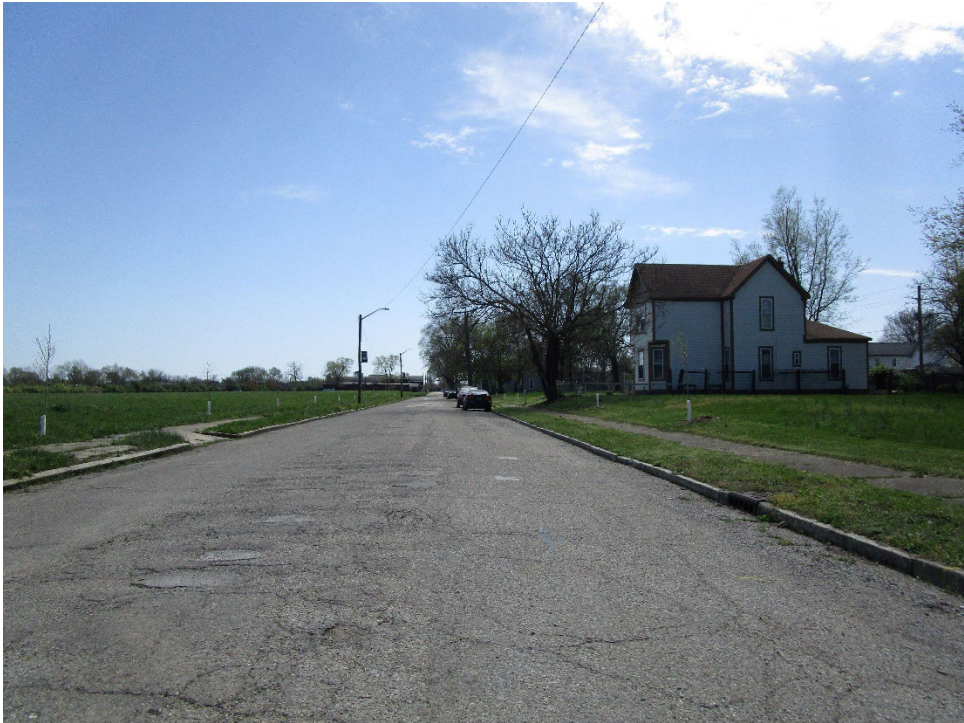
View looking south along Winthrop Avenue
