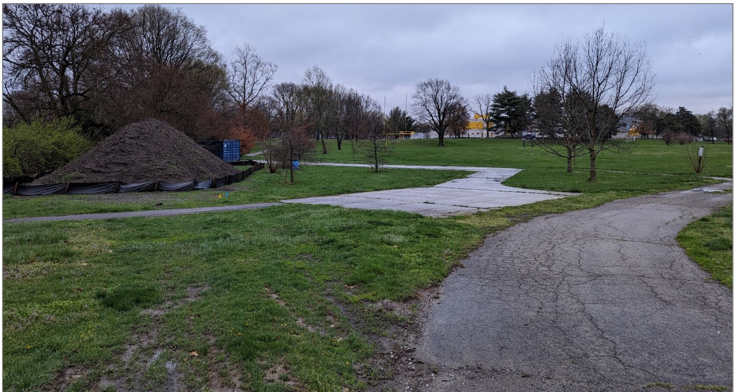
Site photo – northern area of improvements
