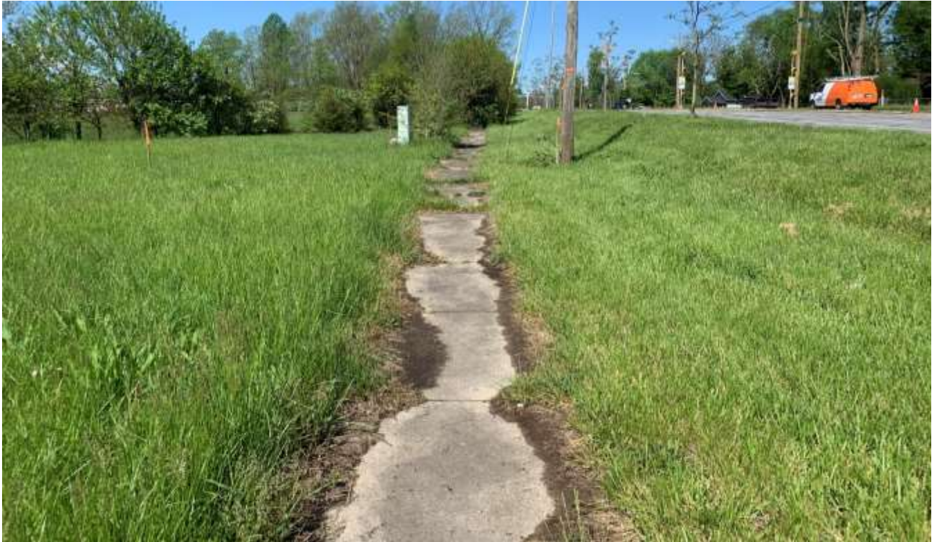
Photo of the existing sidewalk along Raymond Street looking west.
