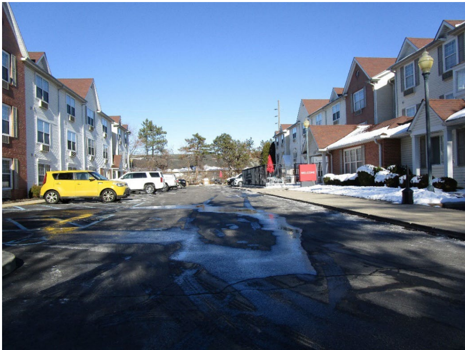
View of site looking north at parking between the two buildings
