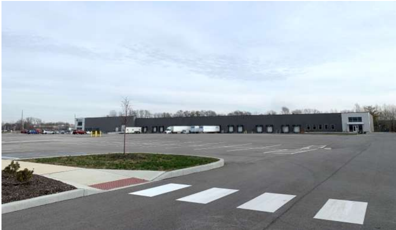
West building façade of Building 2 looking east.
