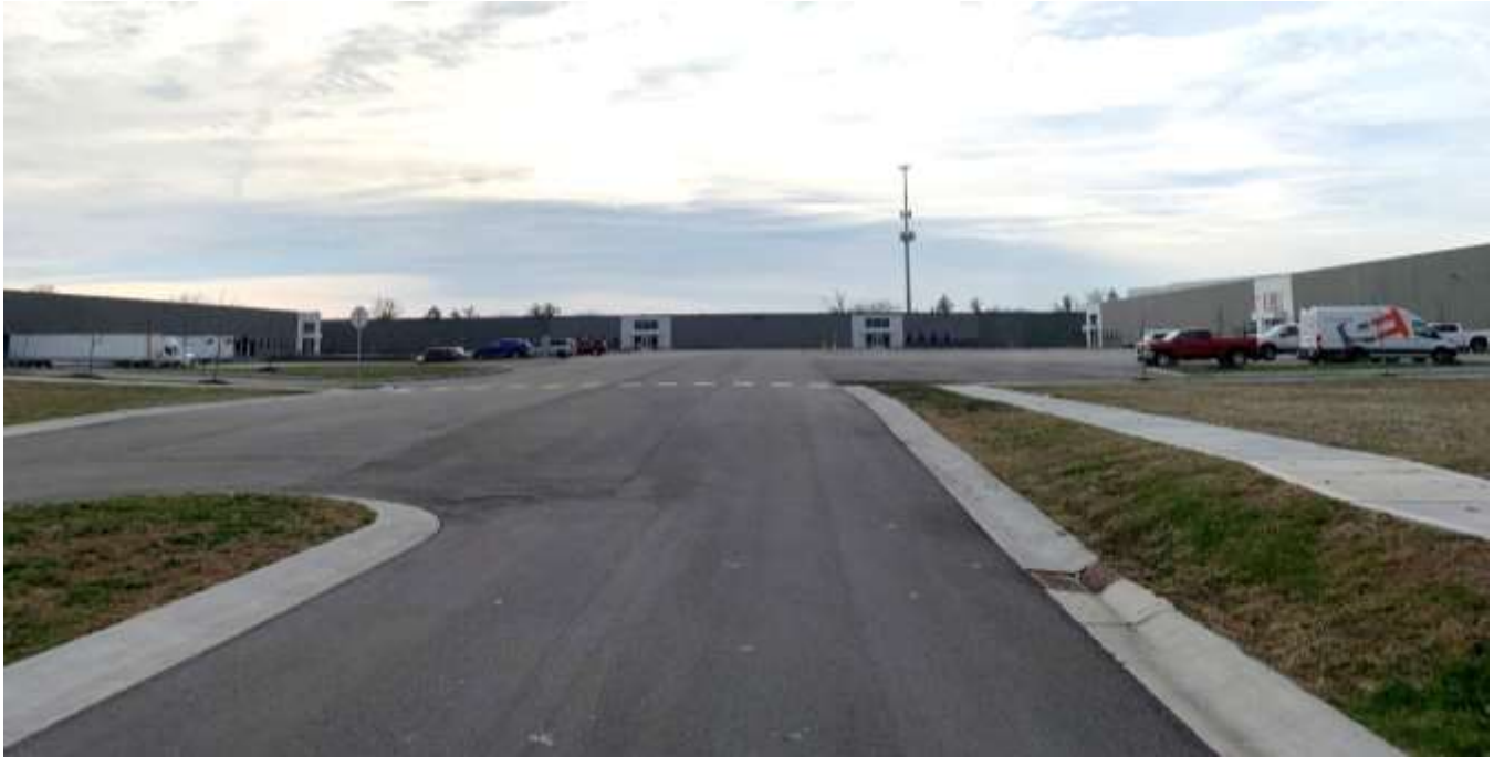
Photo of Building 1 looking south.
