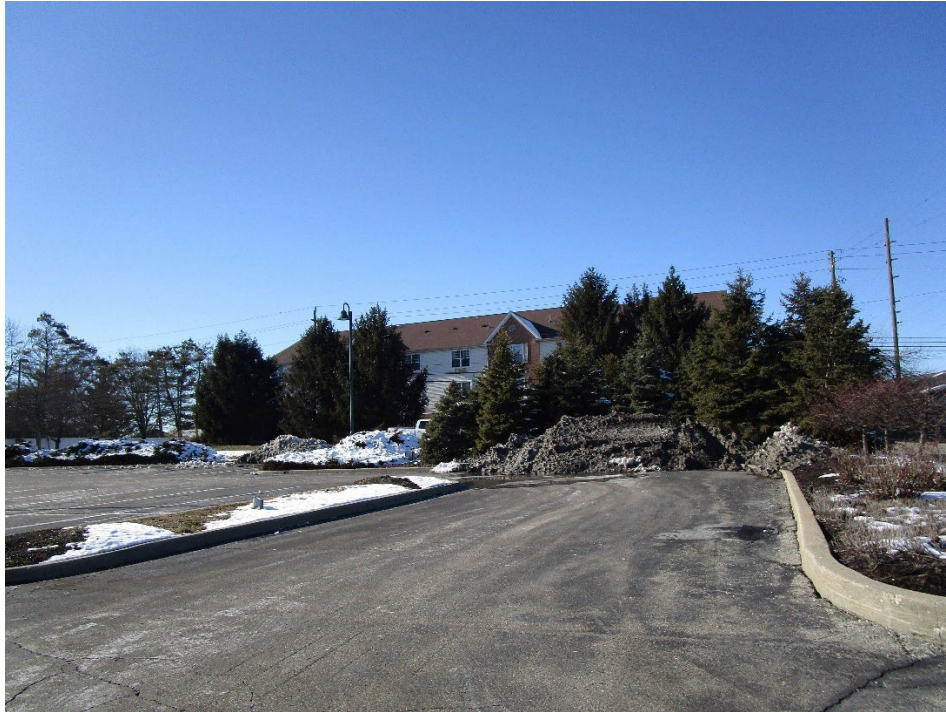
View of site looking west across parking lot located east of site
