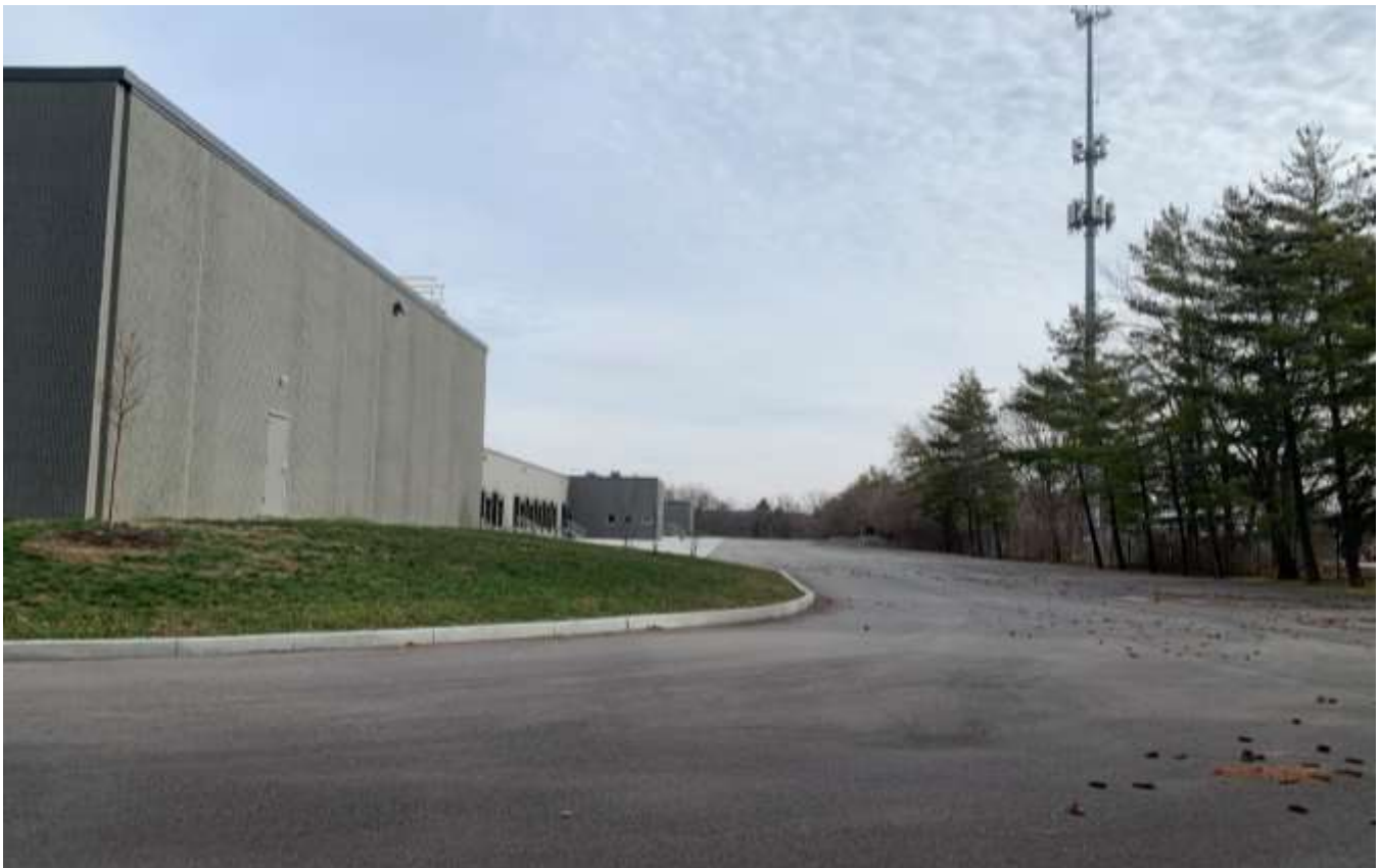
Rear view of Building 1 looking east along the southern property boundary.
