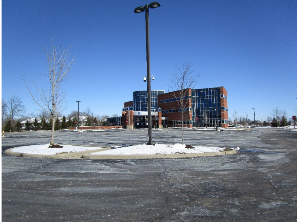
View of site looking east
