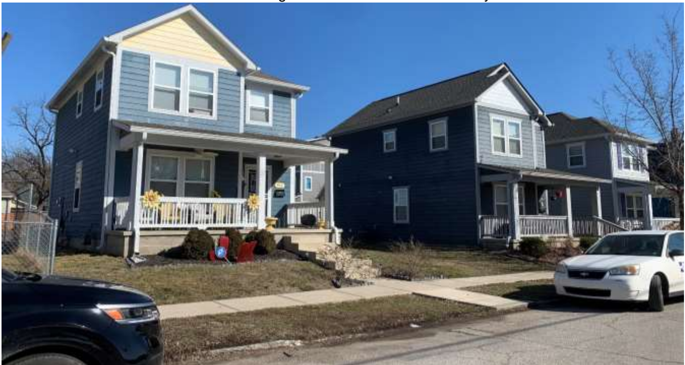
Photo of the dwellings east of the site.
