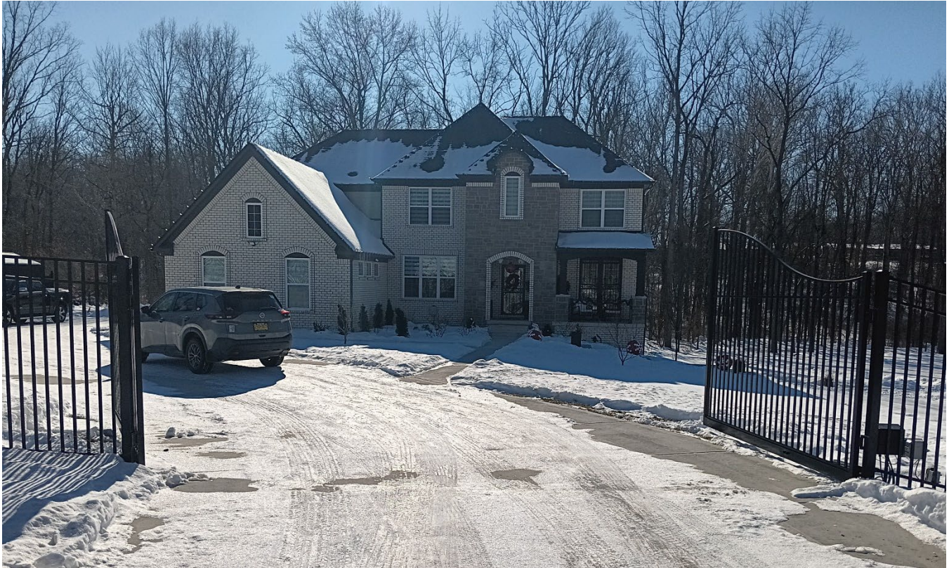
Exhibit 5: The primary structure at 4235 East 46 th Street.
