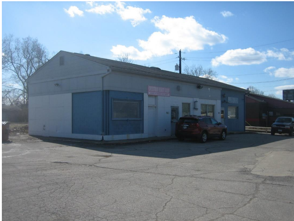
Photo of adjacent commercial property to the north, looking southwest.
