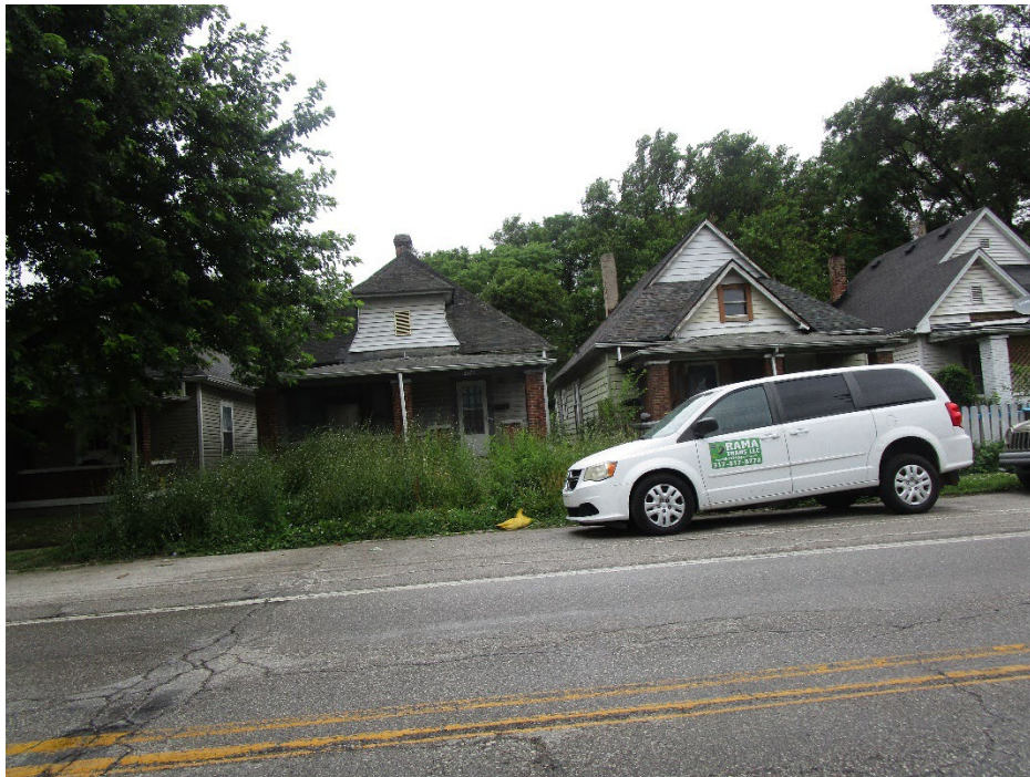
View of adjacent properties to the east of site looking north across Prospect Street
