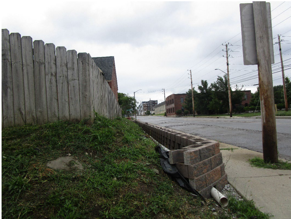
View looking east from north / south alley
