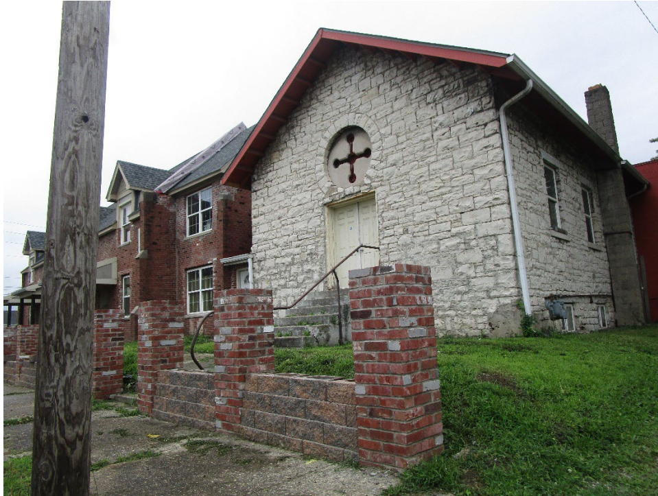
View of site looking southwest
