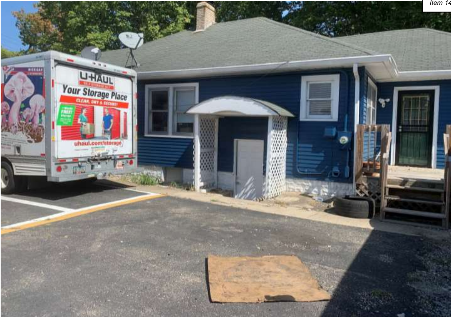
Photo of the western office façade.
