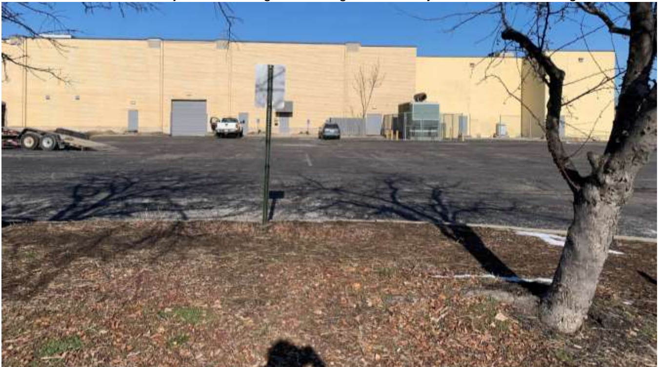
Photo of the subject site looking west at the existing building.
