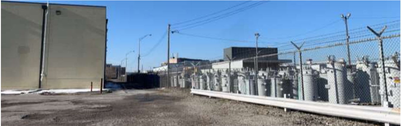
Photo of the industrial property north of the subject site.
