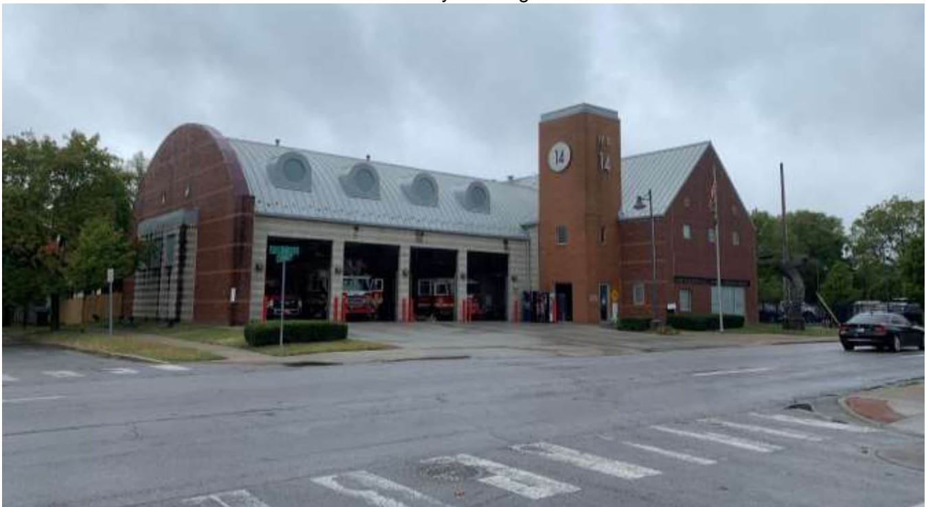
Photo of the fire station south of the site.
