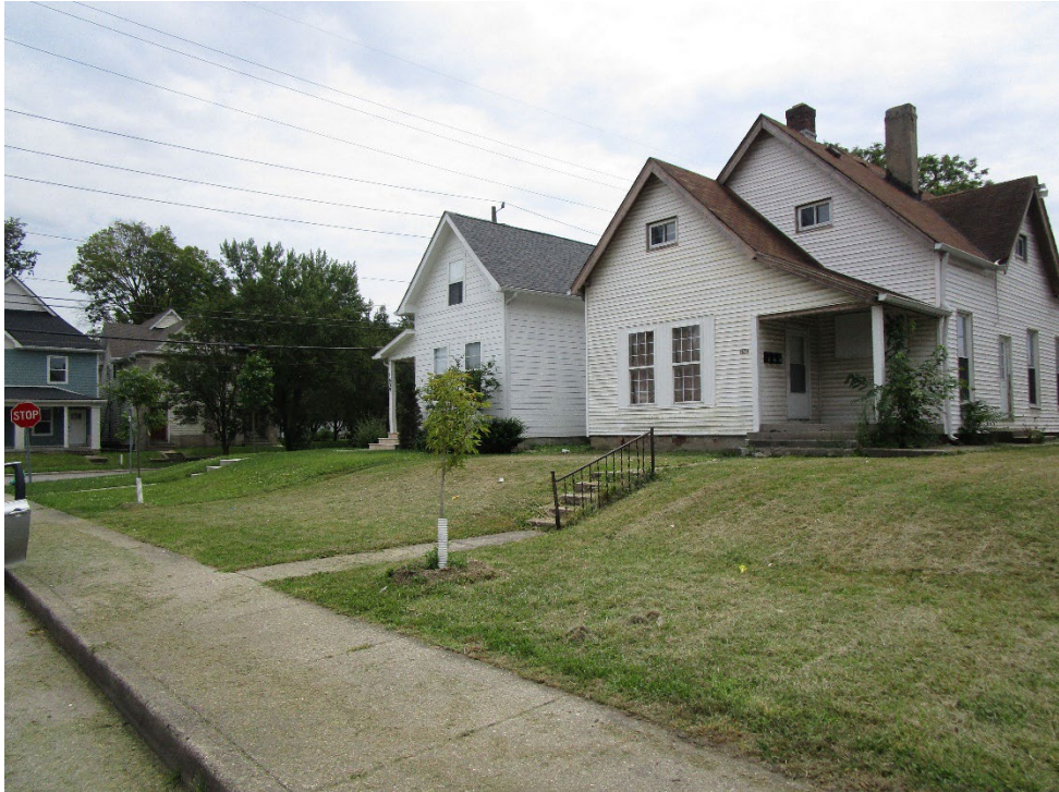
View of existing dwelling (1631 Woodlawn Avenue) looking southeast ac
