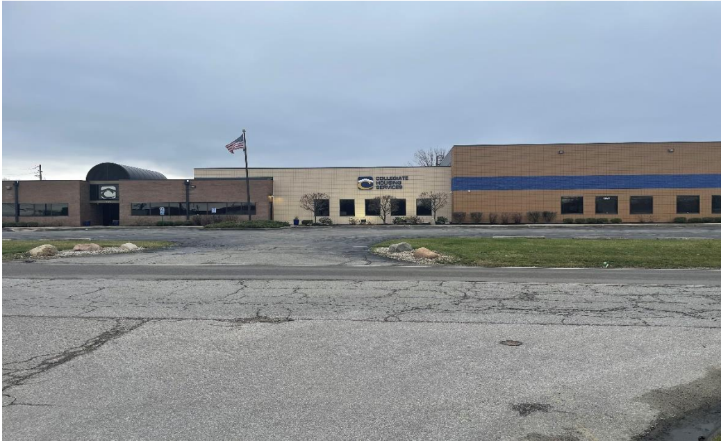
Photo Five: Development Across East 65 th Street, Facing South
