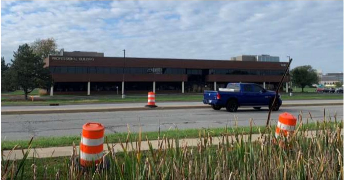
Photo of the northern building façade.
