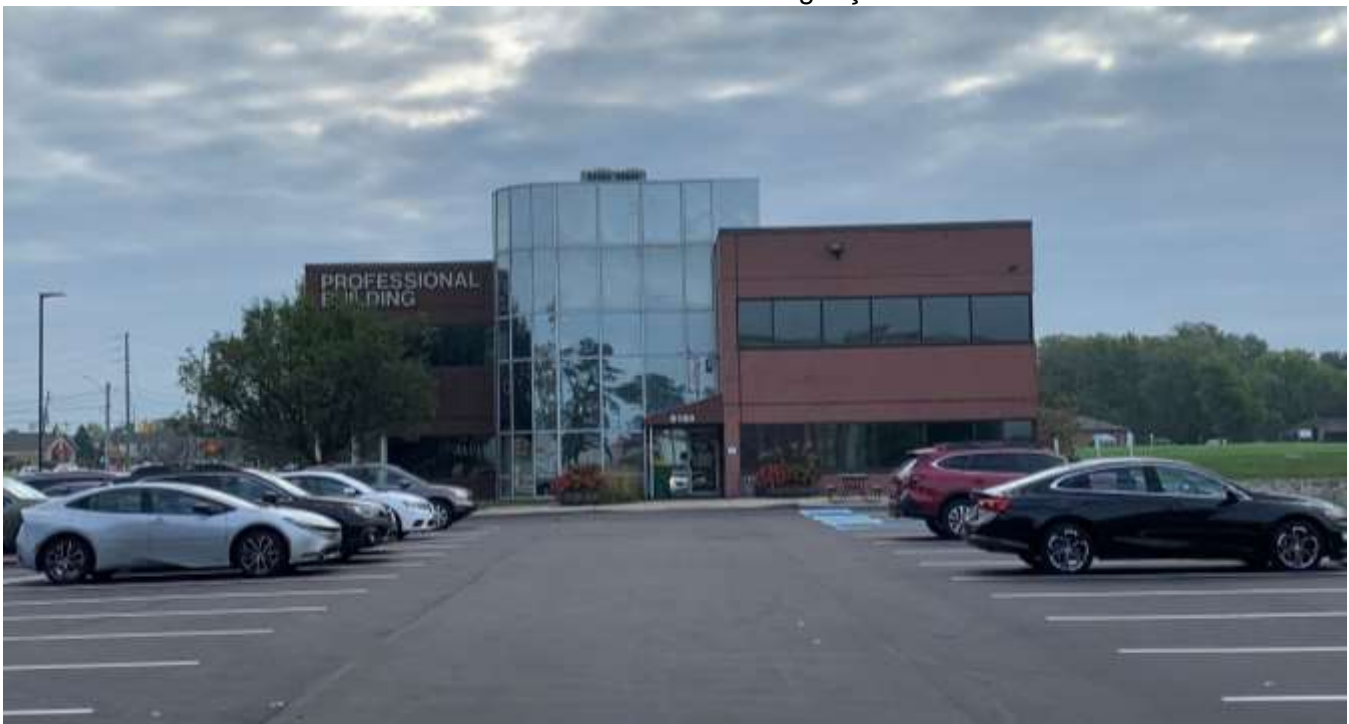
Photo of the western building façade.
