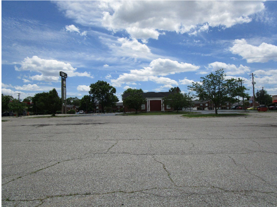
View from site looking south
