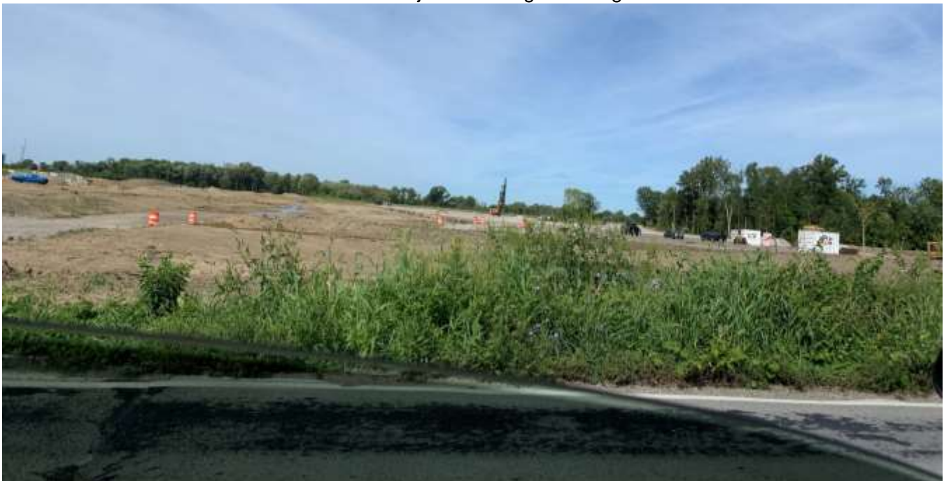
Photo of the subject site looking west from Arlington Avenue.
