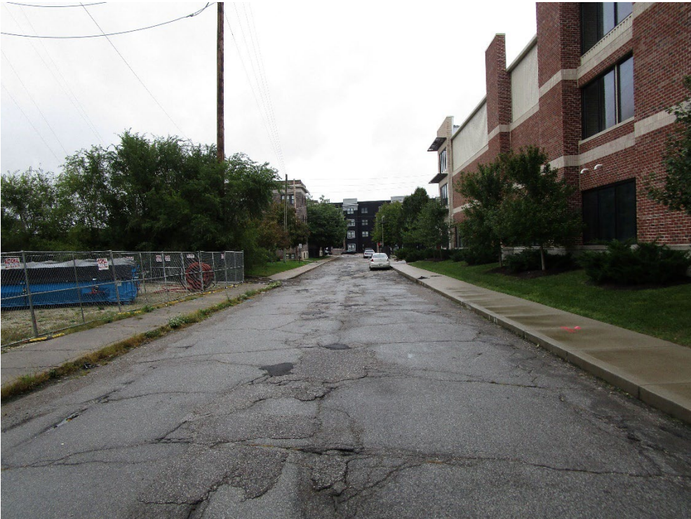
View looking east along Mc Lean Place
