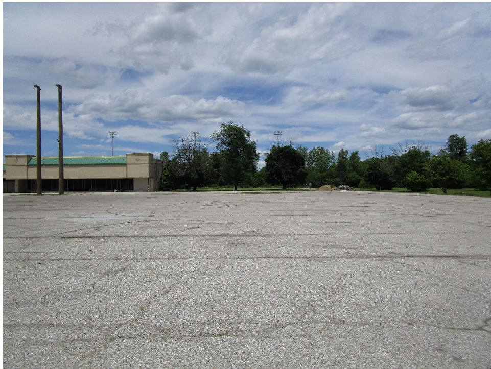
View of site looking north
