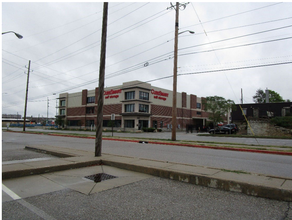
View of site looking northeast across North Illinois Street
