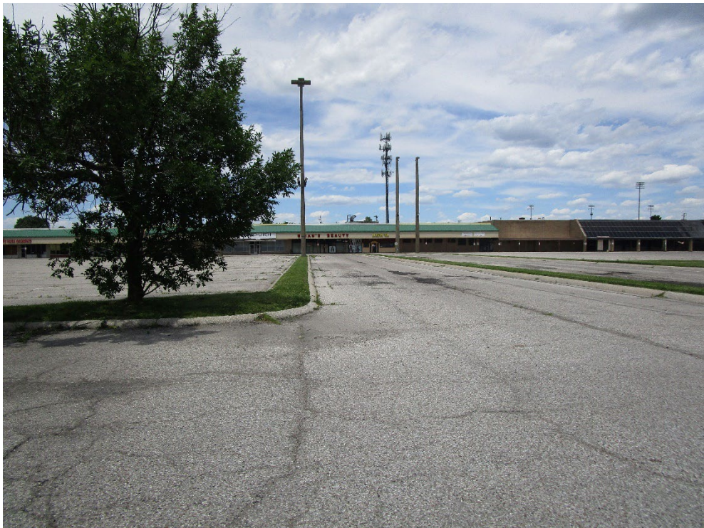
View of site looking north
