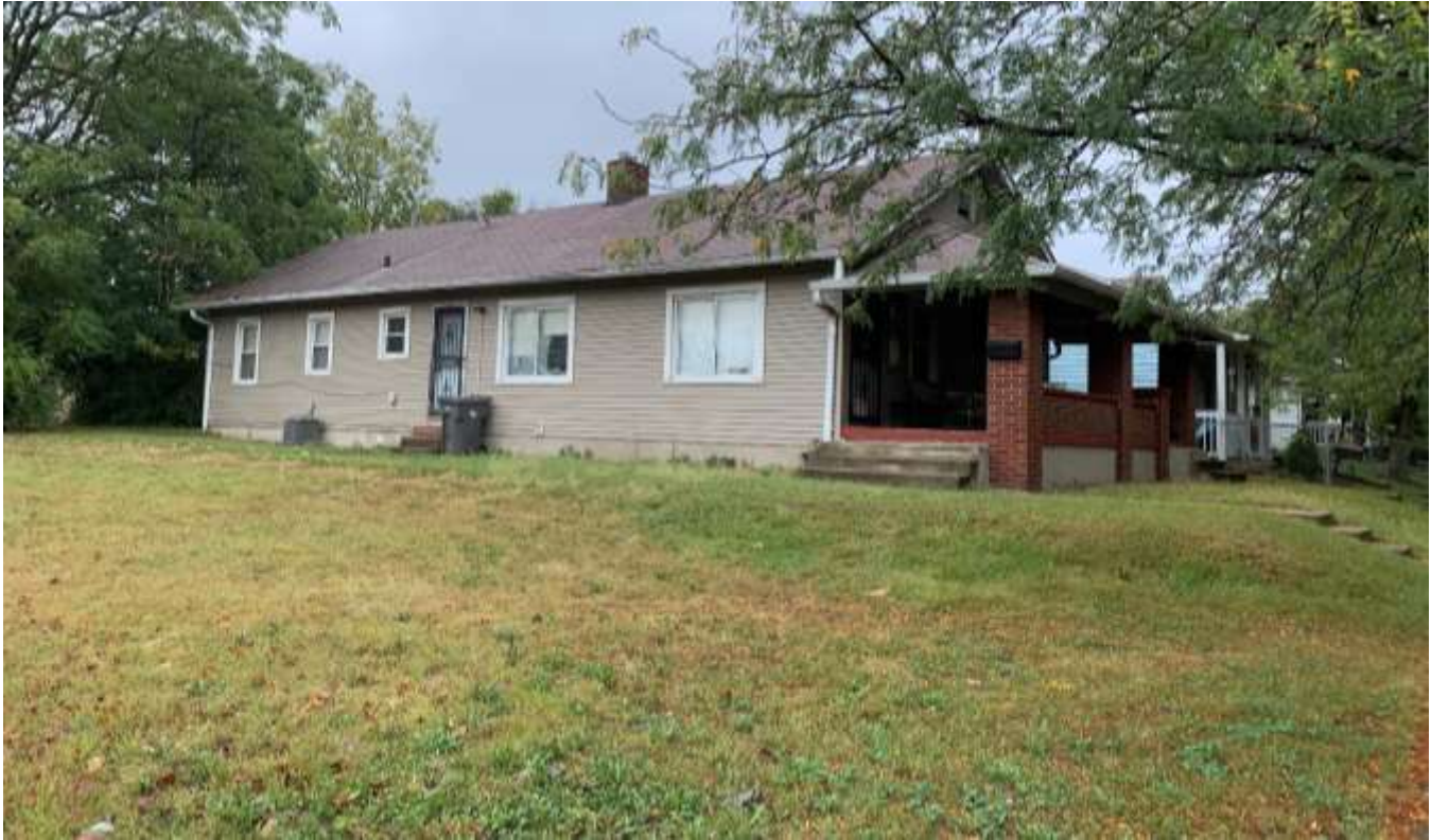
Photo of the two-family dwelling north of the site.
