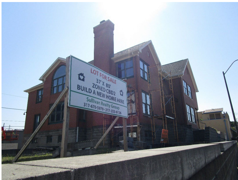
View looking southeast at adjacent two-family dwelling
