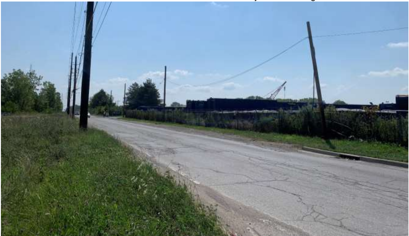
Photo of the subject site street frontage along 21 st Street looking east.
