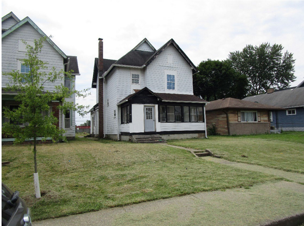
View of existing dwelling (1627 Woodlawn Avenue) looking south
