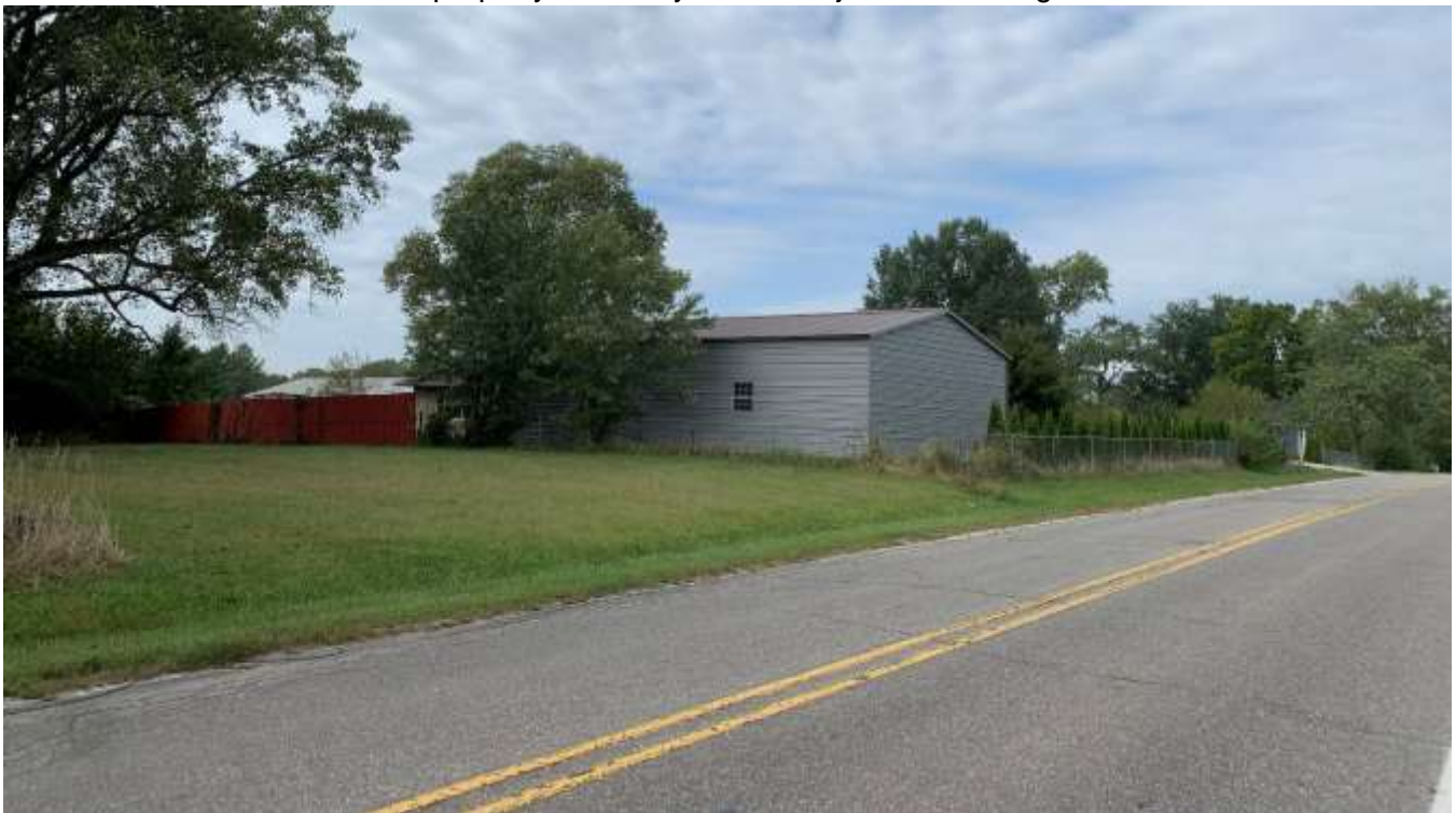
Photo of the single-family dwelling west of the subject site.
