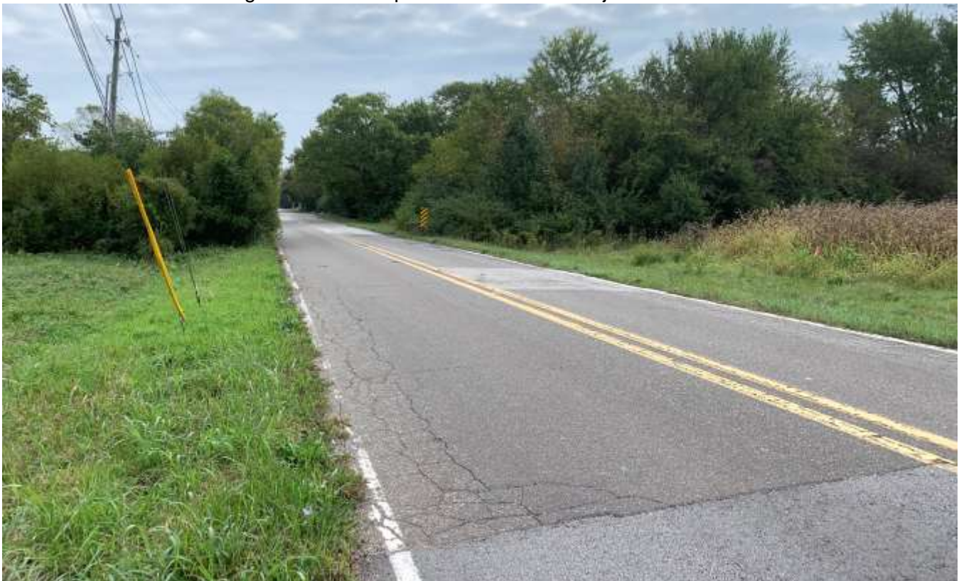
Looking east on Southport Road with the subject site on the right at the northeast corner of the site.
