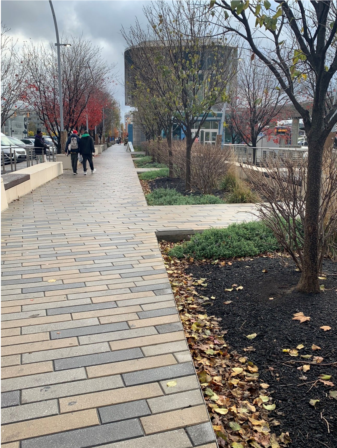
Close view of existing infrastructure within the Washington Street right-of-way
