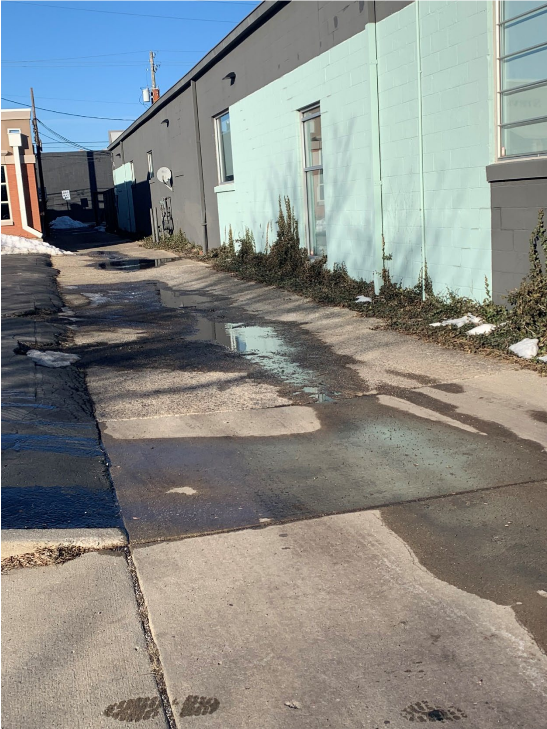
View of the southern portion of the subject alley
