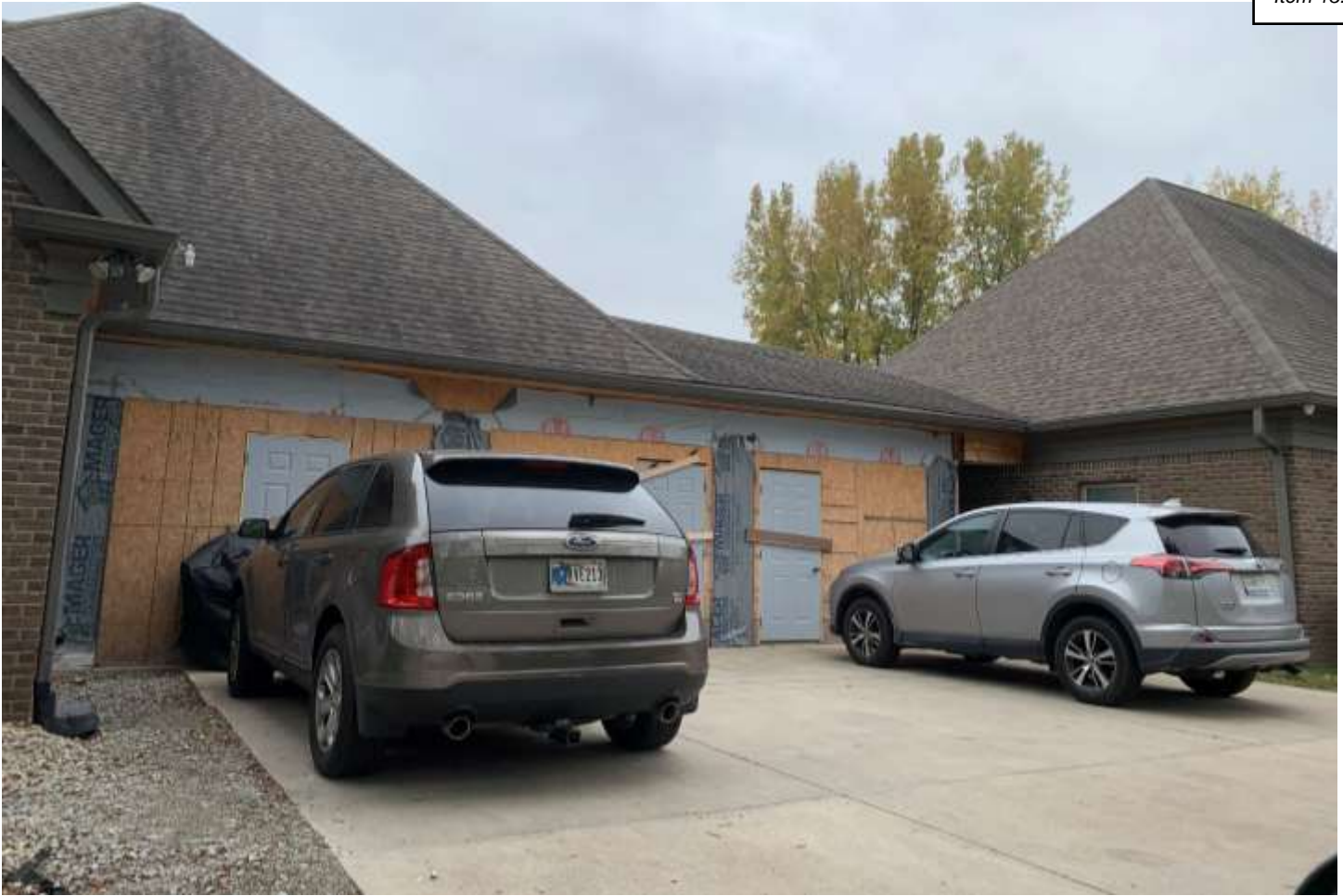
Photo of the northern buiding façade.
