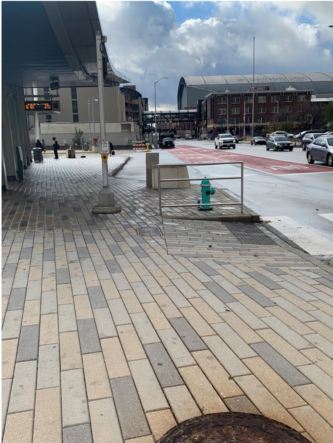
Close view of existing infrastructure within the Delaware Street right-of-way
