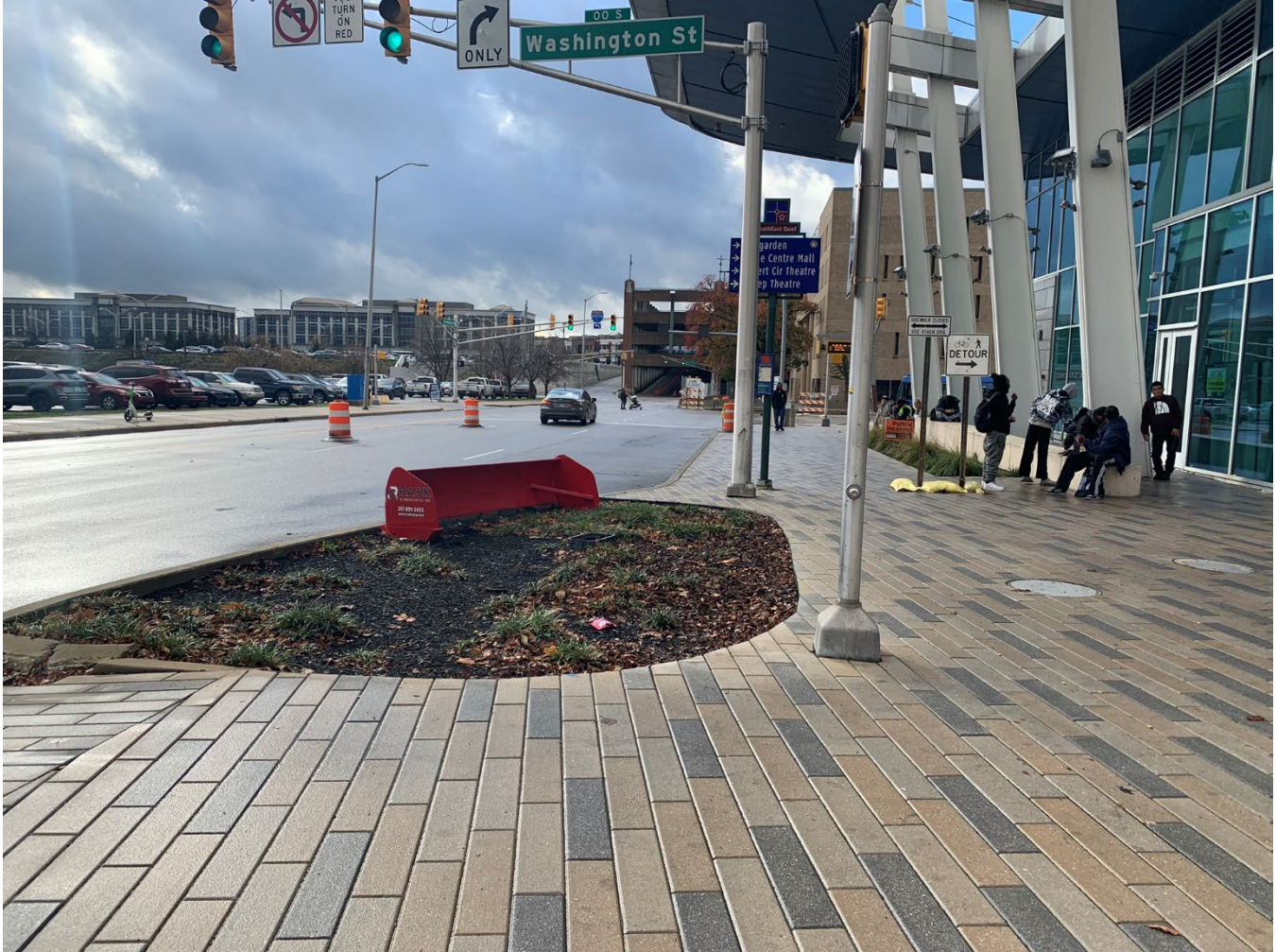
View of existing infrastructure within the Alabama Street right-of-way, from the Washington Street intersection, looking south
