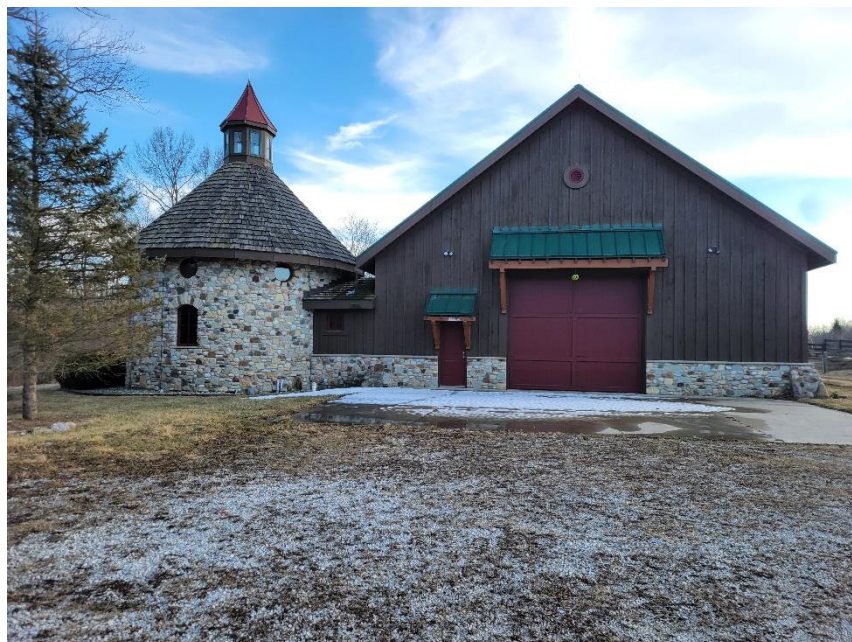
Photo 4: Subject Building Viewed from North
