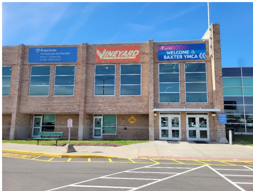
Photo 2: Primary YMCA Entry Viewed from East
