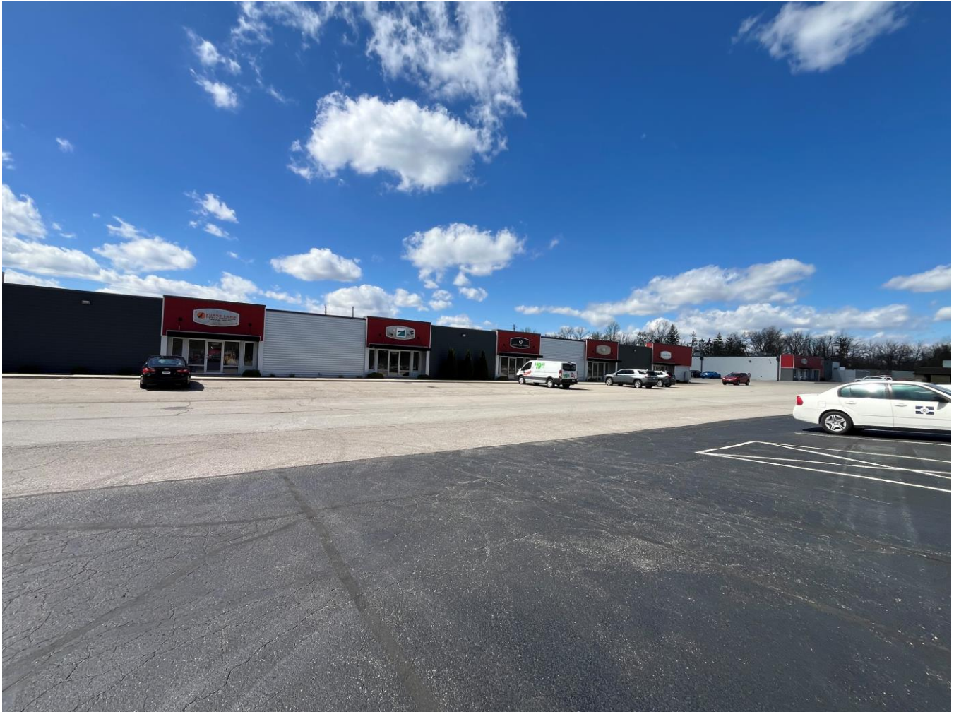
Photo 5: Looking west at neighboring tenant spaces in industrial park
