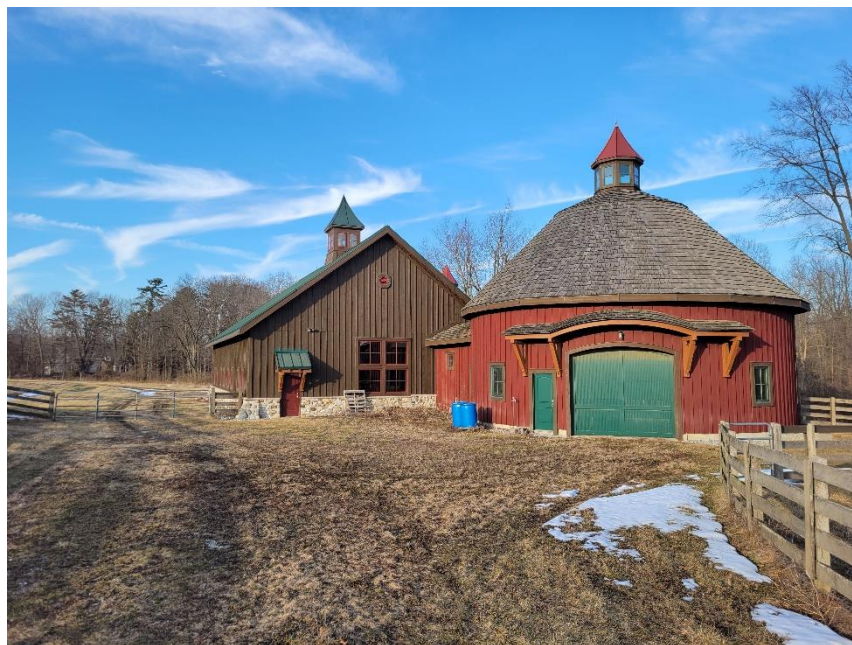
Photo 2: Subject Building Viewed from South
