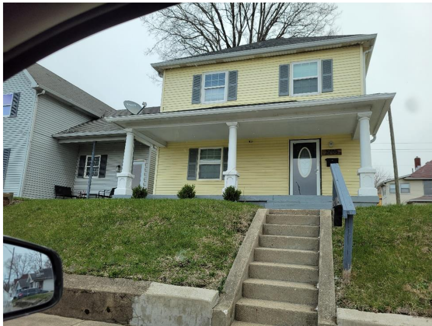
Photo 1: Subject Site Viewed from West
