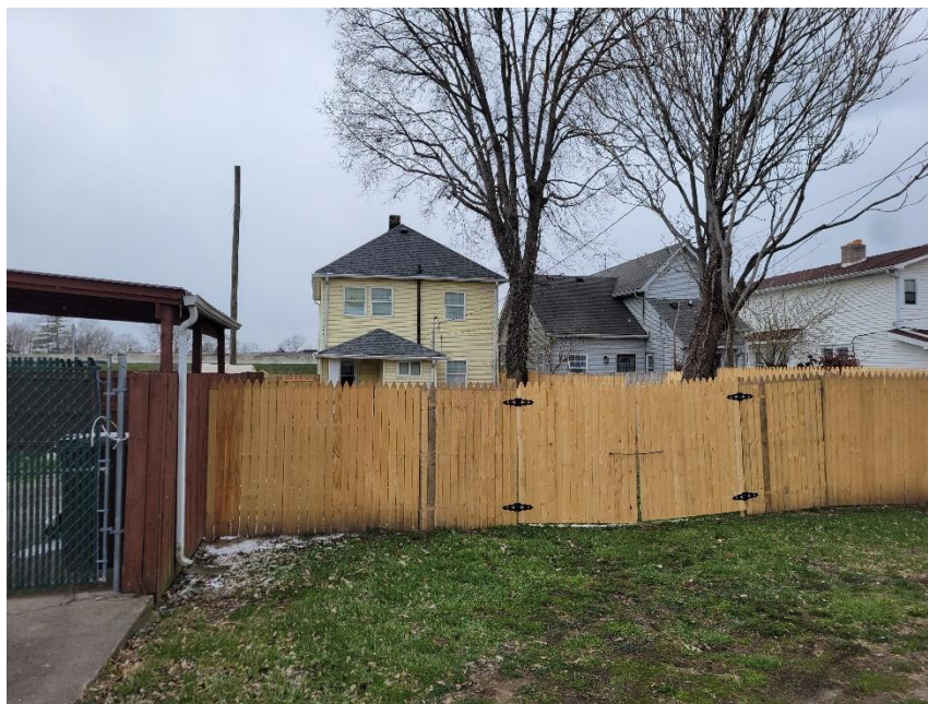
Photo 4: Subject Site Viewed from East
