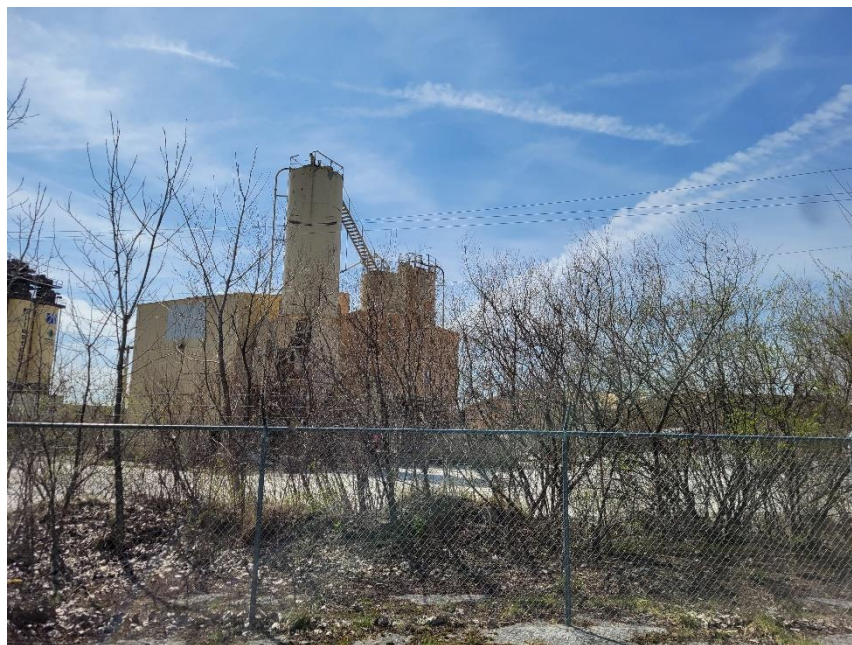
Photo 2: Subject Building Viewed from Northeast
