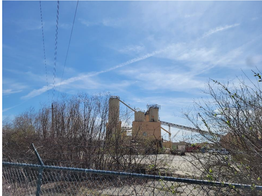
Photo 3: Subject Building Viewed from North
