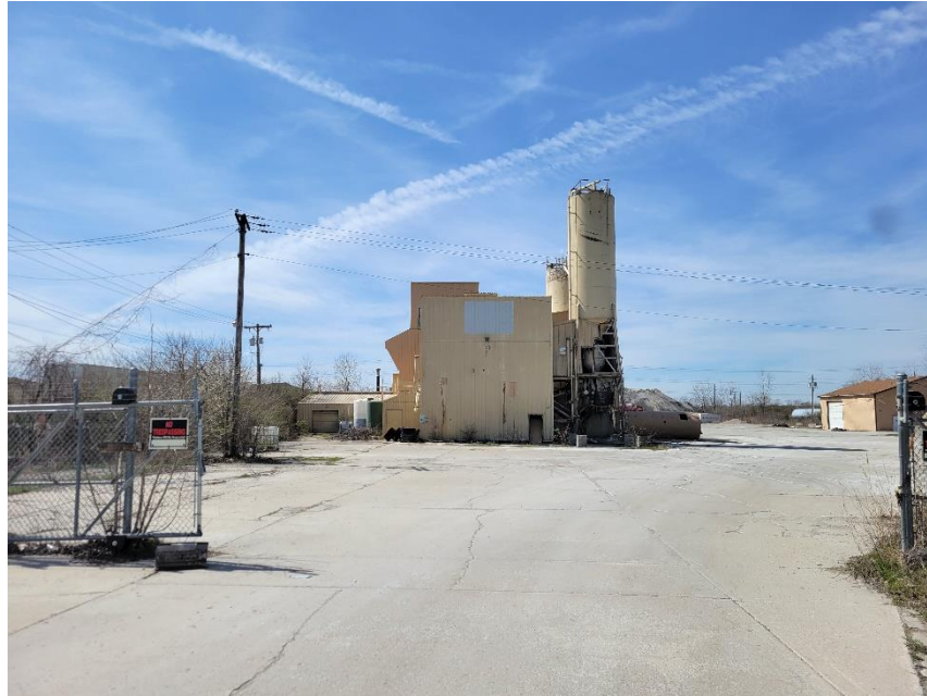
Photo 1: Subject Building Viewed from East
