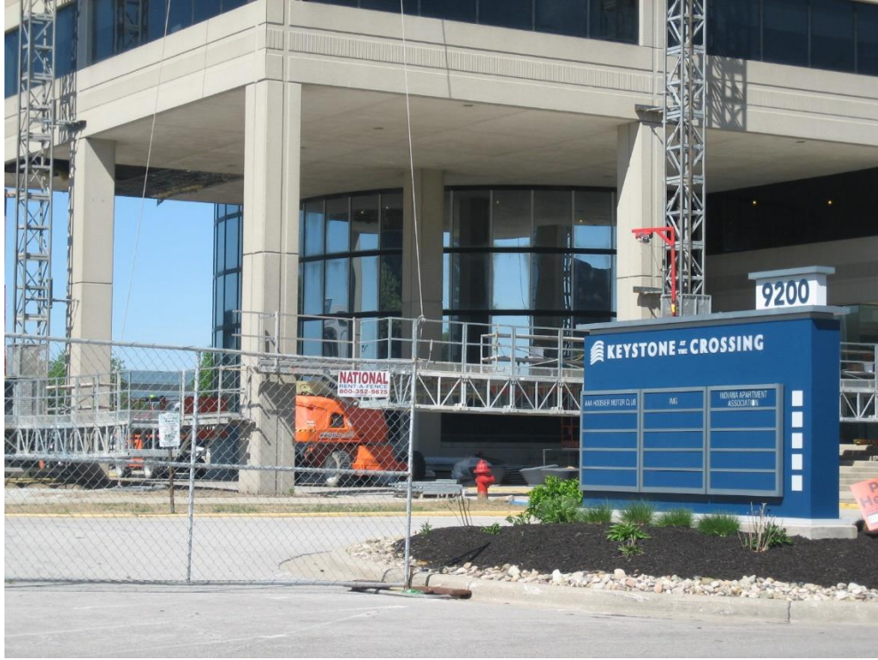
Freestanding monument sign for 9200 Keystone Crossing tenants, easily visible at vehicular / eye level for arriving motorists from the south, looking north.
