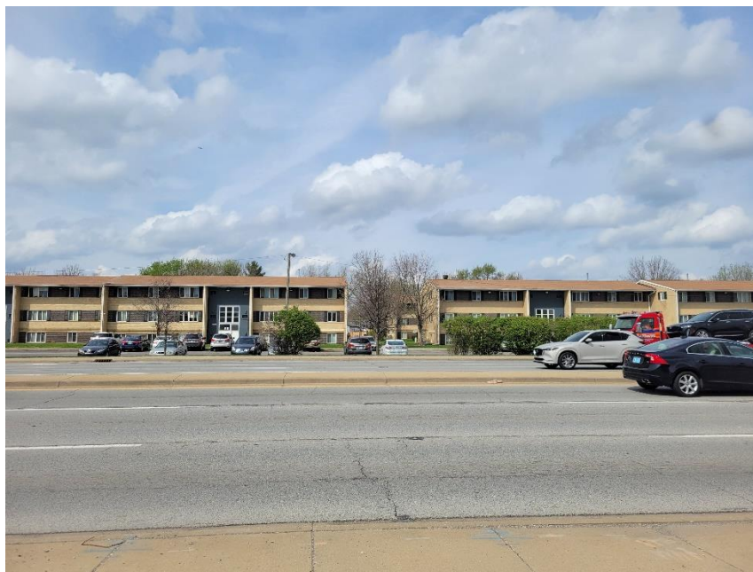
Photo 4: Adjacent Property to North
