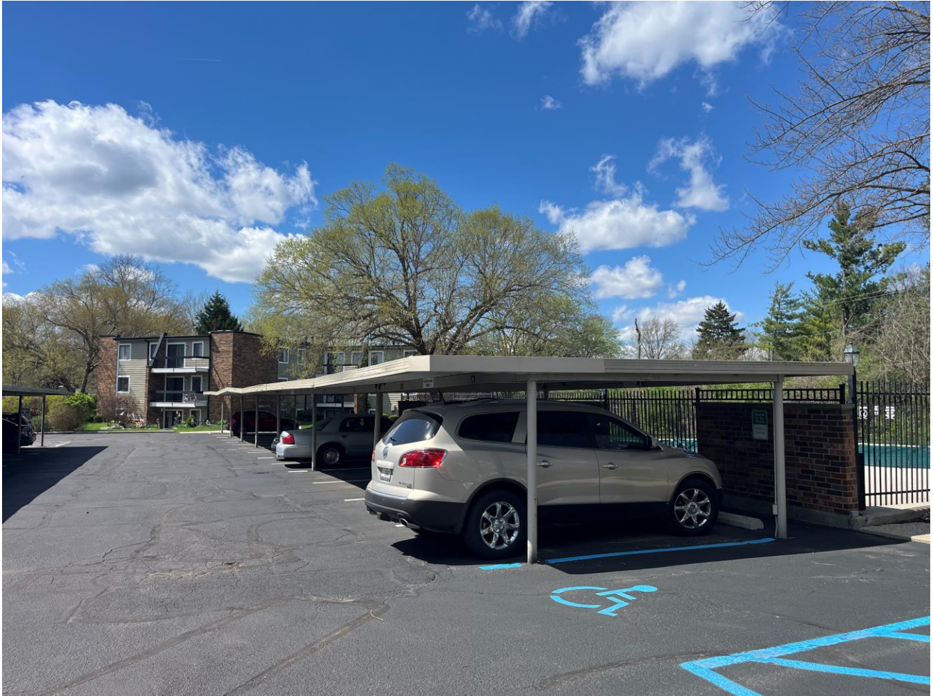
Photo 2: View of apartment parking area with pool in background
