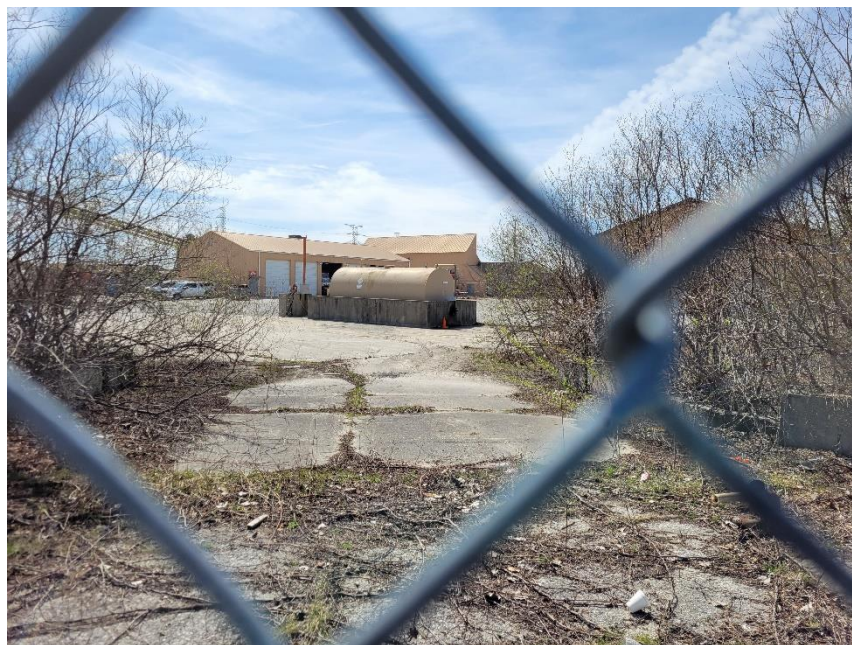
Photo 4: Subject Site Viewed from North
