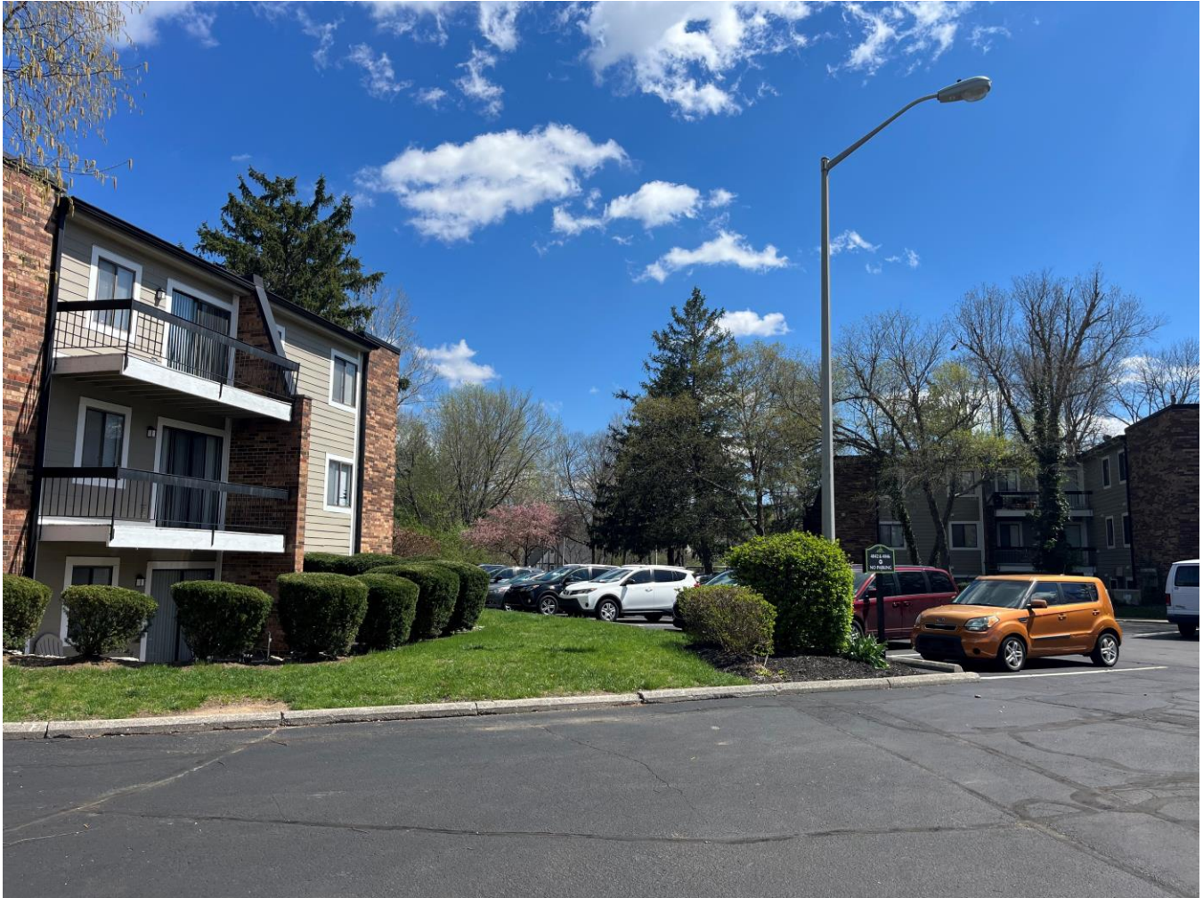
Photo 1: View of apartment complex
