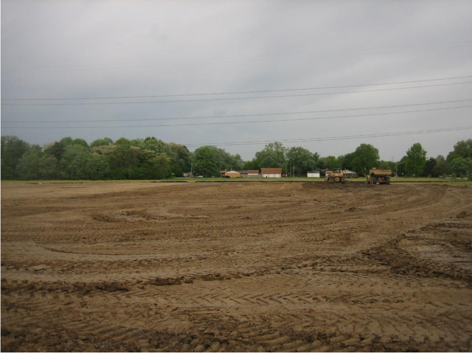
Subject site, looking north from Highcrest Road.
