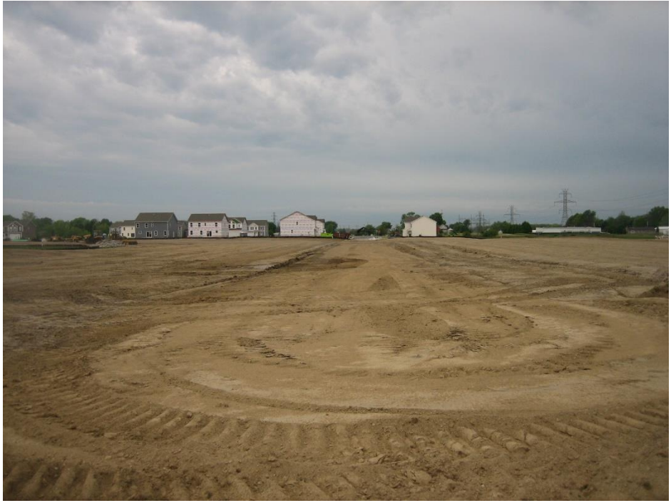
Subject site, looking west from Asher Way.
