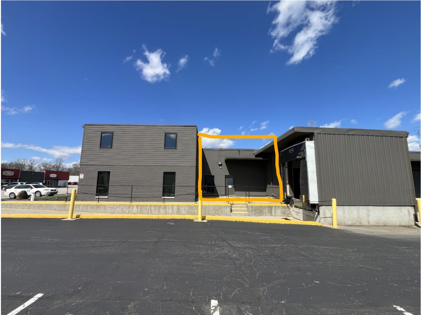
Photo 2: South side of the building; deck will not encroach on ramp space
