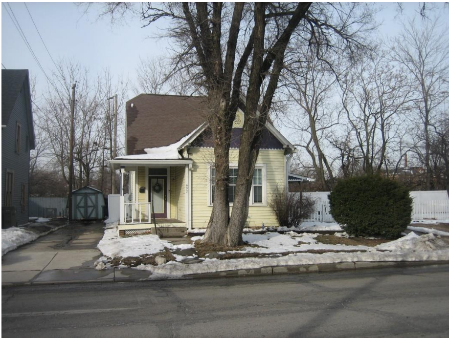
Adjacent dwelling to the west, looking north.
