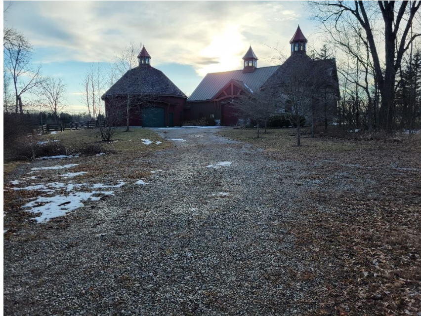
Photo 1: Subject Building Viewed from East
