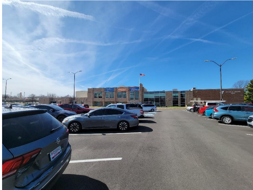
Photo 1: Subject Site Viewed from East
