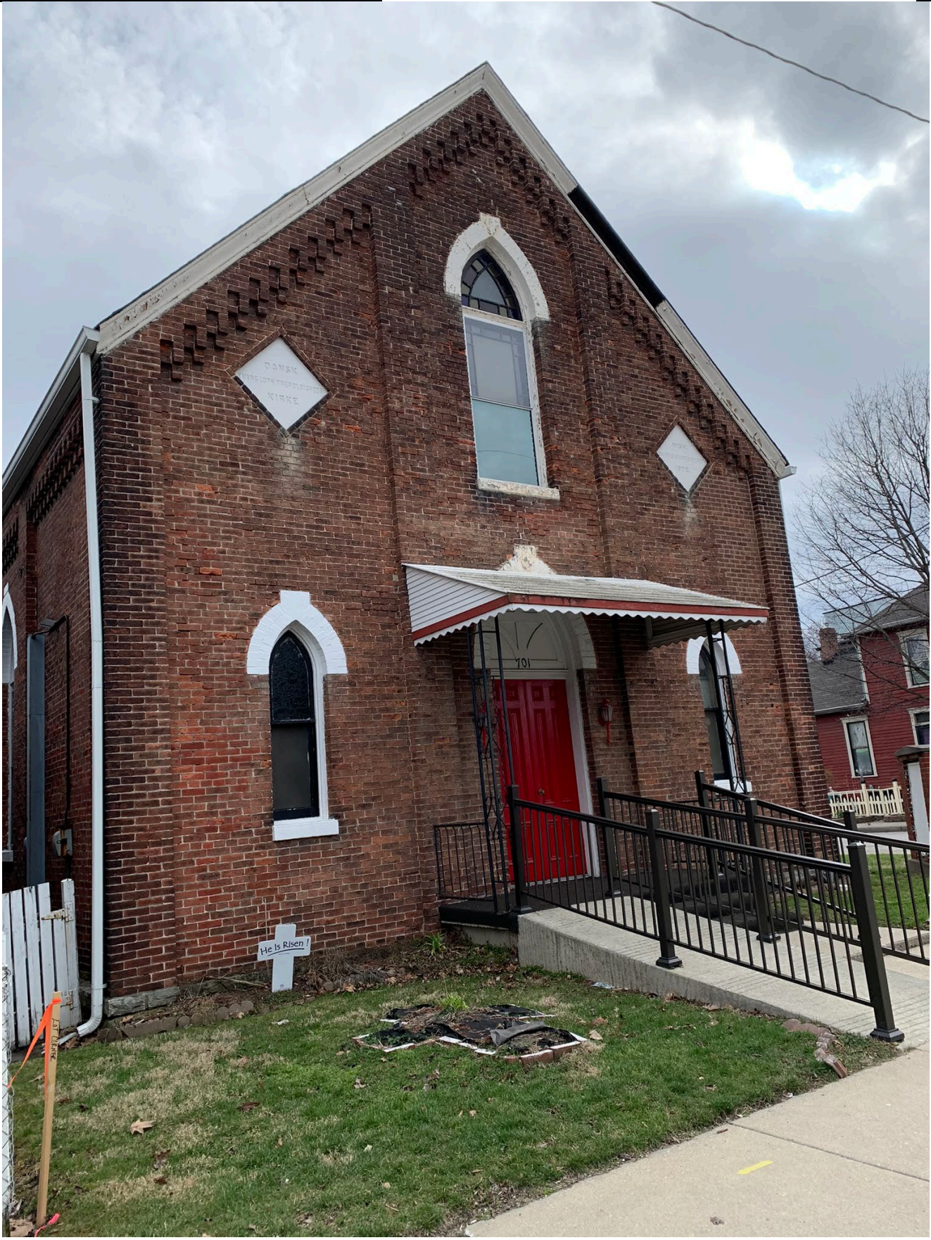
View of the front of the building along McCarty Street
