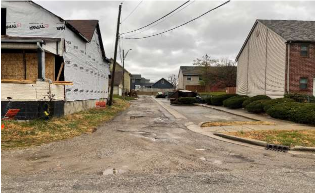
Photo Three: Looking East Along Marlowe Avenue.
