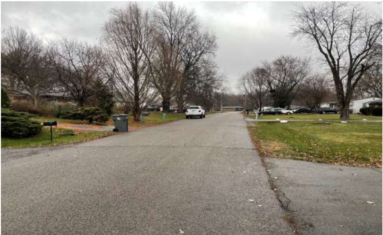
Photo Two: Looking South Along Kristen West Drive.
