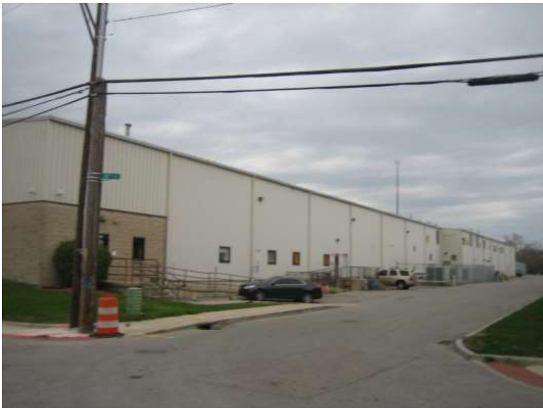
Adjacent government residential work release facility to the northeast
