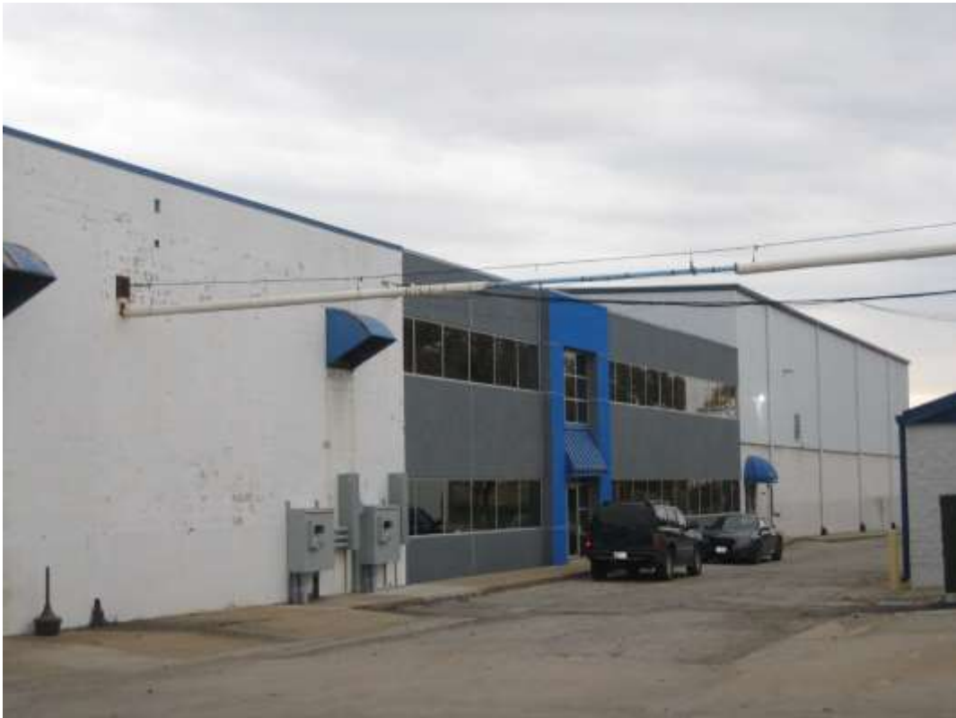
Adjacent manufacturing facility to the southeast.
