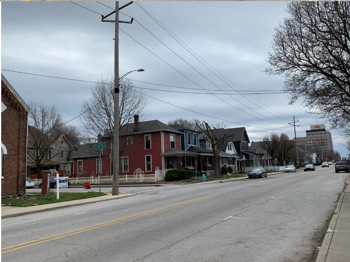
Views of the abutting dwelling to the east and subject building (top); and dwellings to the west, along McCarty Street
