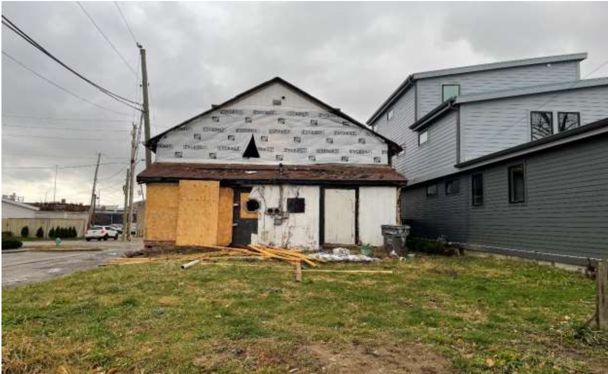
Photo Five: Rear of Subject Site.
