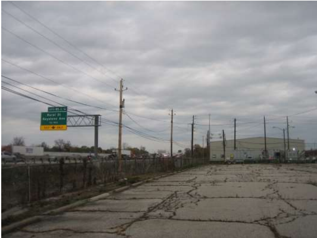
Photo of subject site, looking northeast.
