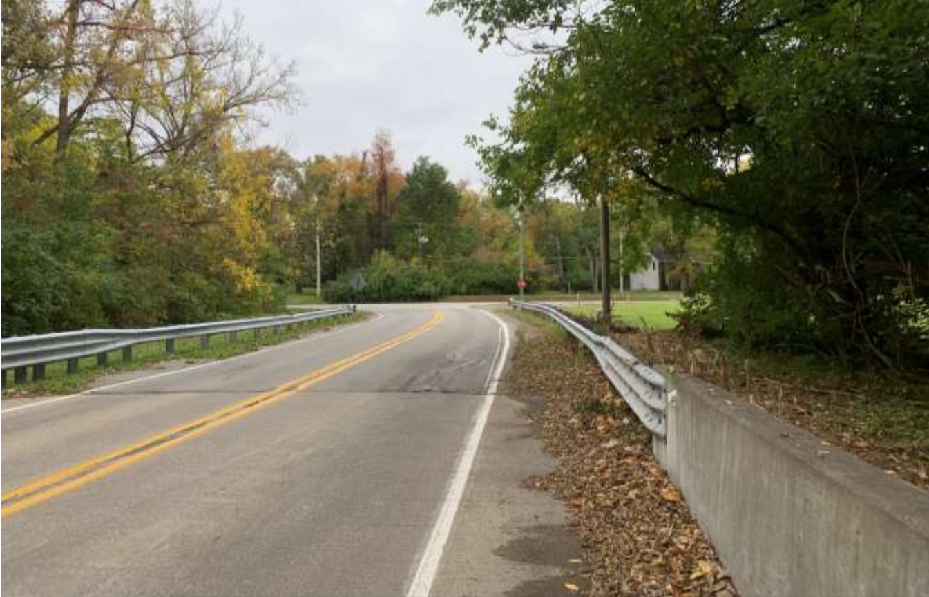
Photo of the eastern street frontage looking south on Millersville Road.
