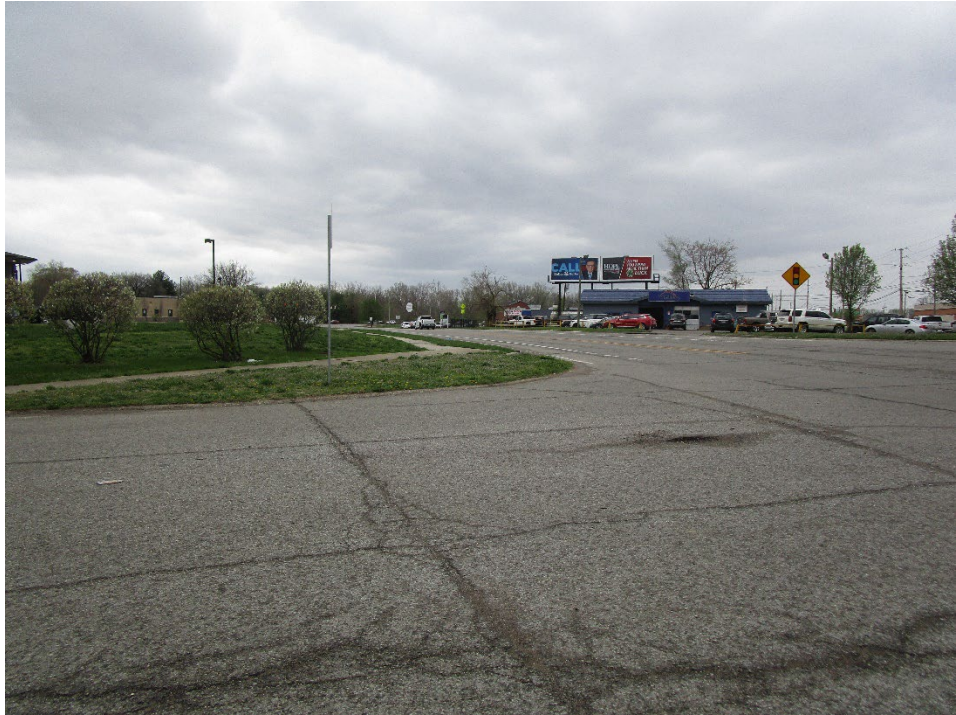
View looking south along Allisonville Road
