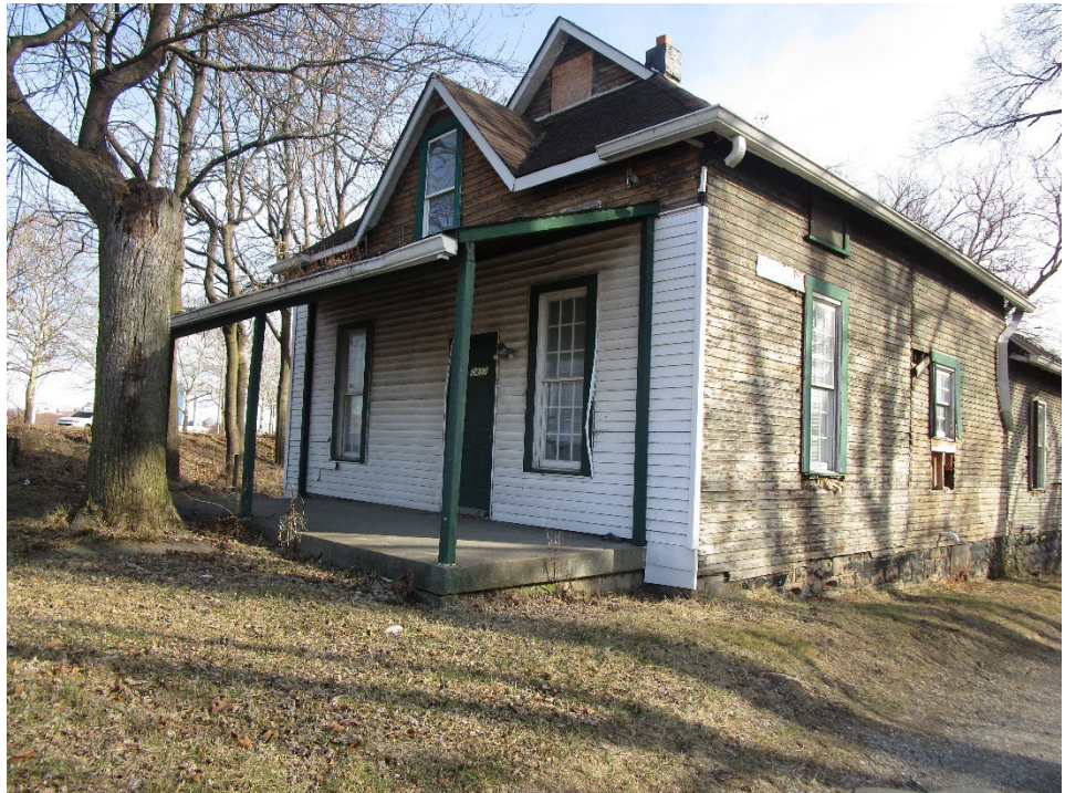
View of site looking southeast at last dwelling on Saulcy Street
