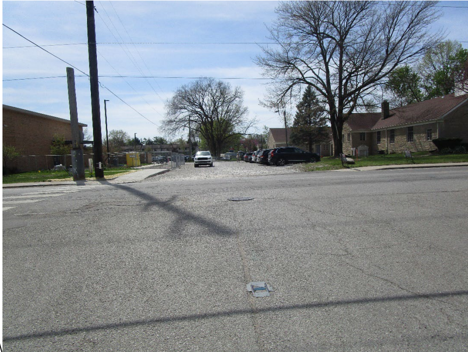
View looking south across intersection of East 54 th Street and Haverford Avenue
