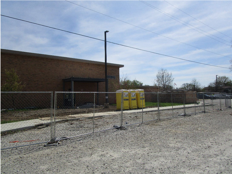
View of site looking southeast across Haverford Avenue
