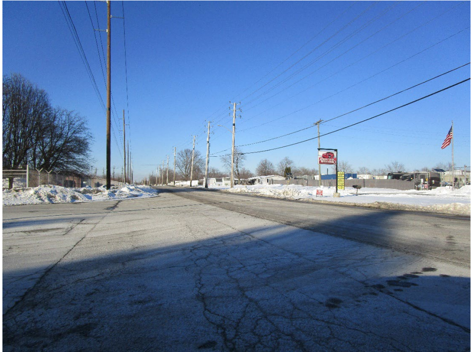
View looking north along South Shortridge Road
