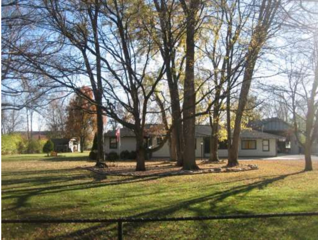
The residence, looking south, from 69 th Street.
