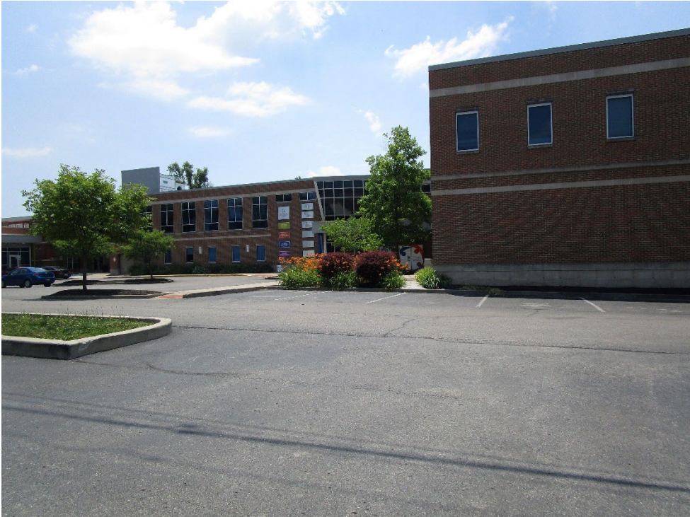
View from site looking southeast
