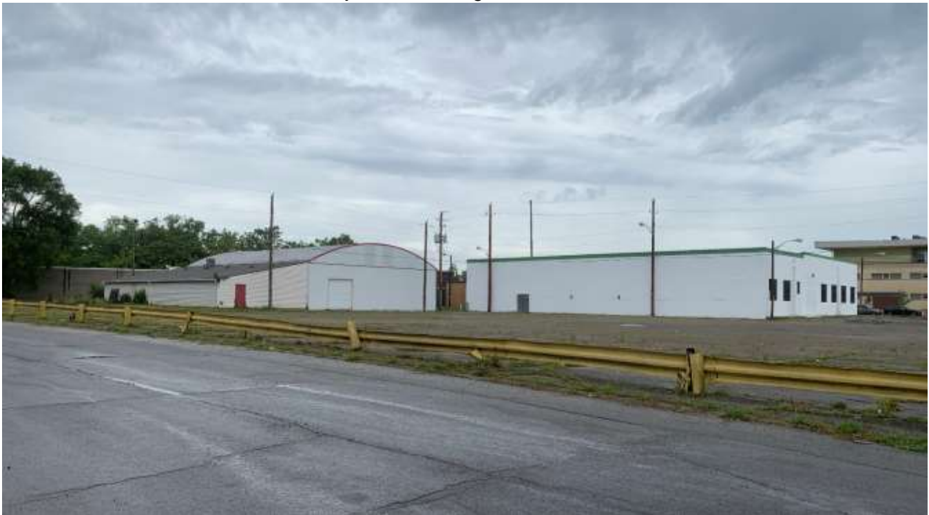
Photo of the southern property boundary looking north.
