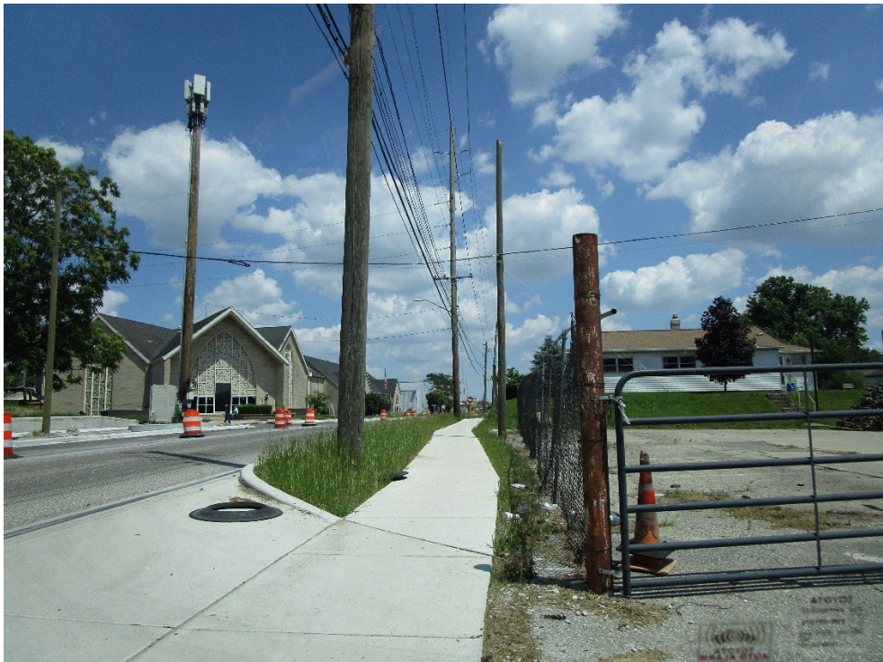
View looking east along West Morris Street
