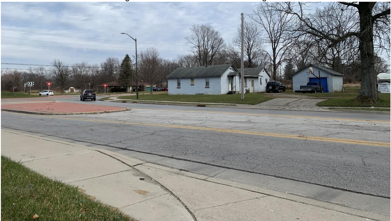
Photo looking east across German Church Road to the corner subject site. Buildings to be removed .
