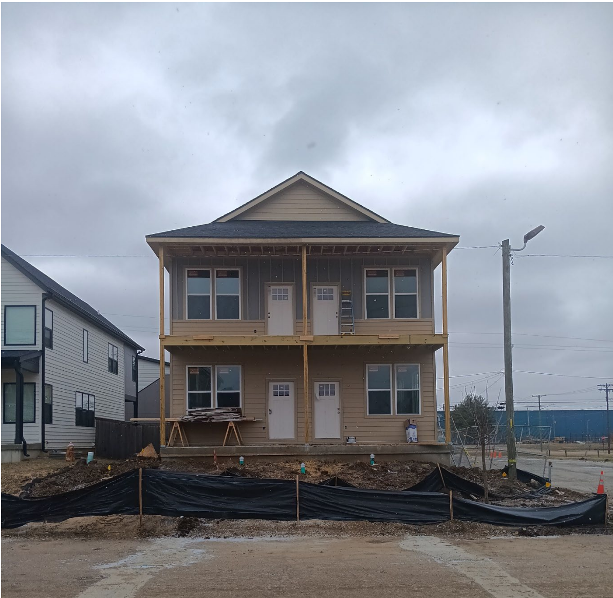
Exhibit 4: Duplex constructed on 2013 Yandes Street.
