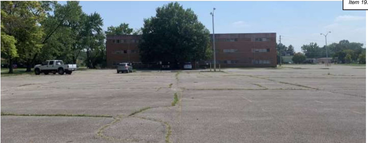
Photo of the remaining church parking lot and building.
