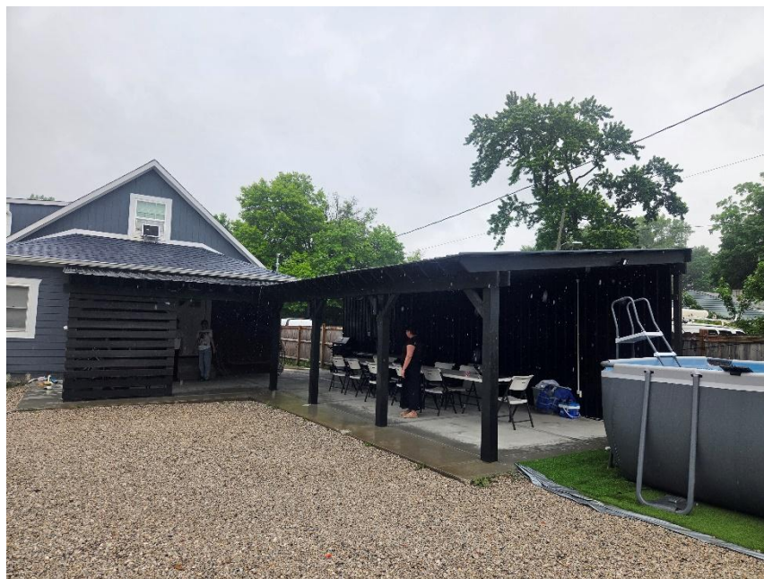
Photo 4: Subject Shelter Viewed from Southwest (Internal to Lot)
