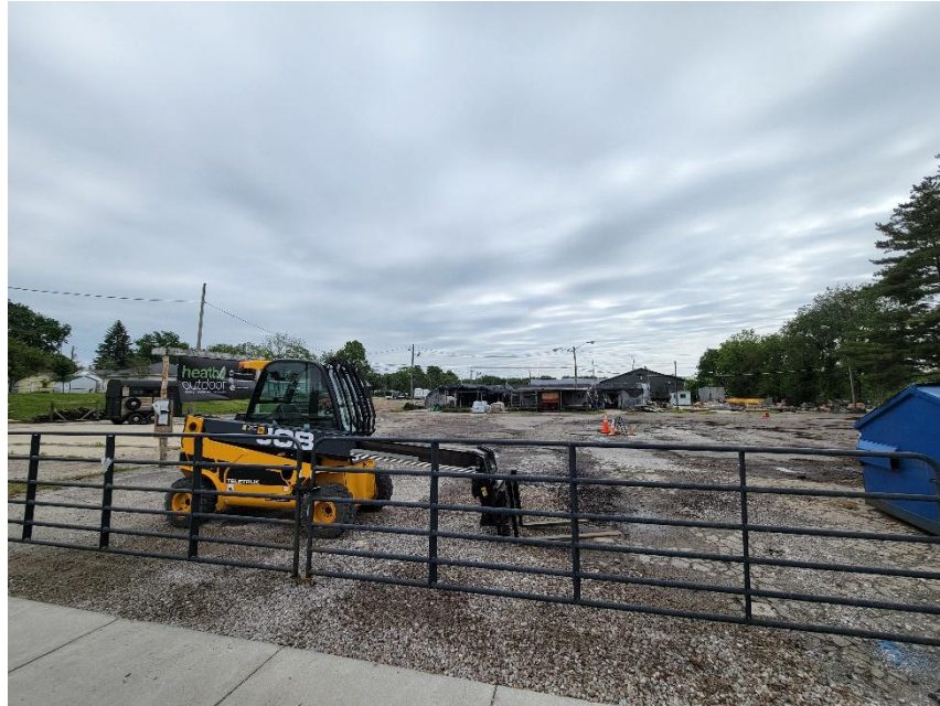
Photo 9: Contractor Use (2401 Morris) Viewed from North
