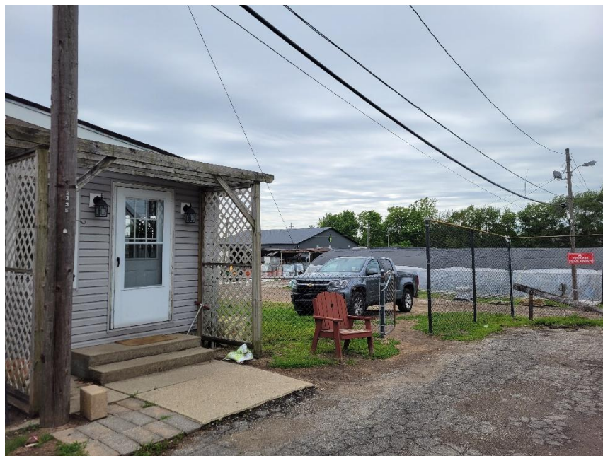
Photo 10: Contractor Use (2401 Morris) Viewed from Northeast (Alley)
