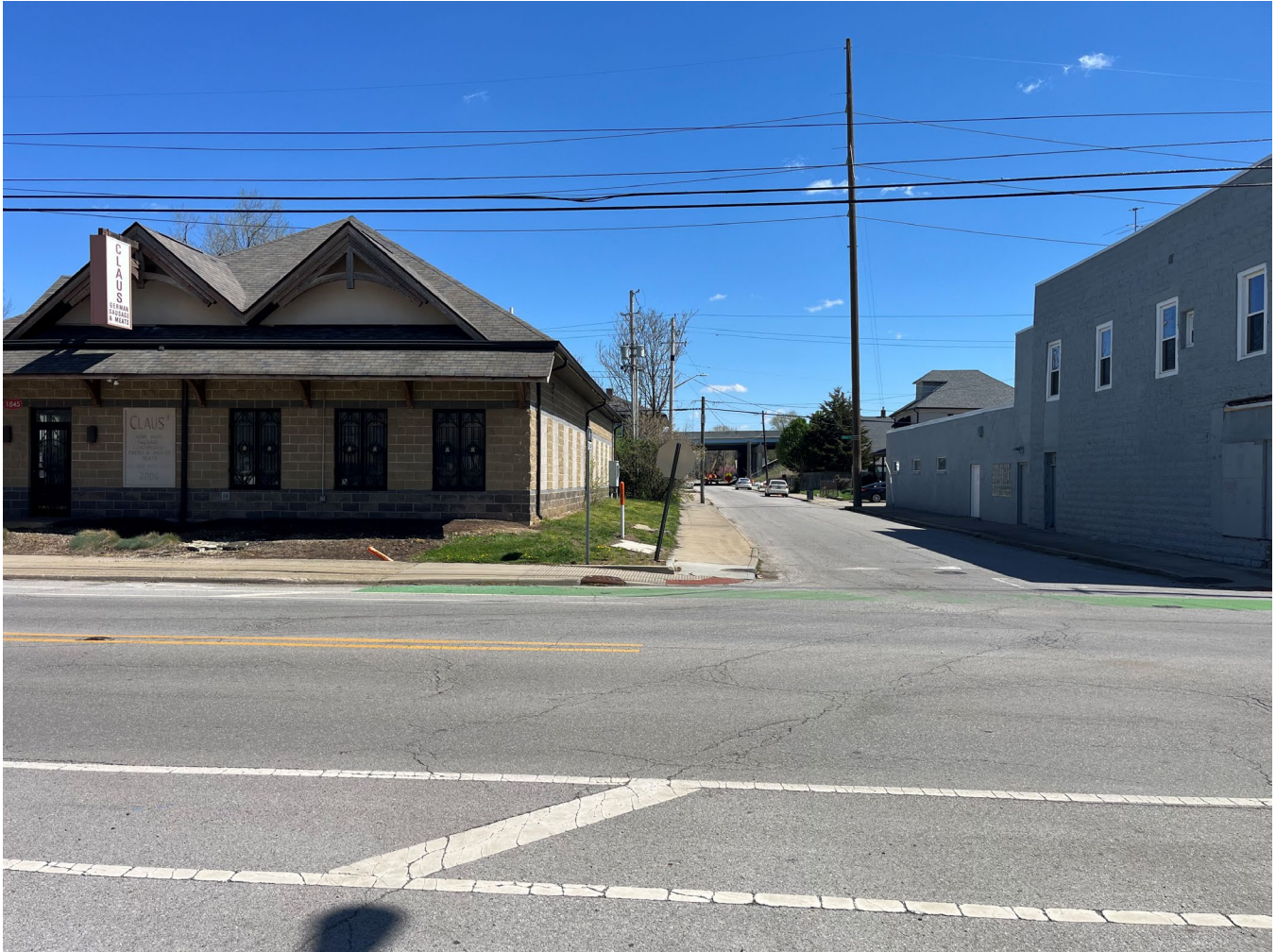
Photo 3: Looking across the street from subject site at butcher shop and Naomi Street
