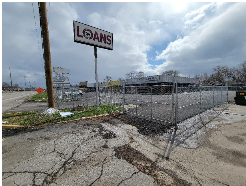
Photo 2: Subject Fence Viewed from Northwest
