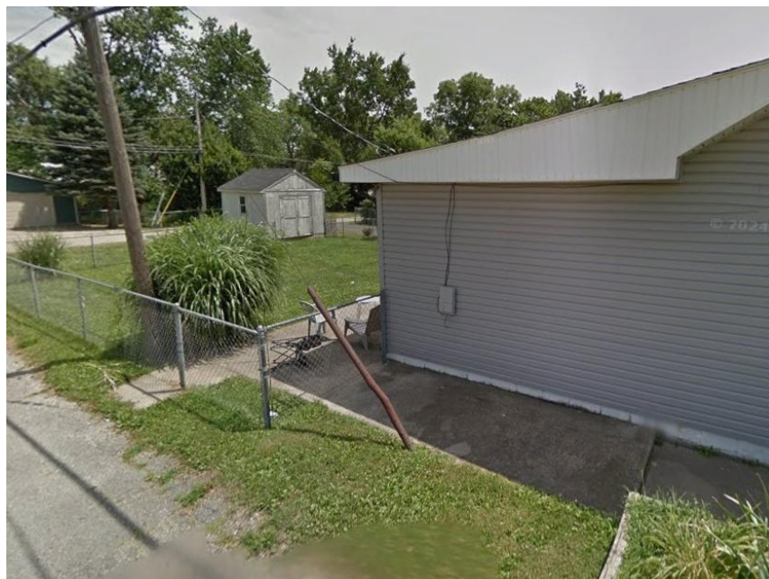
Photo 4: 1211 Tremont Viewed from North (July 2011)
