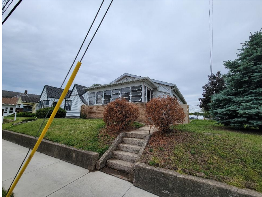
Photo 1: 2335 Morris Viewed from North
