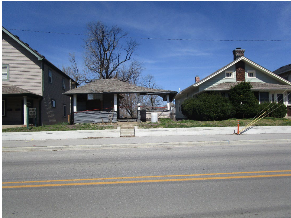
View of site looking north across West Morris Street
