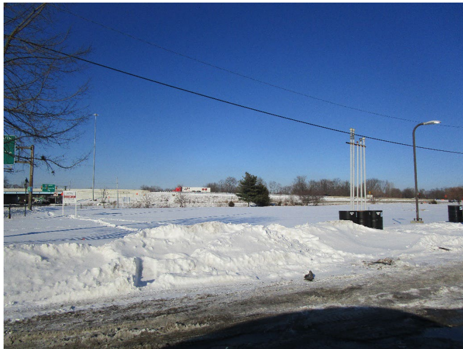
View of site looking northeast
