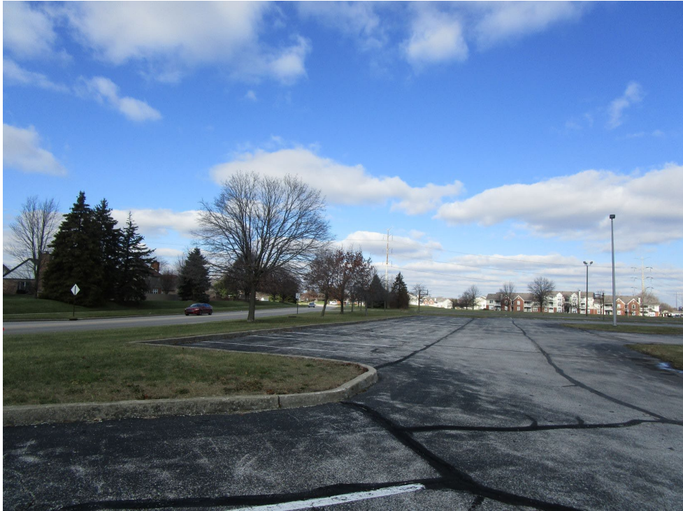
View of site looking north
