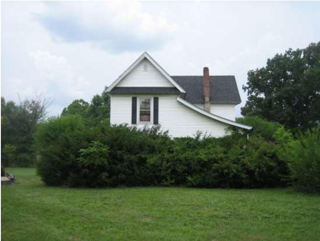
Photo of the subject site, primary dwelling on parcel 1, looking west
