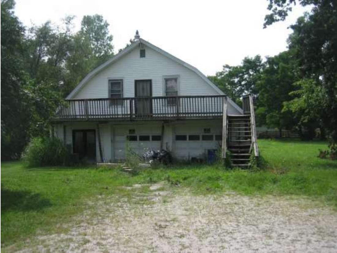
Photo of the subject site, second primary dwelling on parcel 1, looking west
