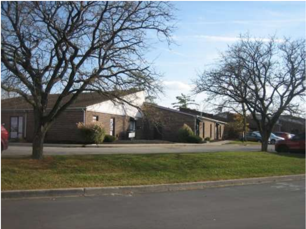
View of adjacent integrated commercial center offices to the southeast.
