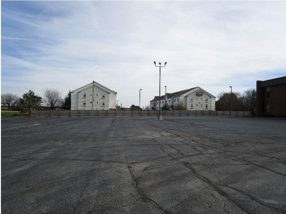
View of site looking east from adjacent property to the west
