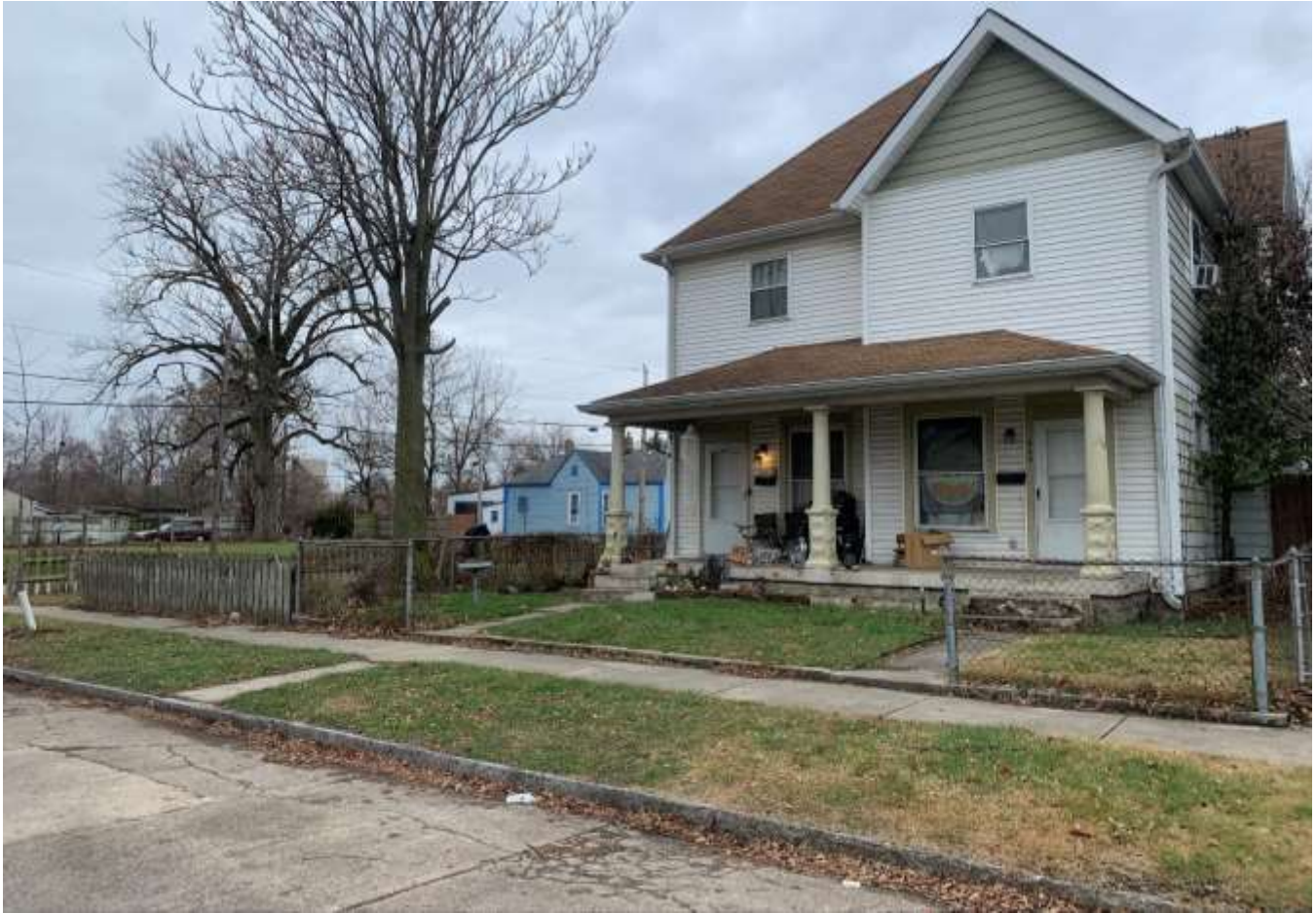
Photo of a two-family dwelling west of the site.
