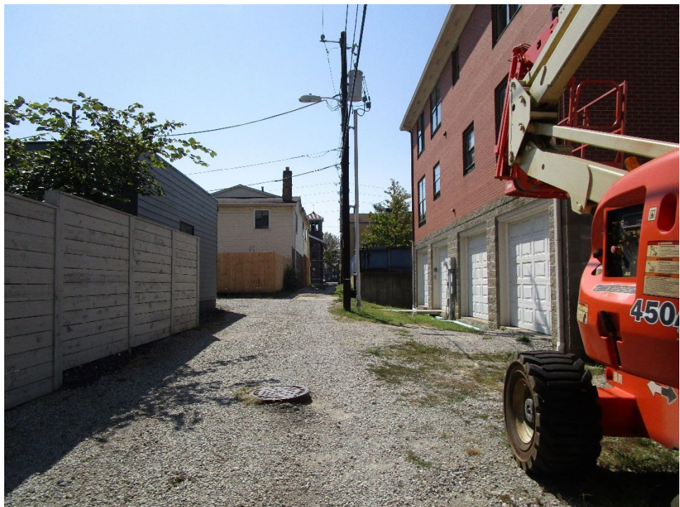
View looking south along north / south alley
