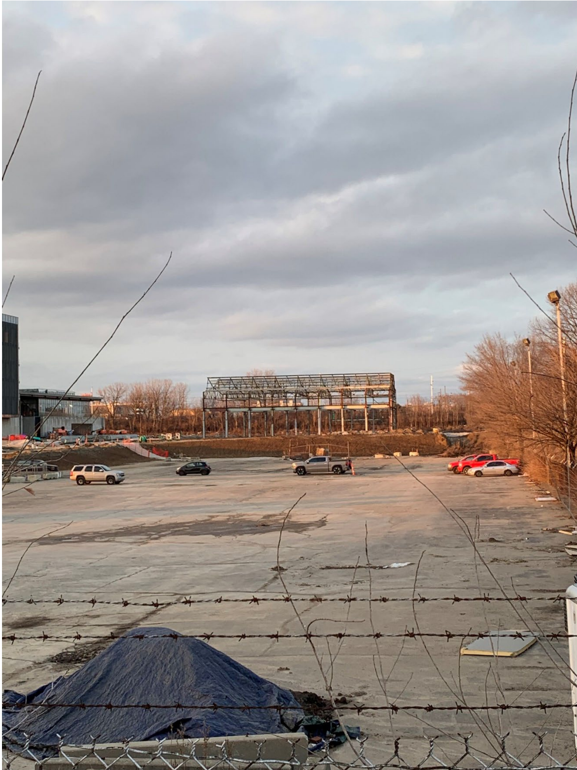
Photo of remaining section of former GM Stamping Plant structure
