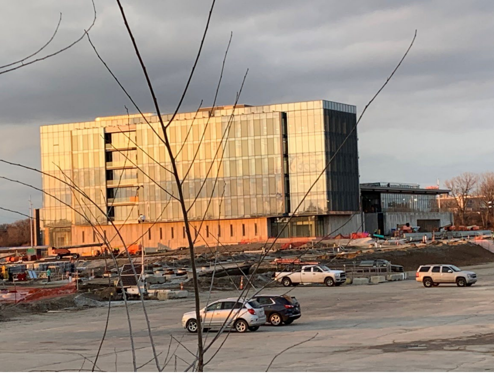
Photos of Elanco campus buildings, under construction
