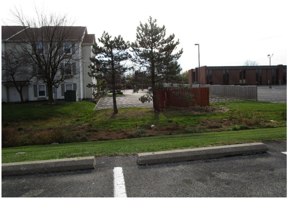
View of site looking south from adjacent property to the north
