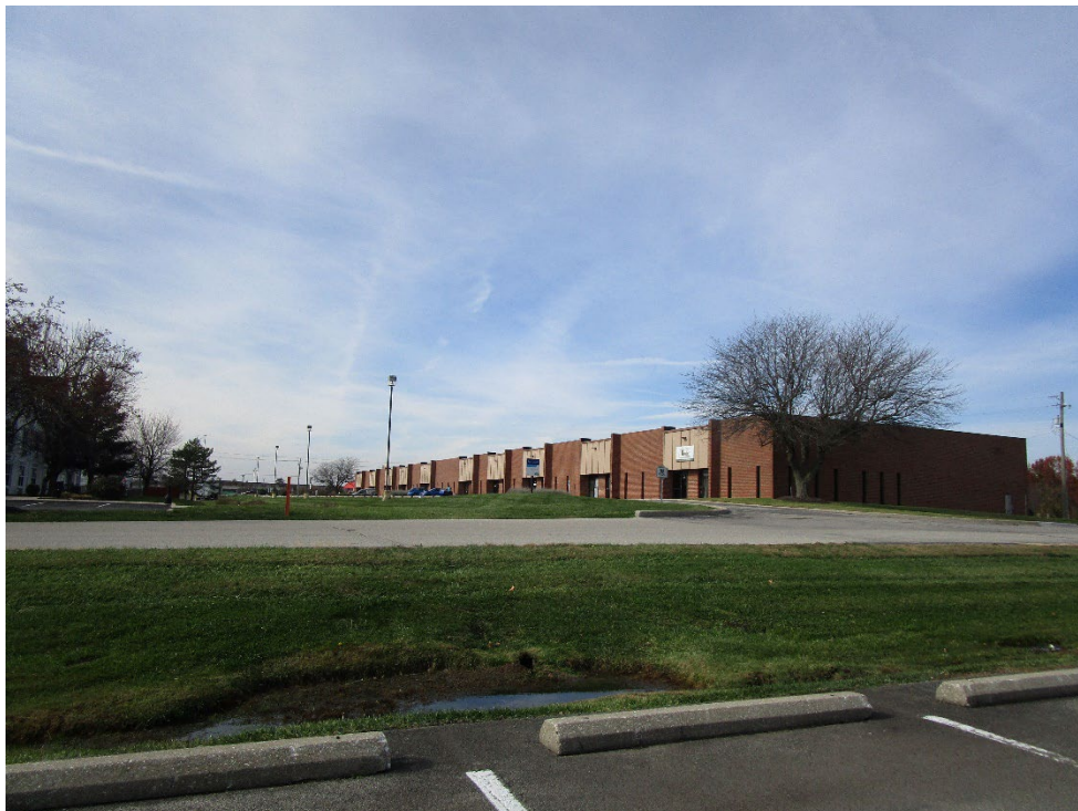
View of adjacent property to the north looking northwest across access drive
