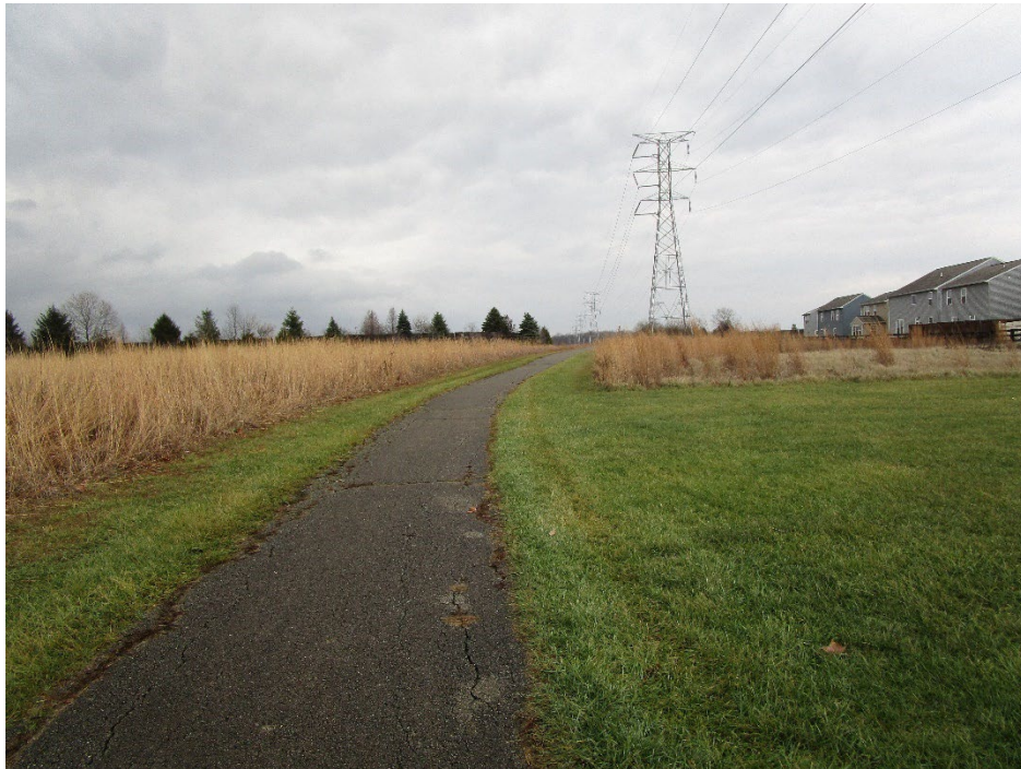
View of site looking east
