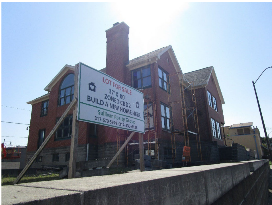
View looking southeast at adjacent two-family dwelling
