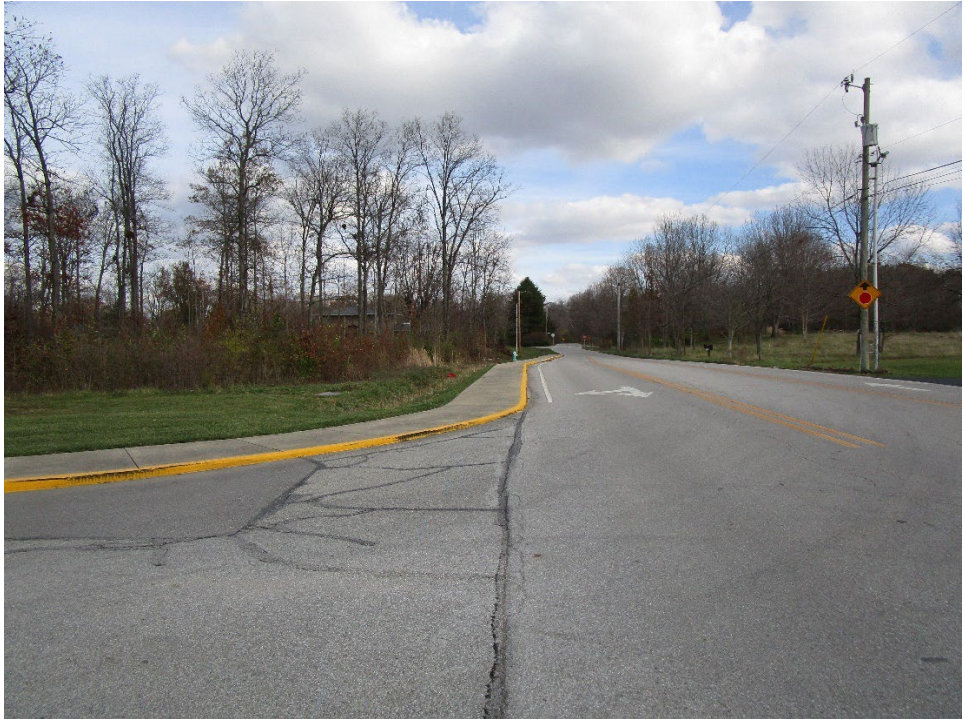
View looking east along Indian Creek Road South
