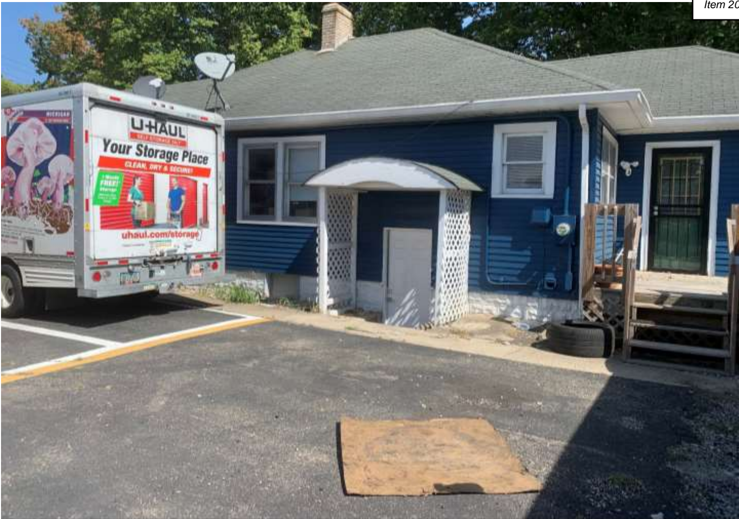
Photo of the western office façade.
