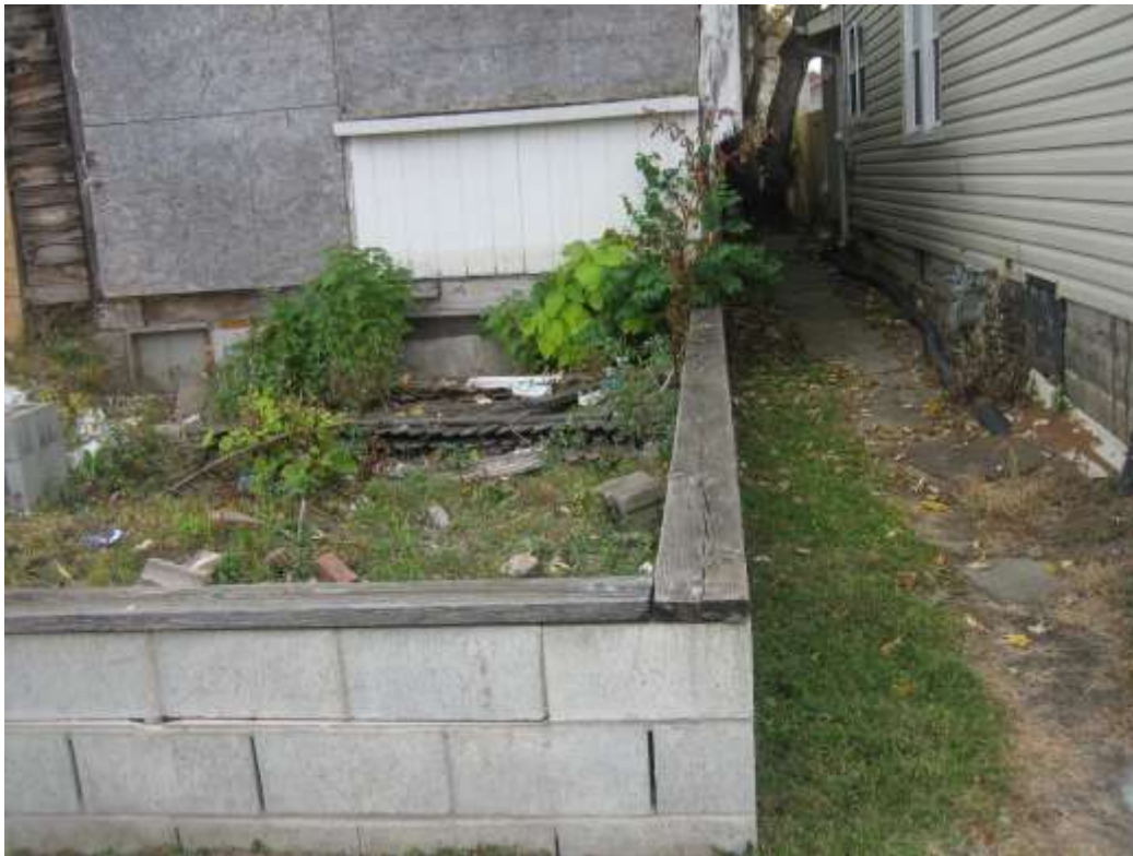
Photo of the existing foundation to be built upon, with the cinder block portion being moved to a two-foot south side setback.
