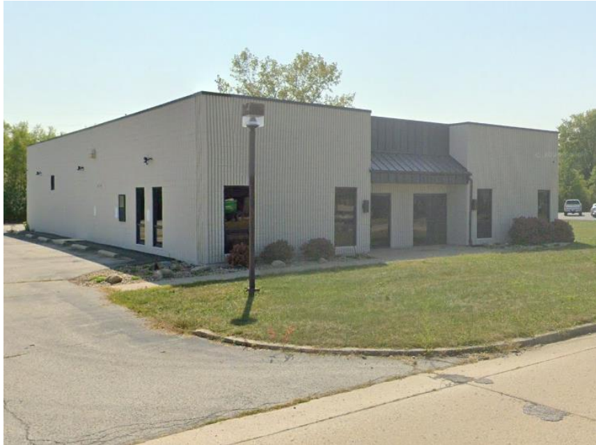
Photo 1: Subject Site Viewed from North (September 2024)
