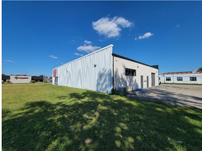
Photo 3: Subject Site Viewed from Southwest
