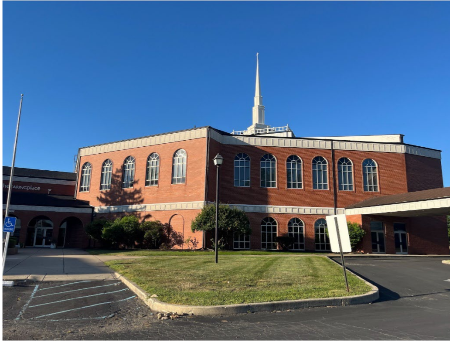
Looking southwest at Church
