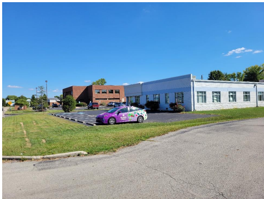
Photo 8: Adjacent Property to East
