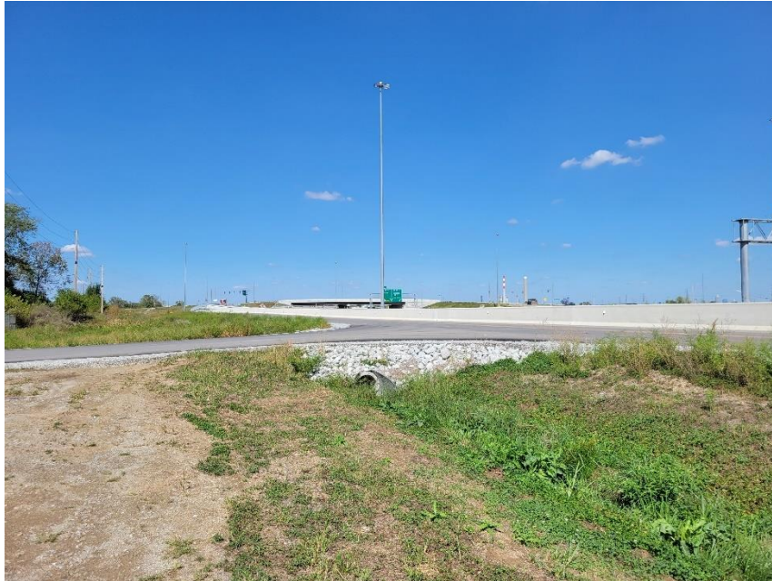
Photo 7: Existing Access Drive to North of Site
