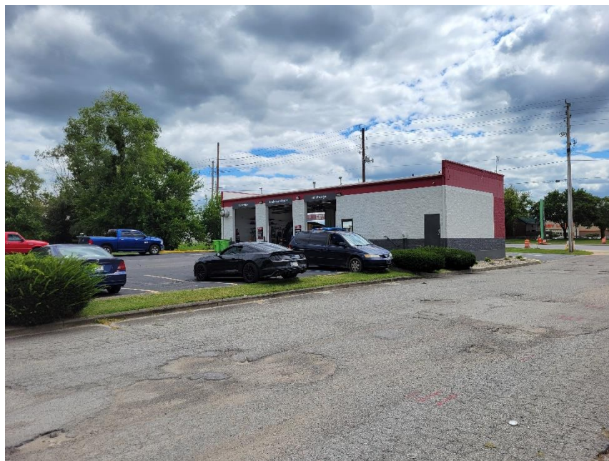
Photo 12: Adjacent Property to East
