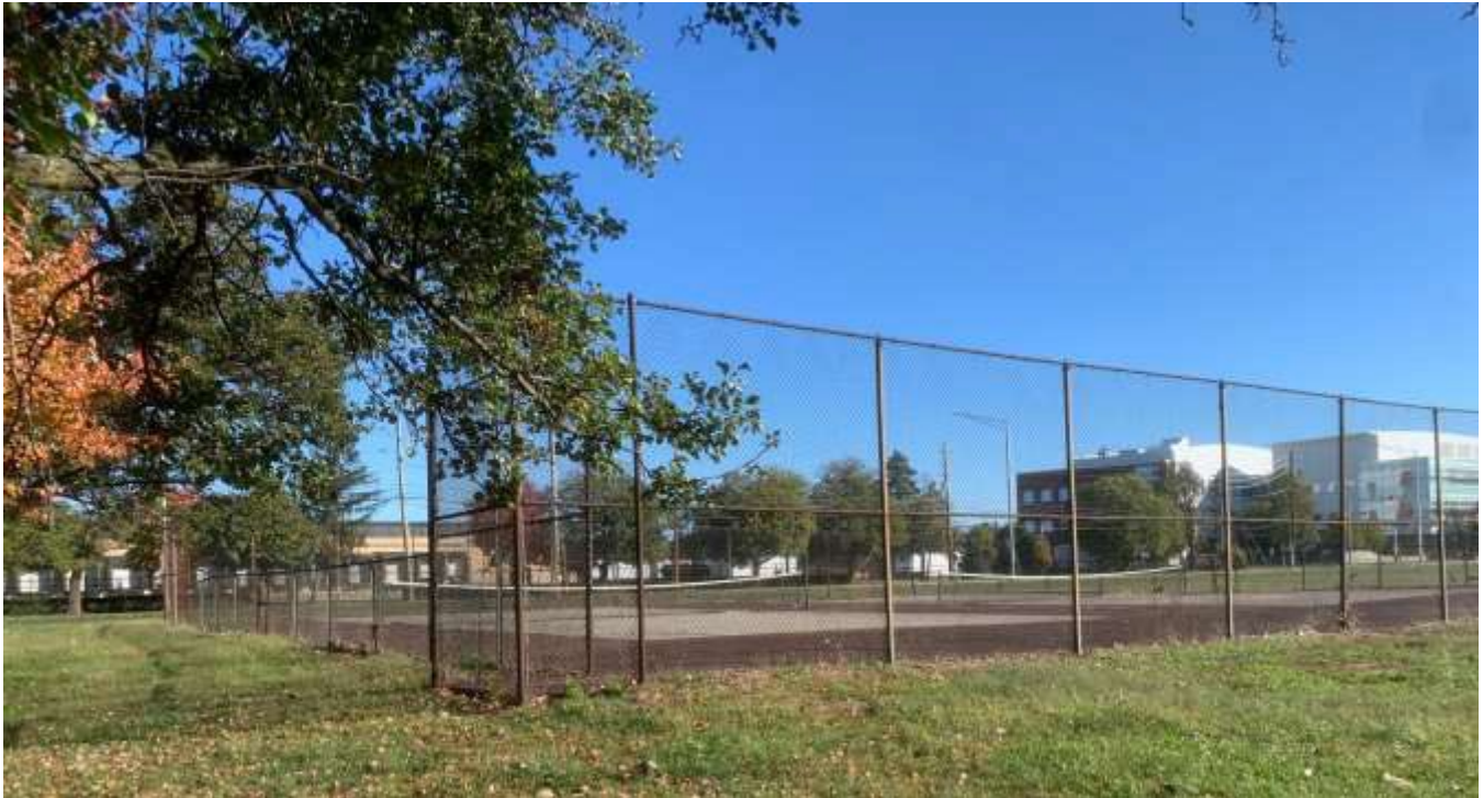
Photo of the existing tennis courts at 700 West 16th Street.
