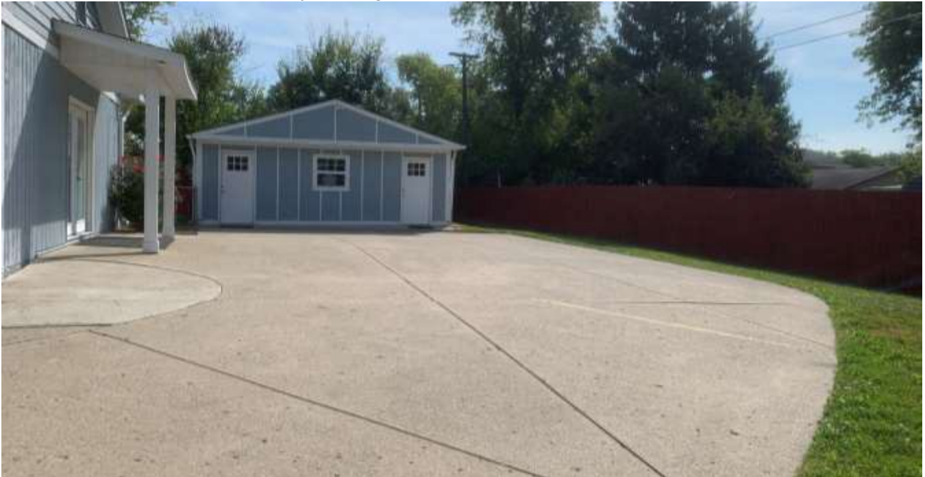
Photo of an accessory building at 2705 North Post Road.
