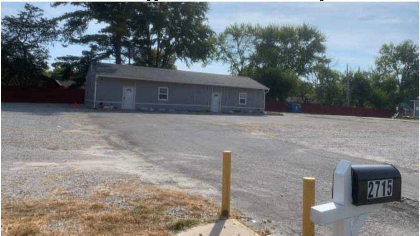
Photo of the existing building on site at 2715 North Post Road.
