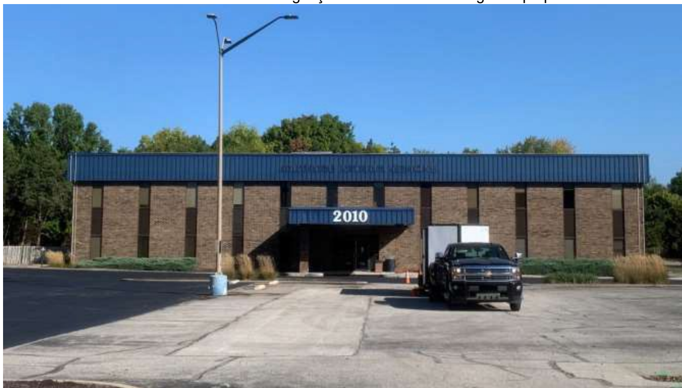
Southern building façade where new wall sign is proposed.
