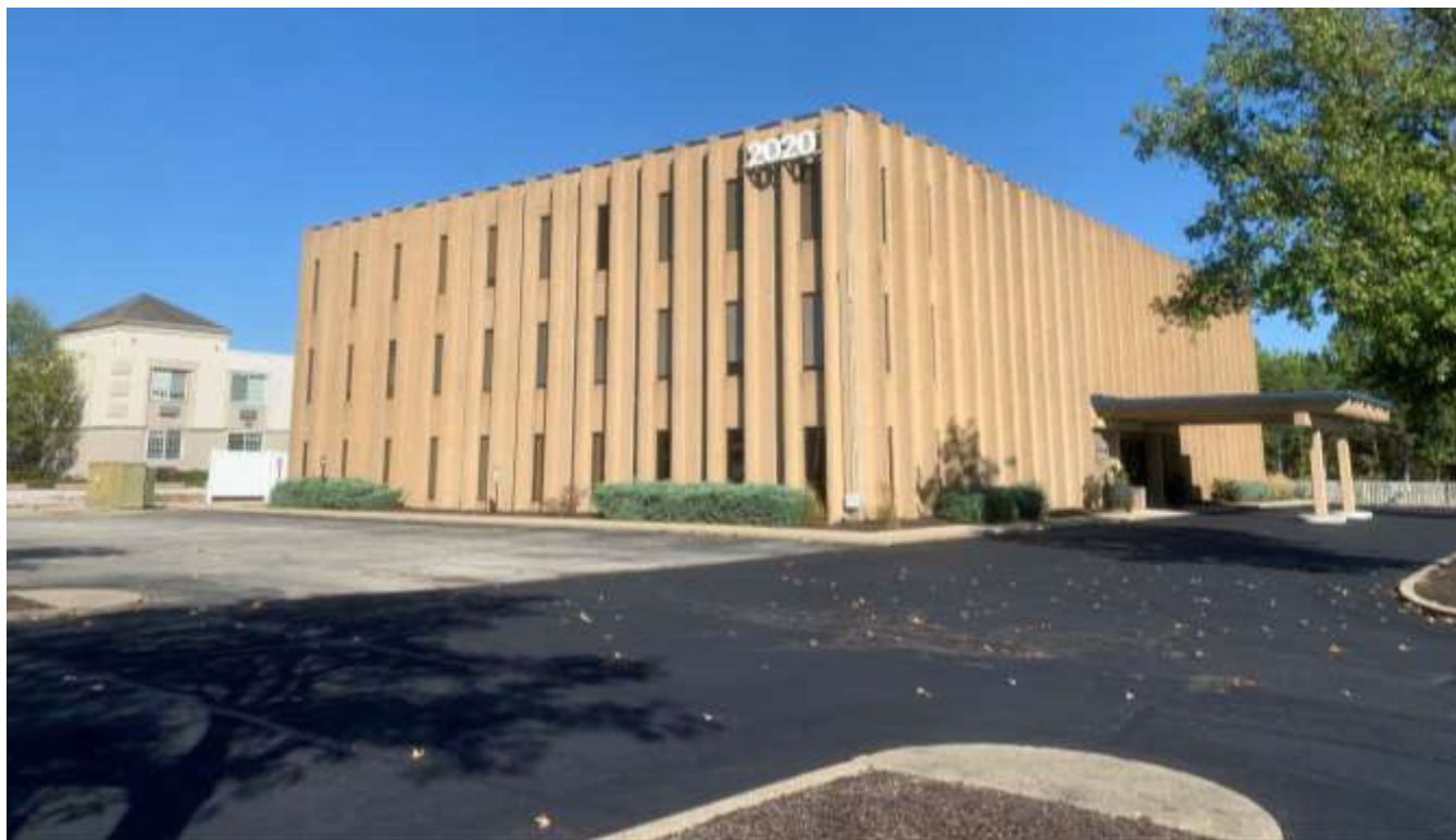
Southern and eastern building façades where new wall sign are proposed.
