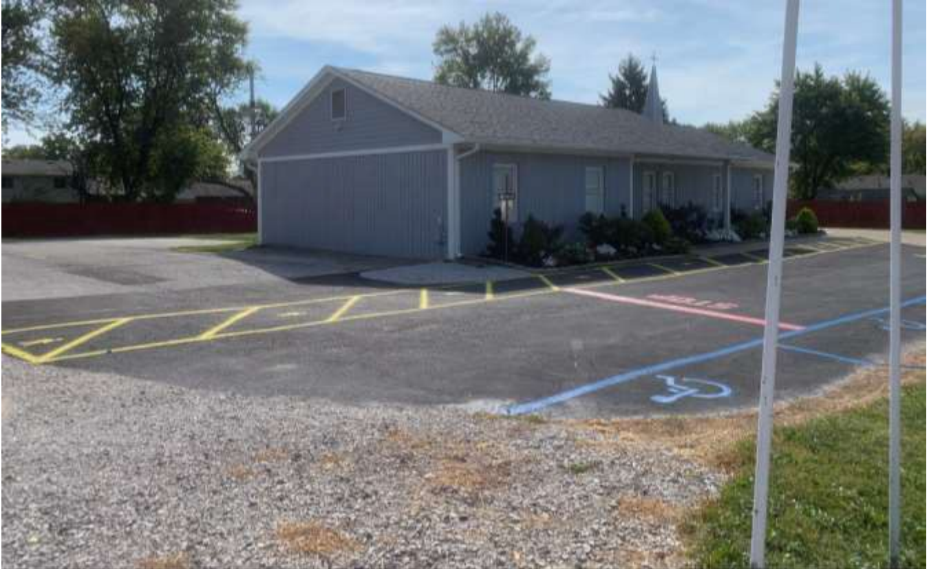
Photo the primary building at 2705 North Post Road used as a church.
