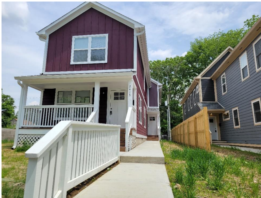
Photo 2: 2415/2417 N Rural Viewed from West
