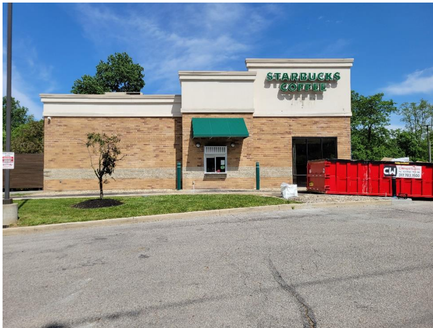
Photo 2: Subject Site viewed from West
