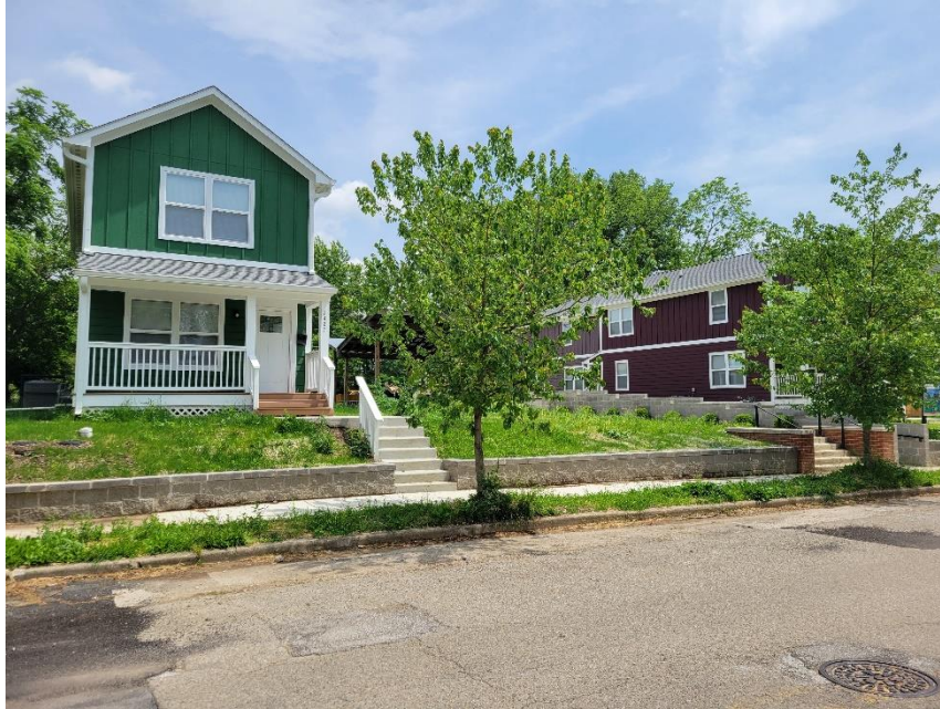
Photo 5: Both Structures Viewed from West
