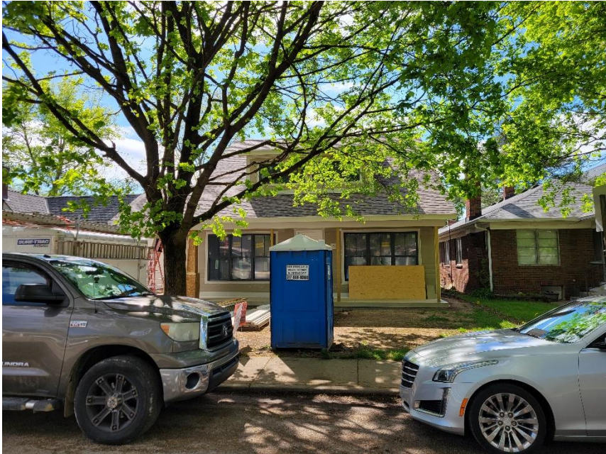
Photo 1: Subject Site from East (Carrollton Ave)
