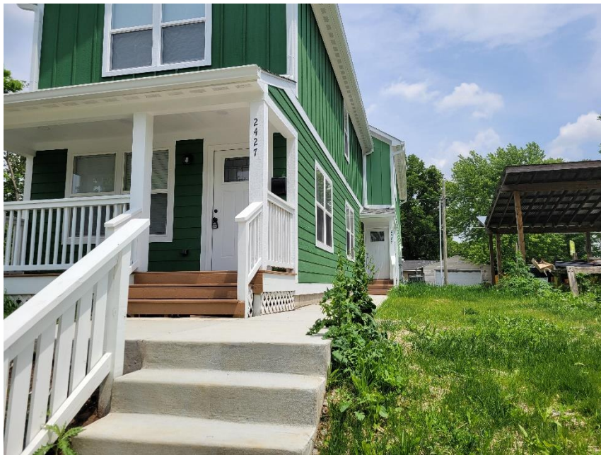
Photo 4: 2427/2429 N Rural Viewed from West
