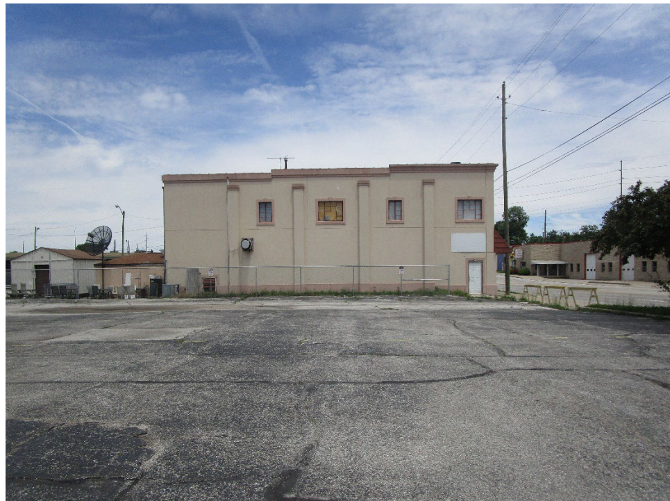
View from site looking north
