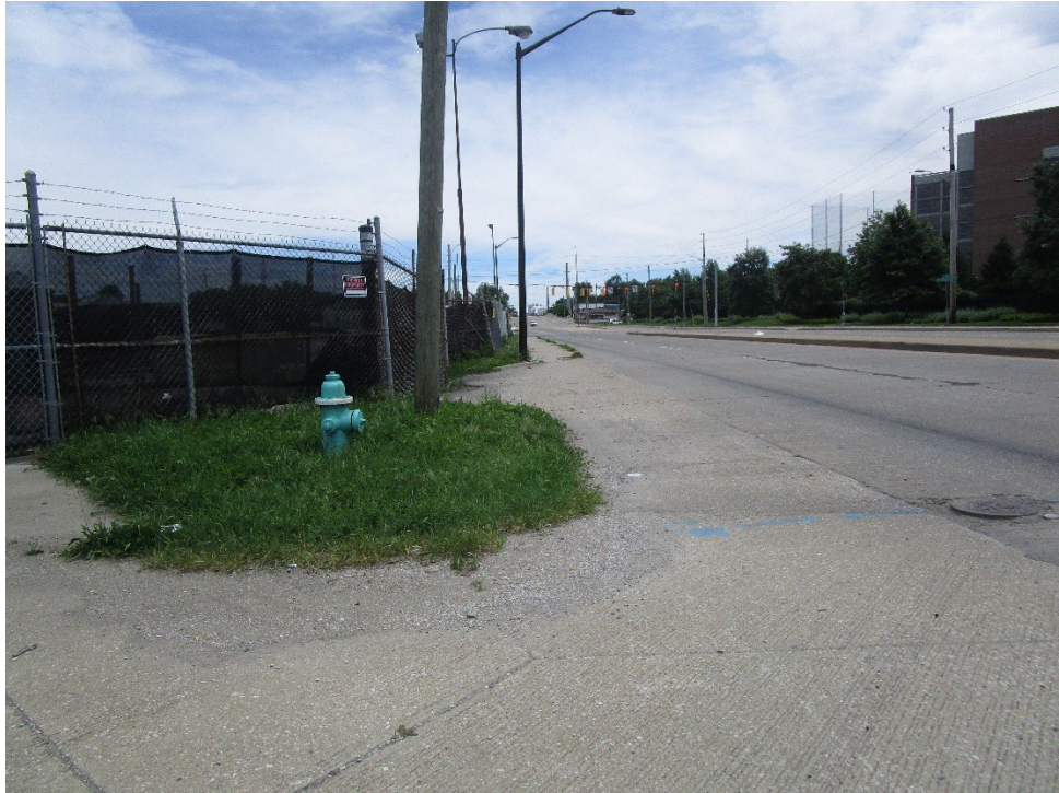
View looking east along West Morris Street
