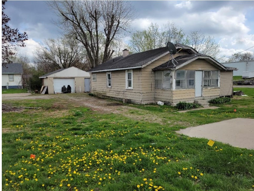
Photo 1: Existing Buildings Viewed from West
