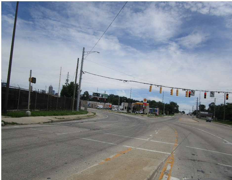
View looking east across intersection of West Morris Street and Kentucky Avenue
