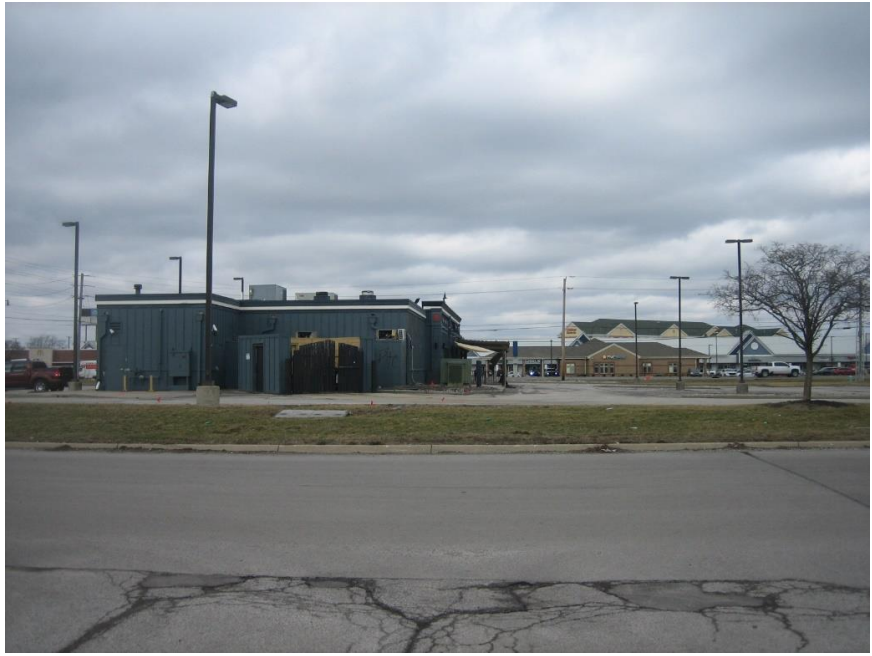
Subject site, existing building to be demolished, looking southeast.
