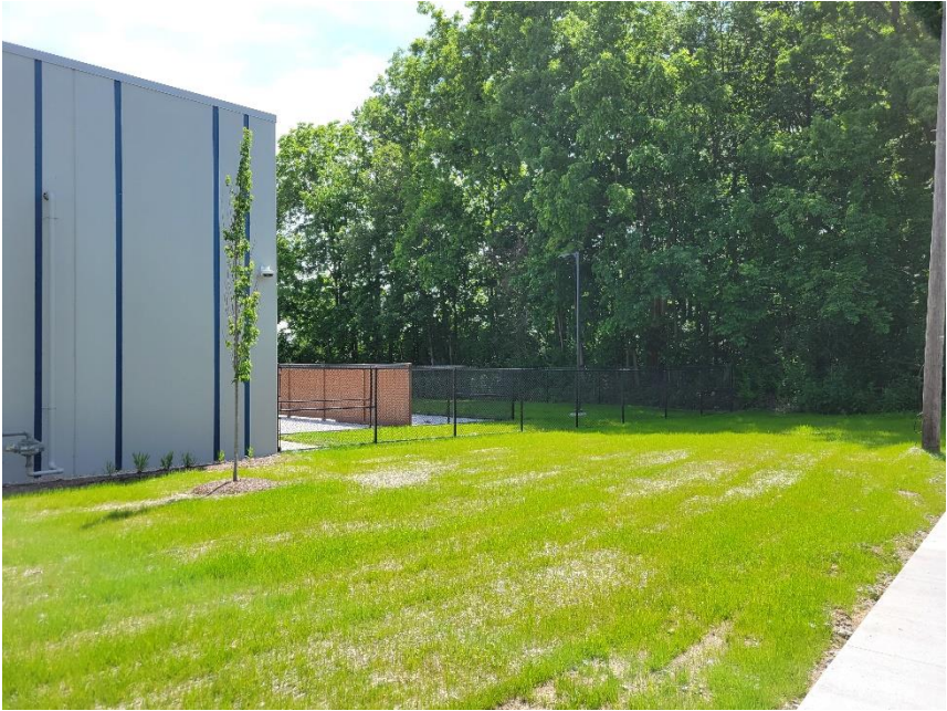
Photo 6: Northwestern Portion of Subject Site
