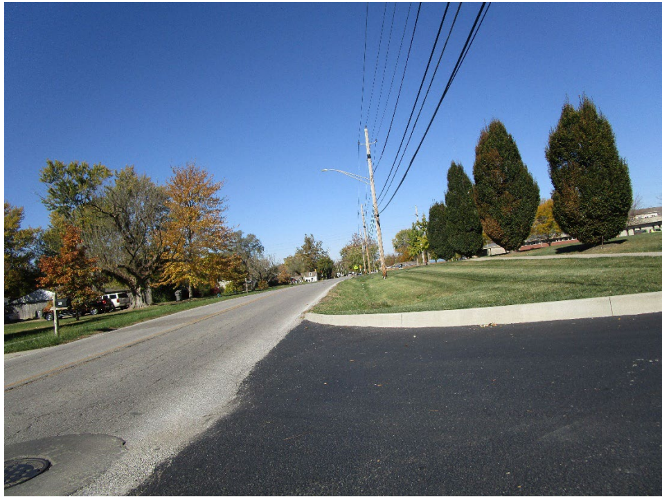
View looking north along North Ritter Avenue
