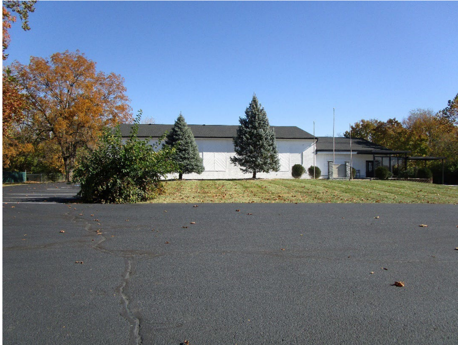
View of site looking east
