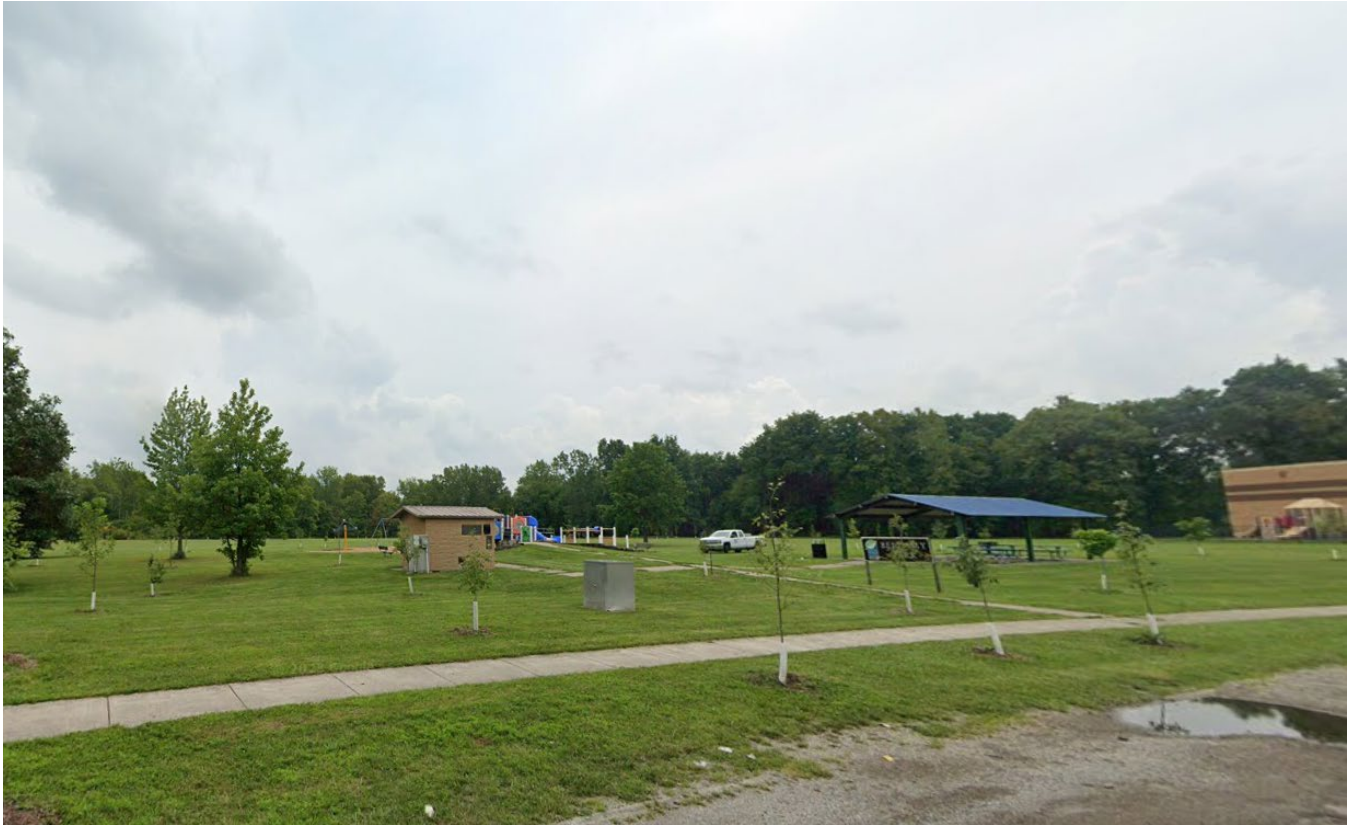
Photo of the exiting park looking southeast.
