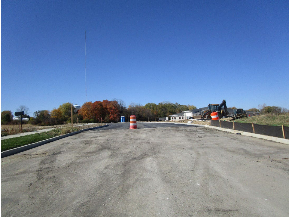
View looking west along private drive
