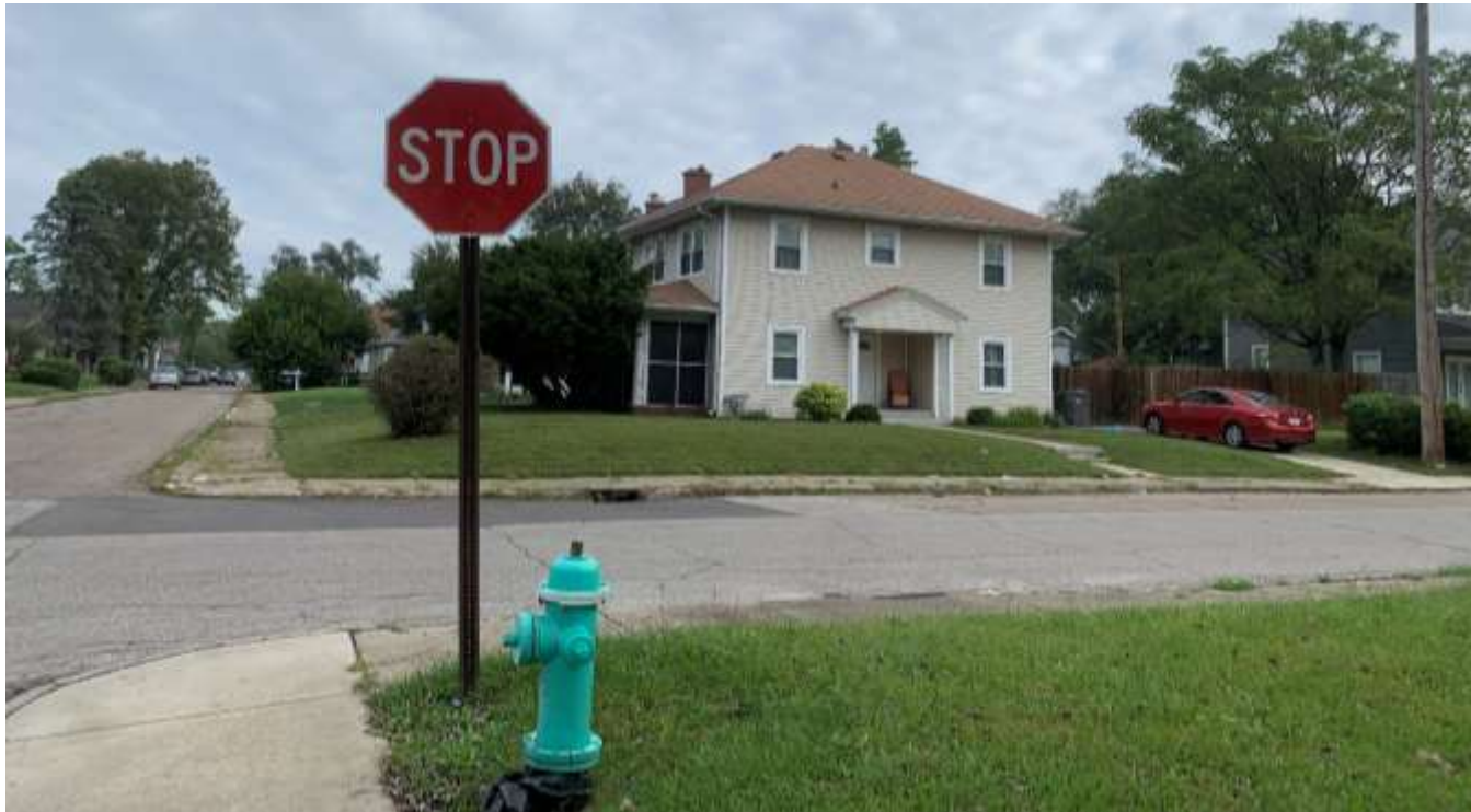
Photo of a single-family dwelling north of the site.
