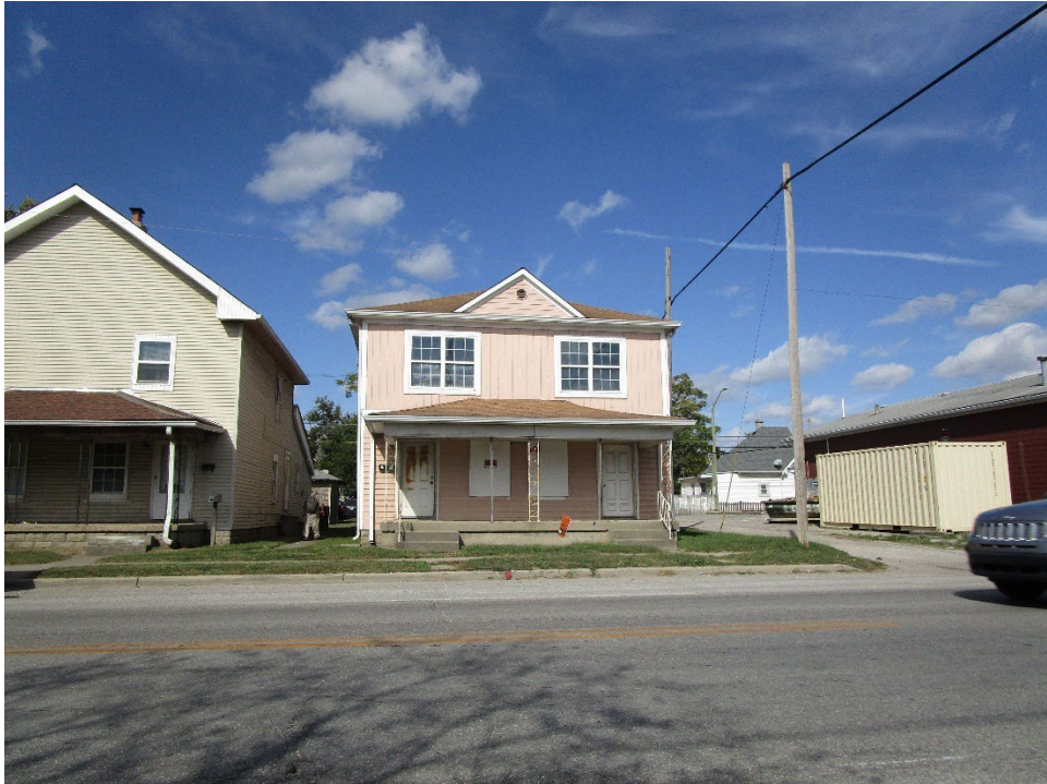
View of site looking north across English Avenue
