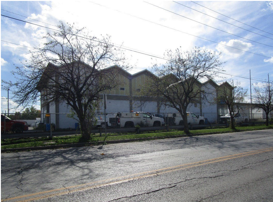
View from site looking south across English Avenue
