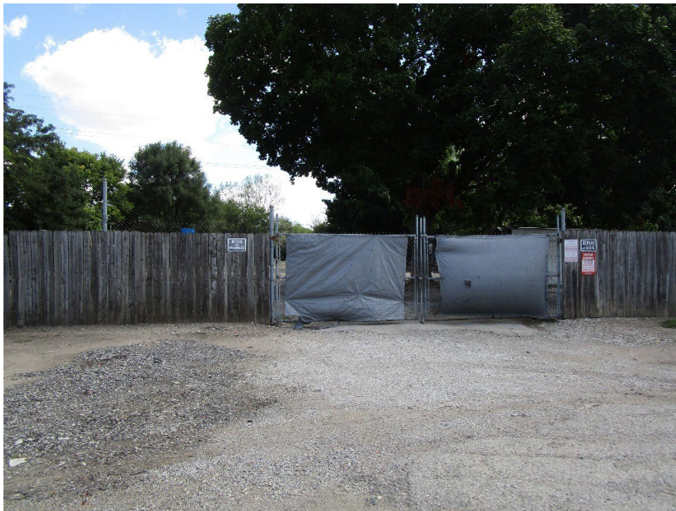
View of site looking west at entrance
