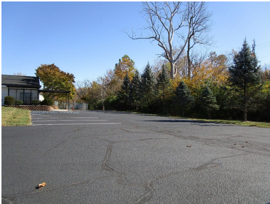
View of site looking southeast
