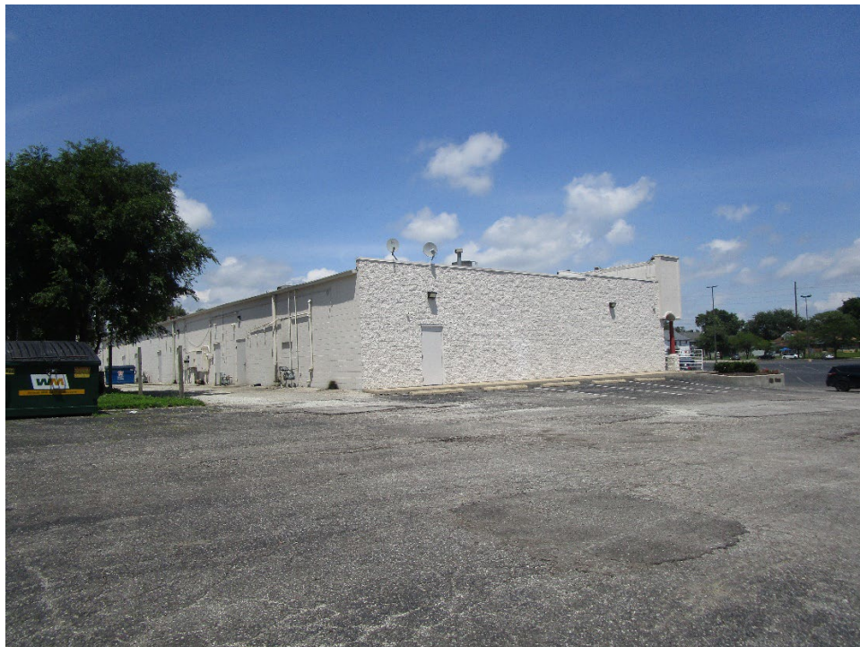
View from site looking northeast
