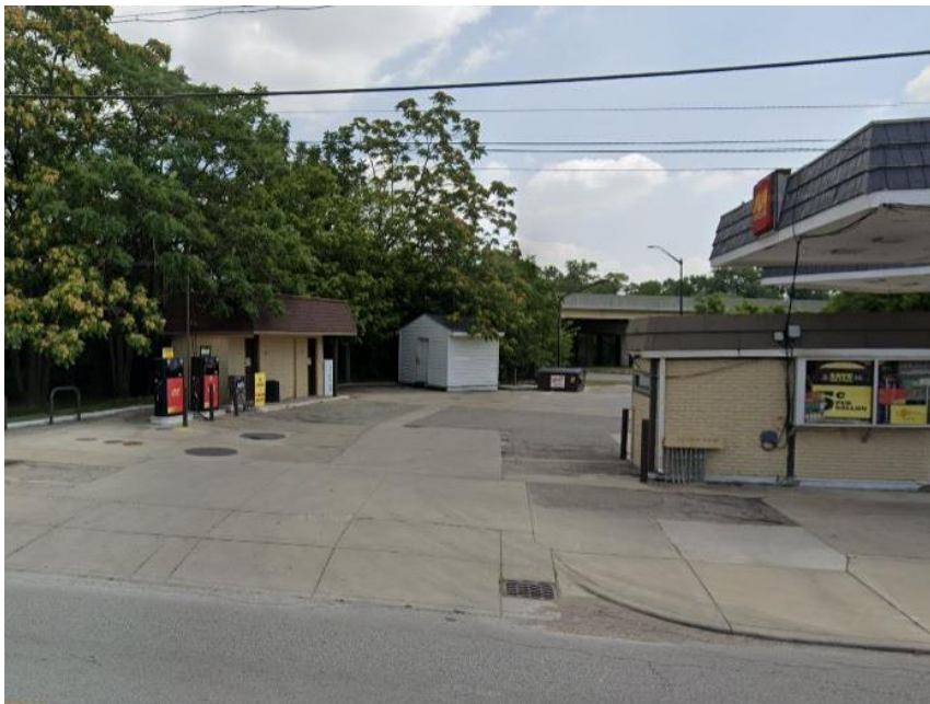
Photo 4: Subject Site from West (taken August 2023)
