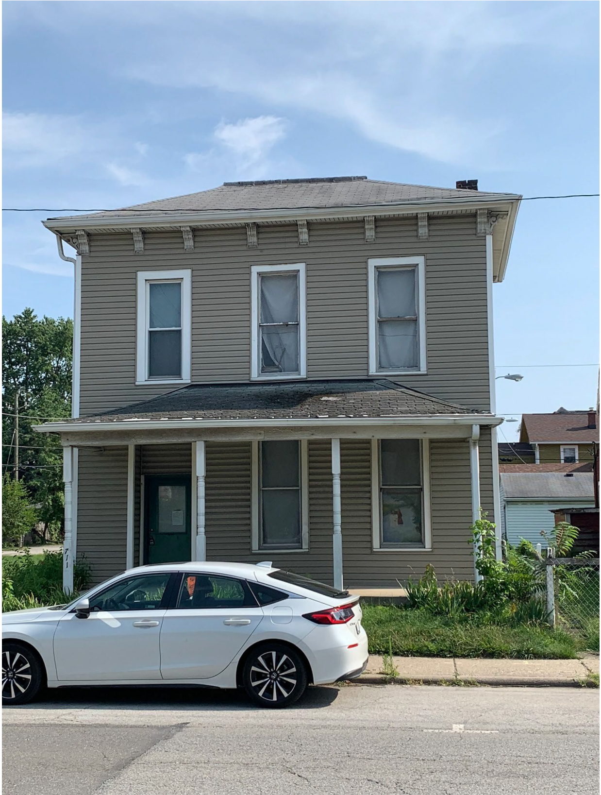
Existing structure at 711 East McCarty Street
