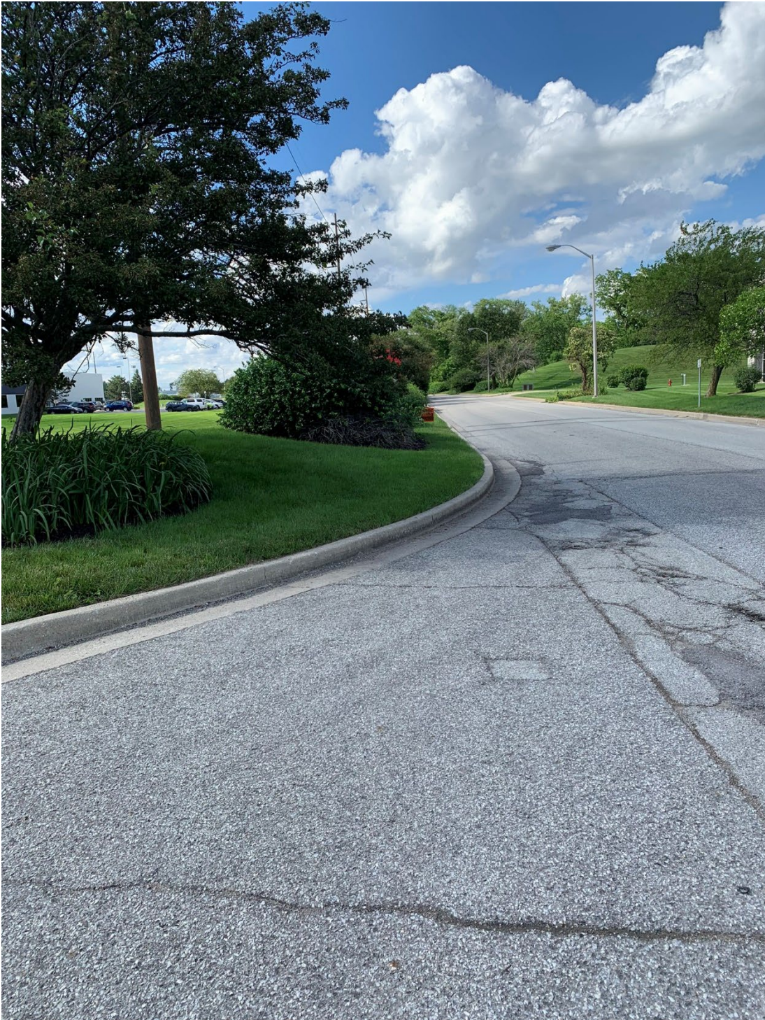
View of an internal drive connecting to Bearing Drive looking north
