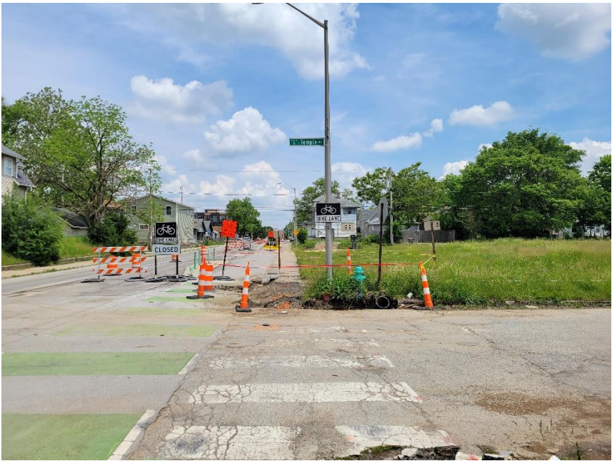
Photo 3: Existing Sidewalk & Bike Lane along New York Street
