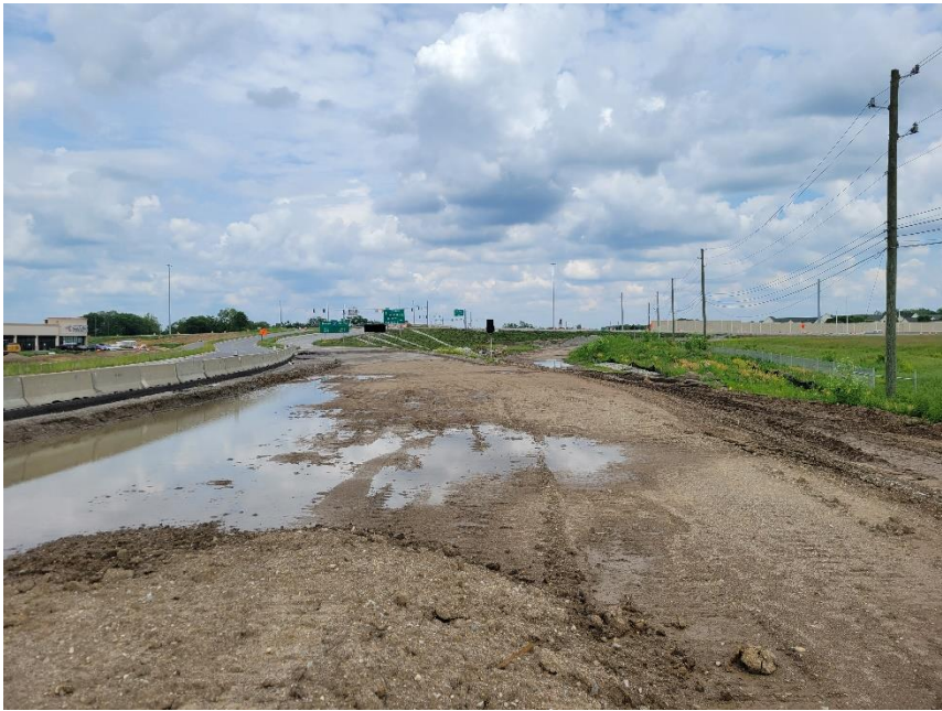
Photo 7: Southport Road Looking East Along Northern Plat Boundary
