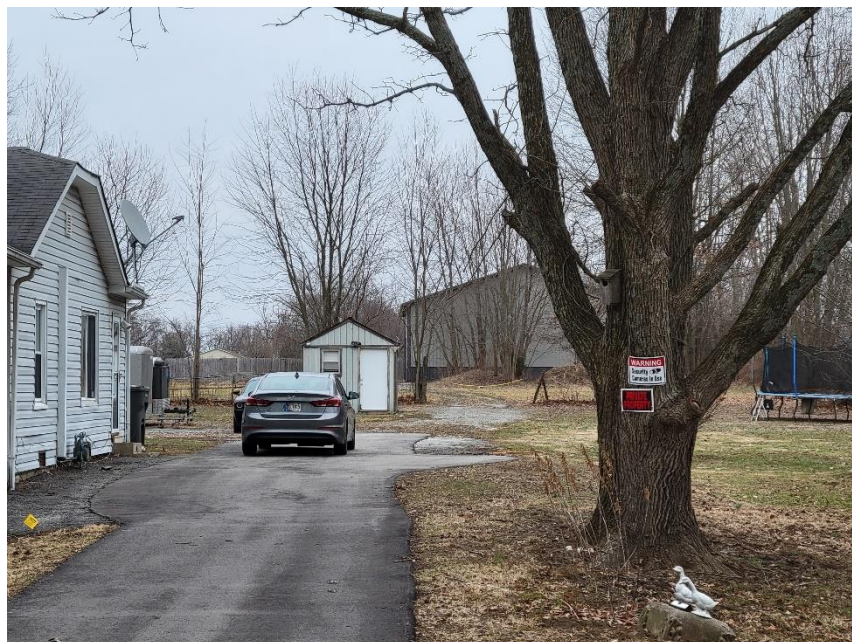
Photo 2: Newer Detached Structure Viewed from Stanley
