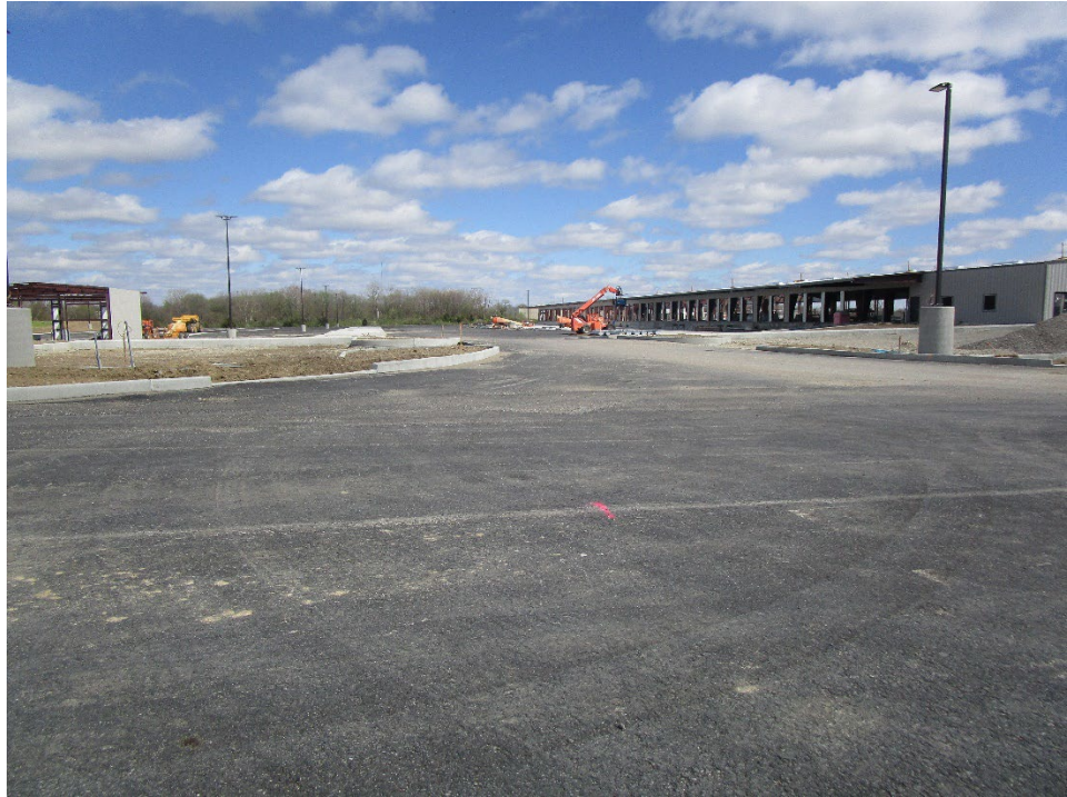
View looking east across Fintail Drive at adjacent land under development
