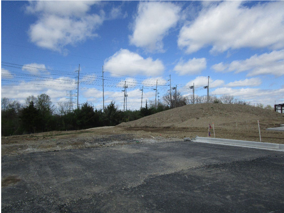
View looking northeast across Fintail Drive at adjacent land under development
