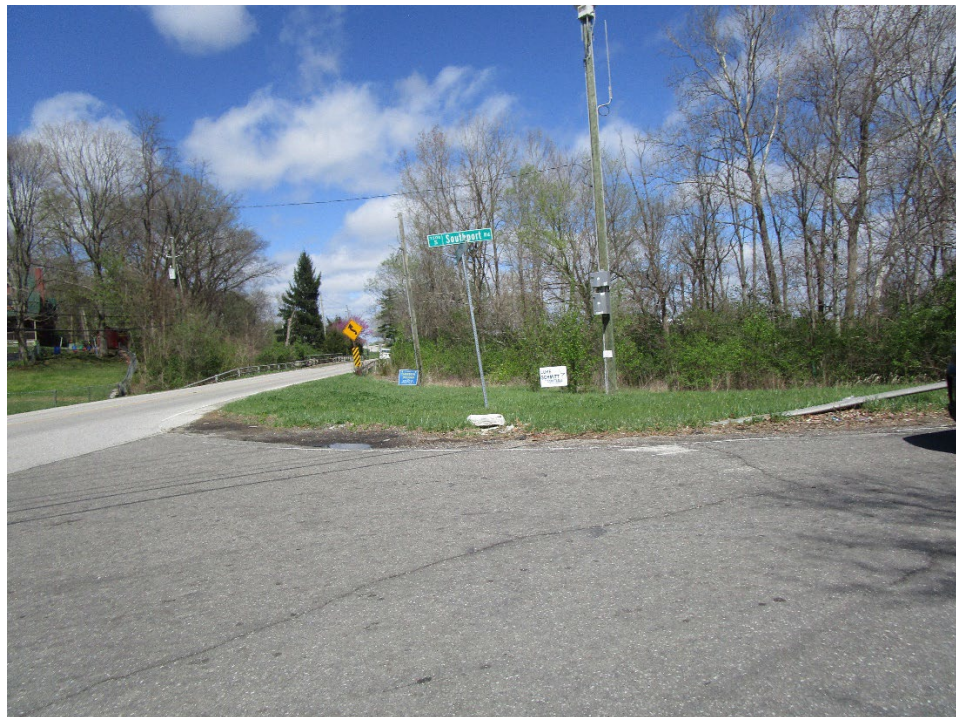
View looking north across intersection of South Mooresville Road and West Southport Road
