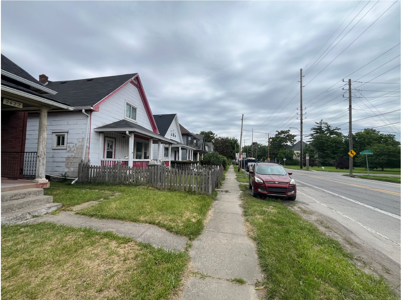
Photo 2: Looking east from 2422 Prospect Street
