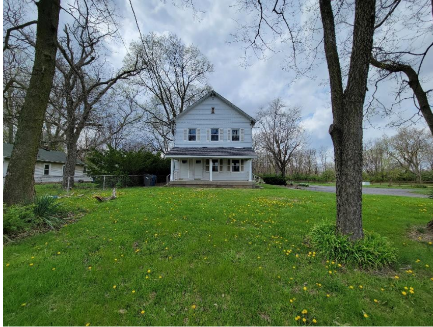
Photo 1: Subject Site Viewed from West
