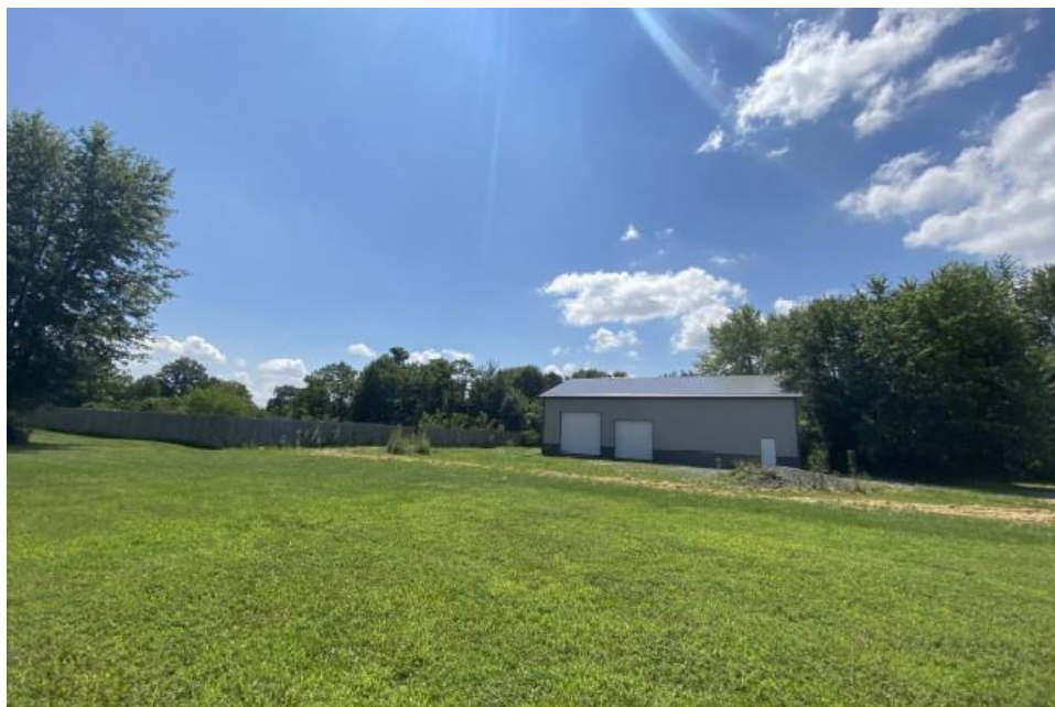
Photo 4: Newer Detached Structure Viewed from North (August 2025)
