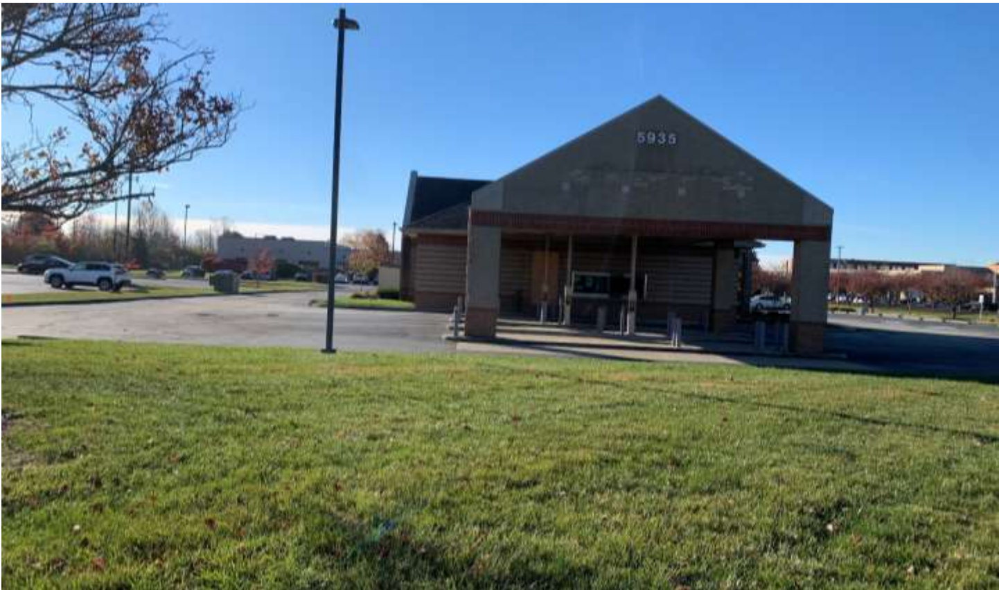
Photo of the existing north building façade.
