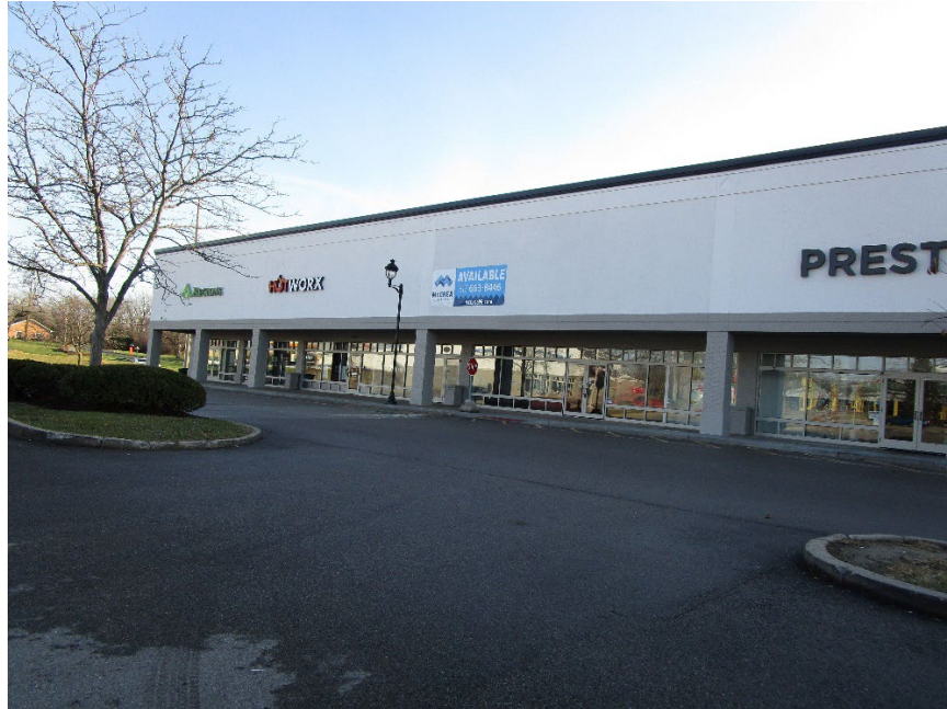
View of site looking southeast at available tenant space
