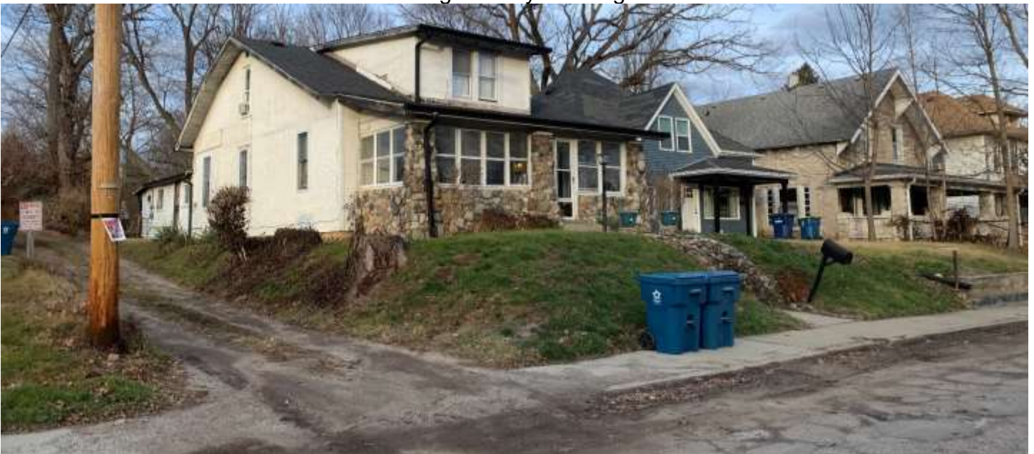
Photo of the single-family dwelling to the east.
