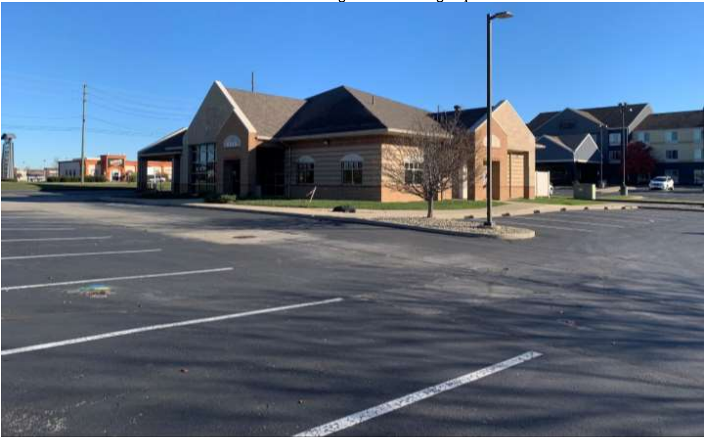
Photo of the existing west building façade.
