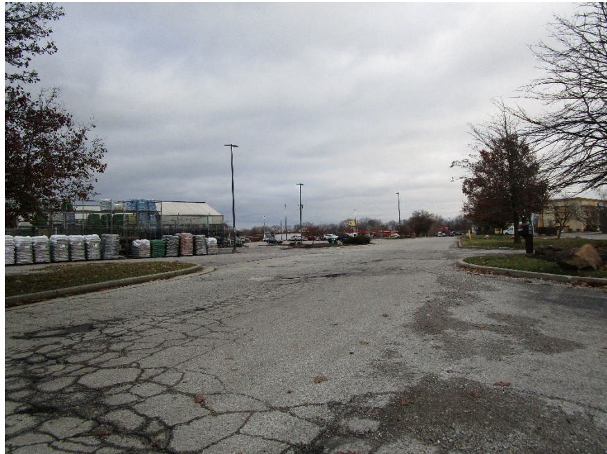
View from site looking northeast across Post Drive
