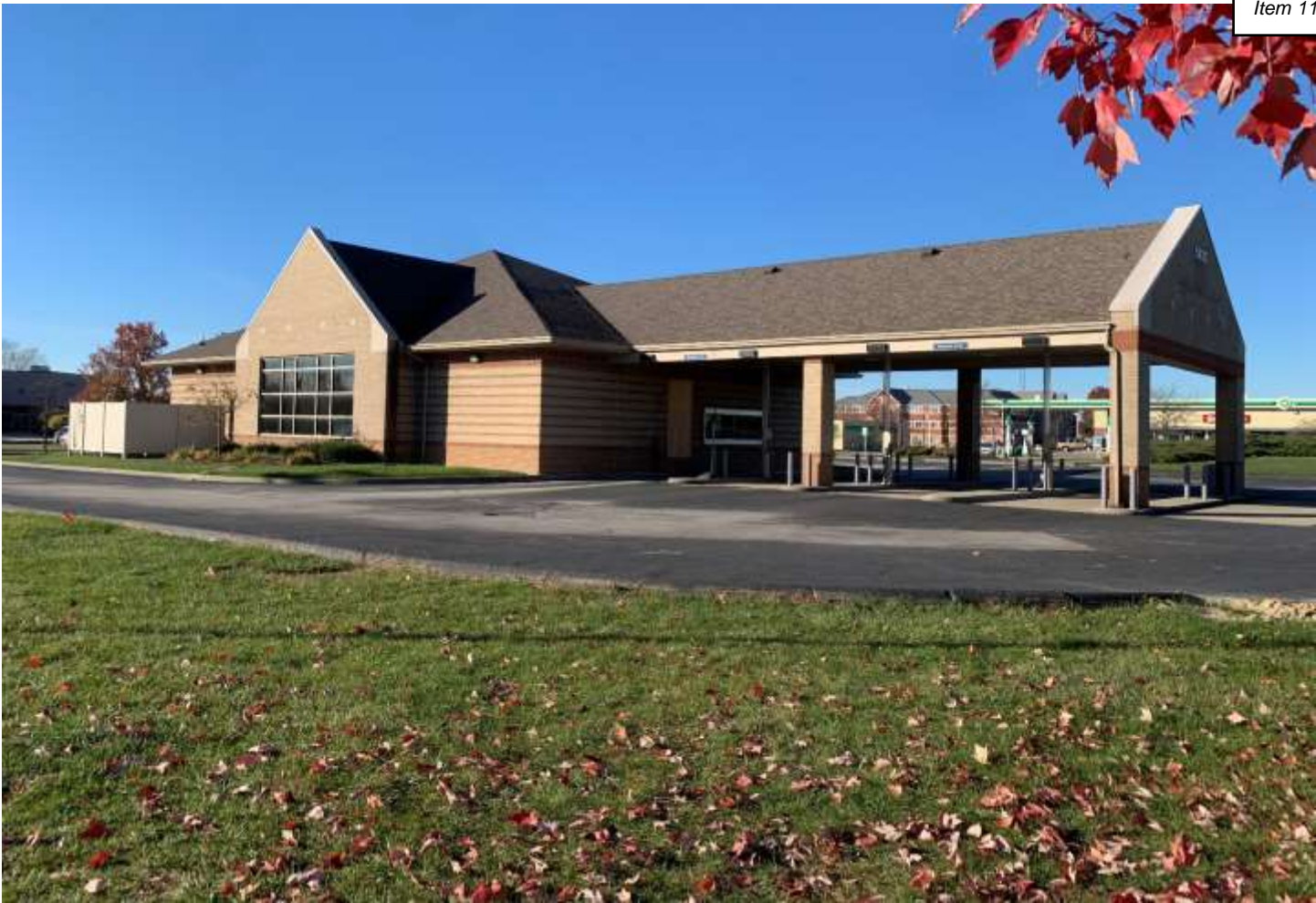
Photo of the existing east building façade.
