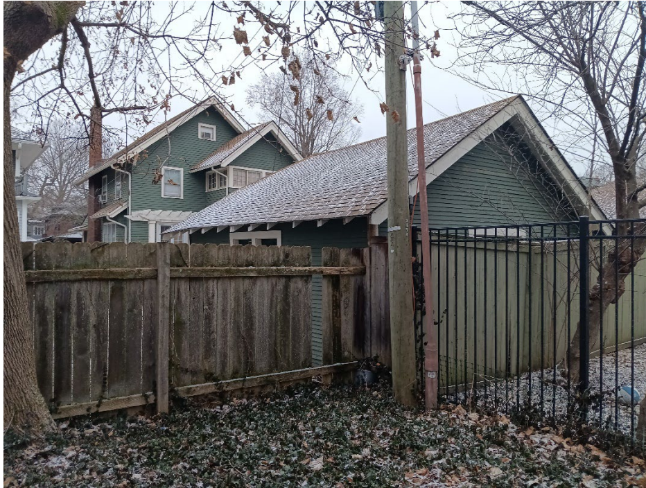
Exhibit 11: Garage of neighbor to the northwest.
