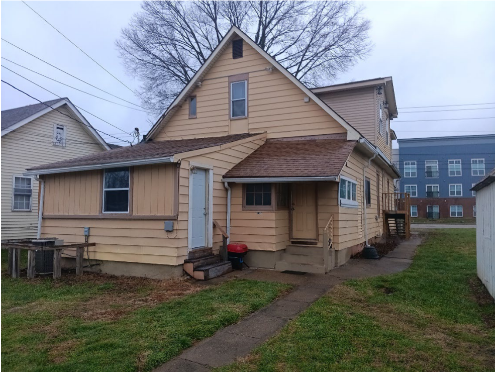
Exhibit 9: Back of 2927 West Washington Street.
