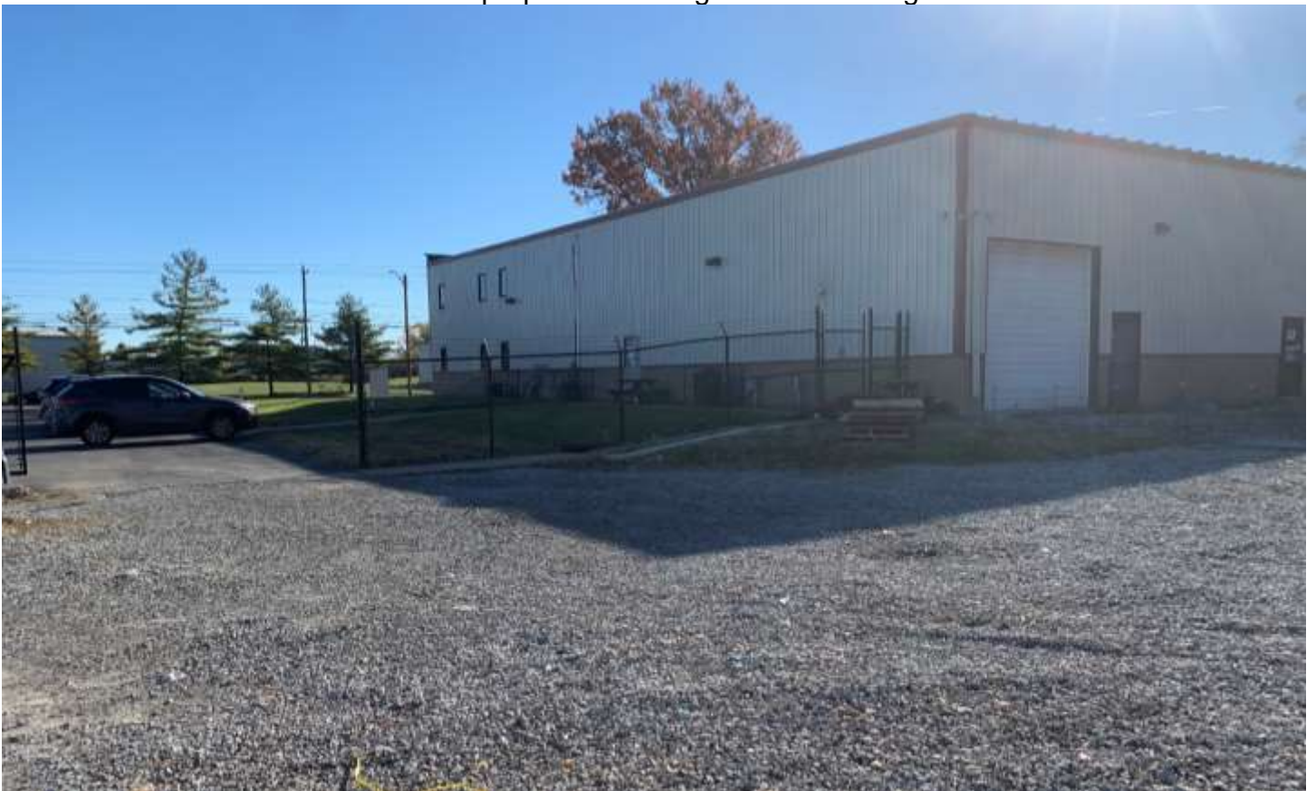
Photo of the northern building façade.
