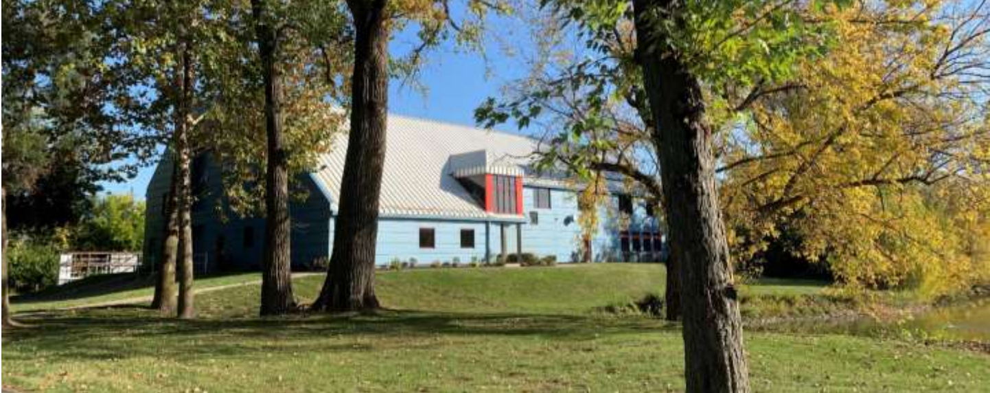
Photo of the second existing commercial building on site.
