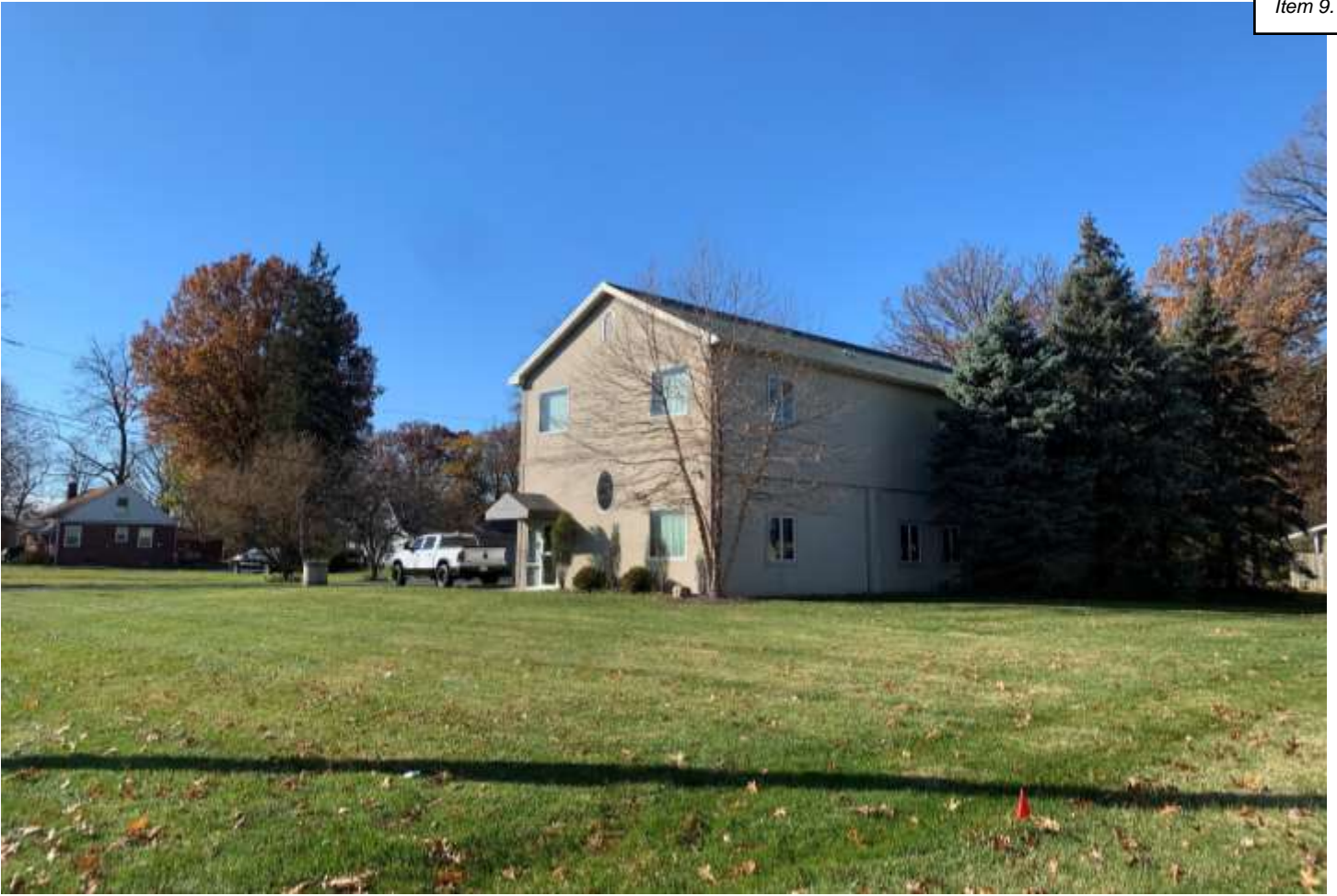
Photo of the office buiding south of the site.
