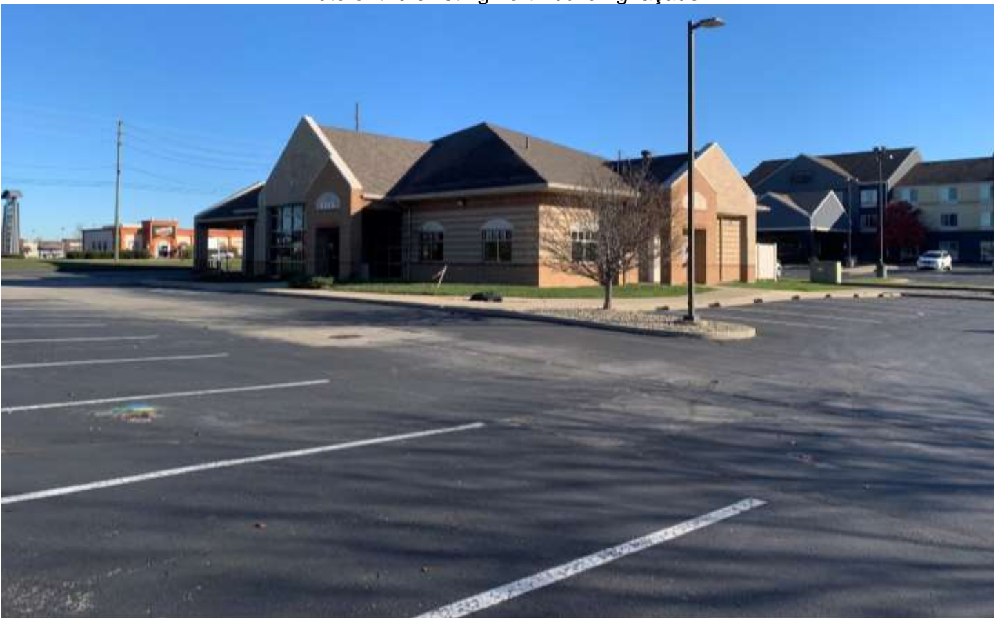
Photo of the existing west building façade.
