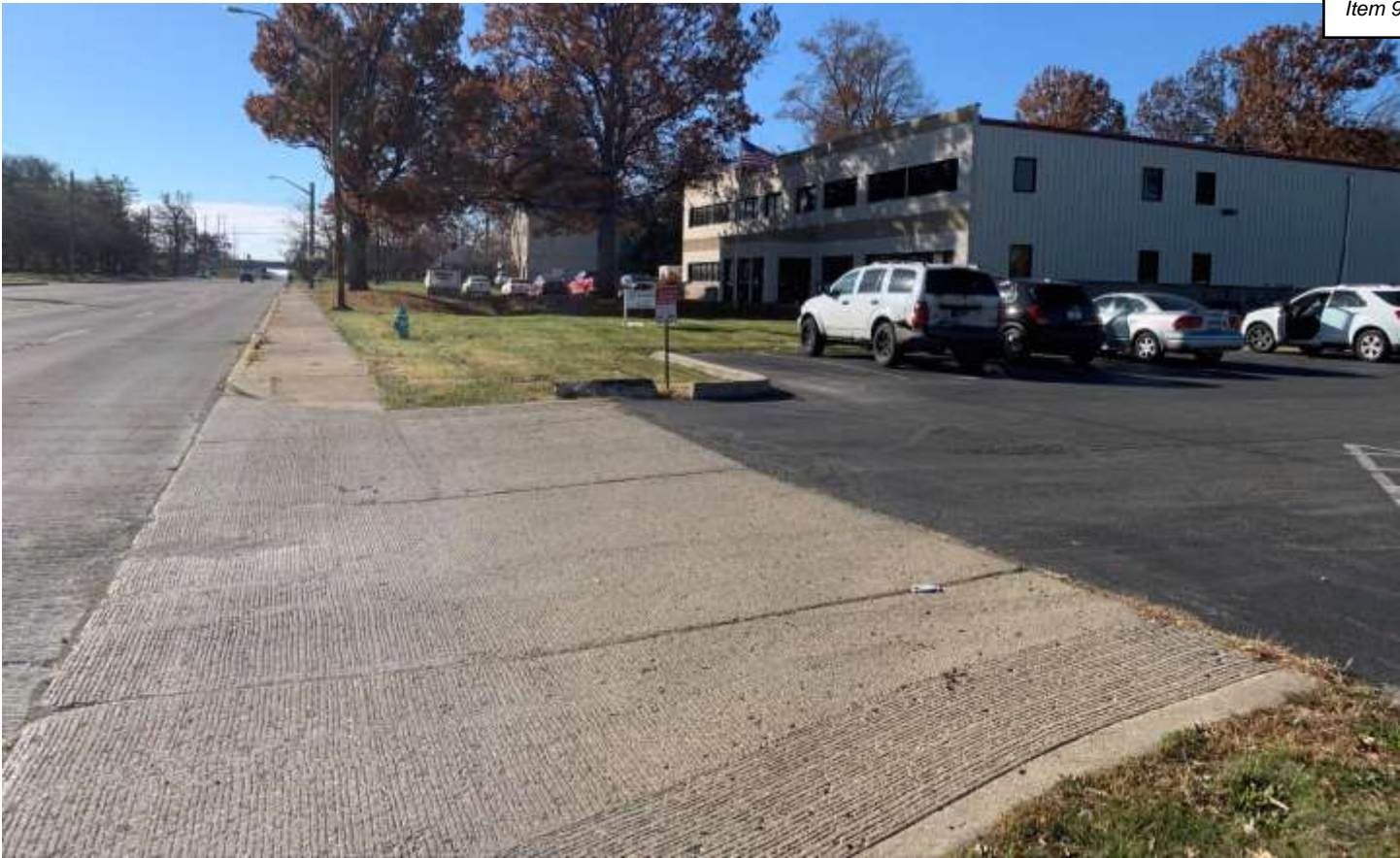
Photo of the street frontage along Arlington Avenue.
