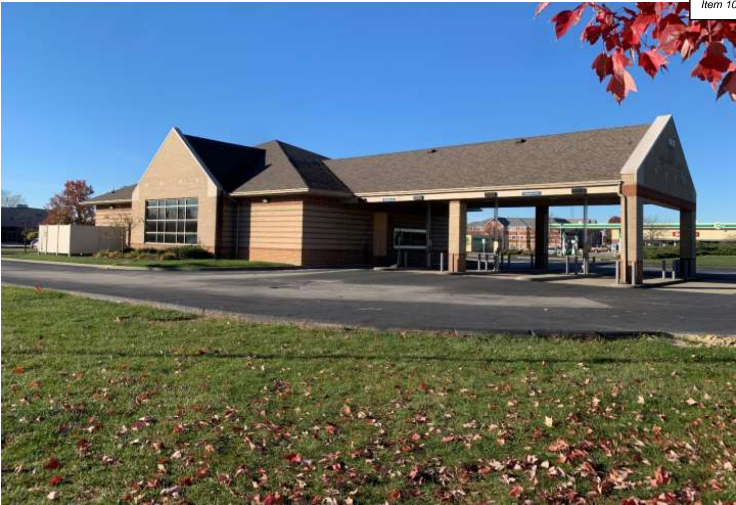
Photo of the existing east building façade.
