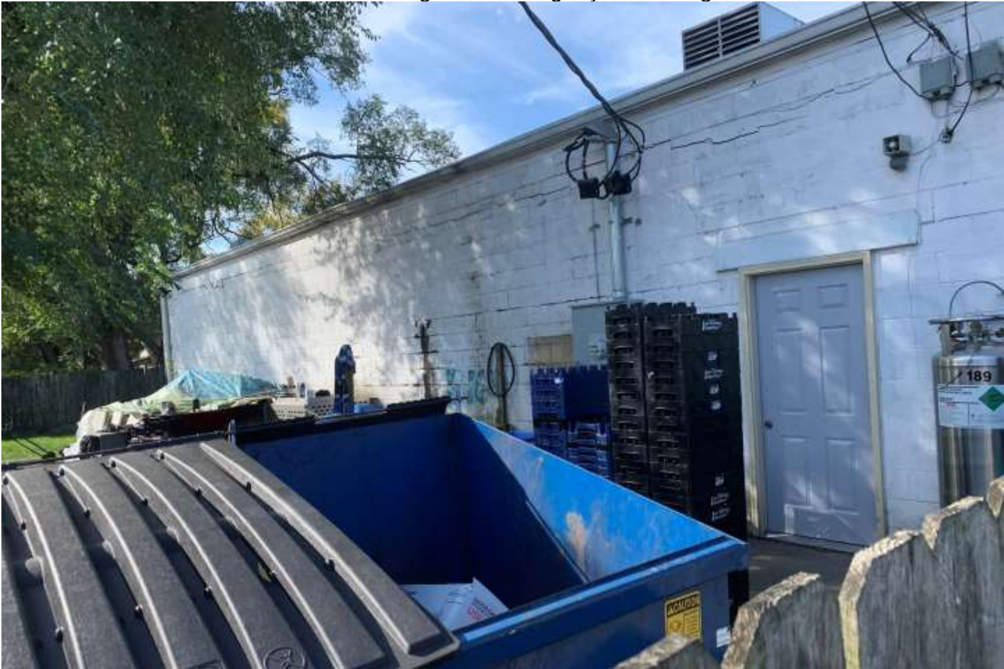
Photo of the existing east building façade looking south.
