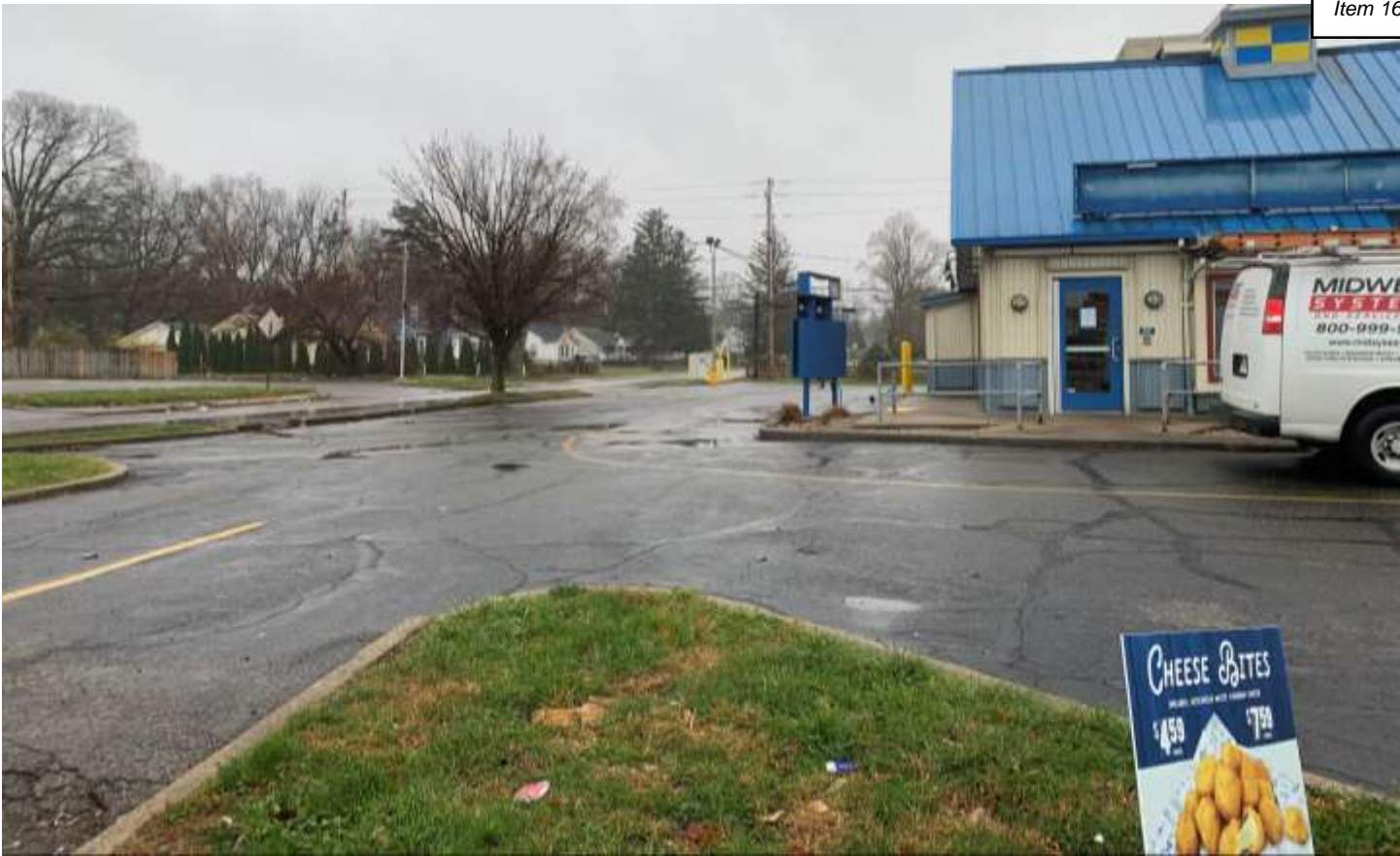
Photo of the eastern side of the property looking south.
