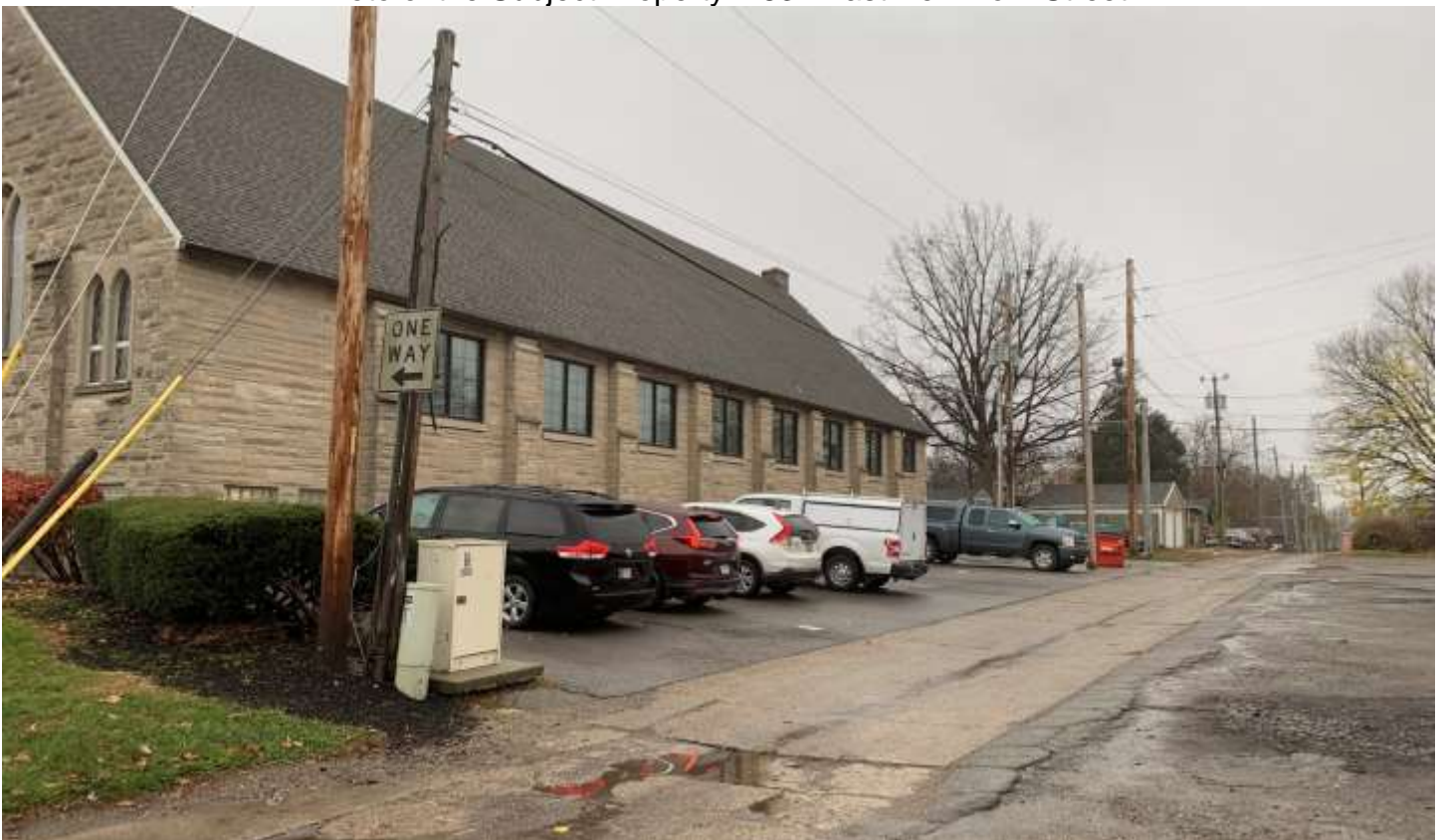
Photo of the on-site parking west of the building.
