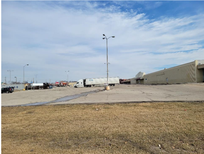
Photo 5: View from East along Emerson
