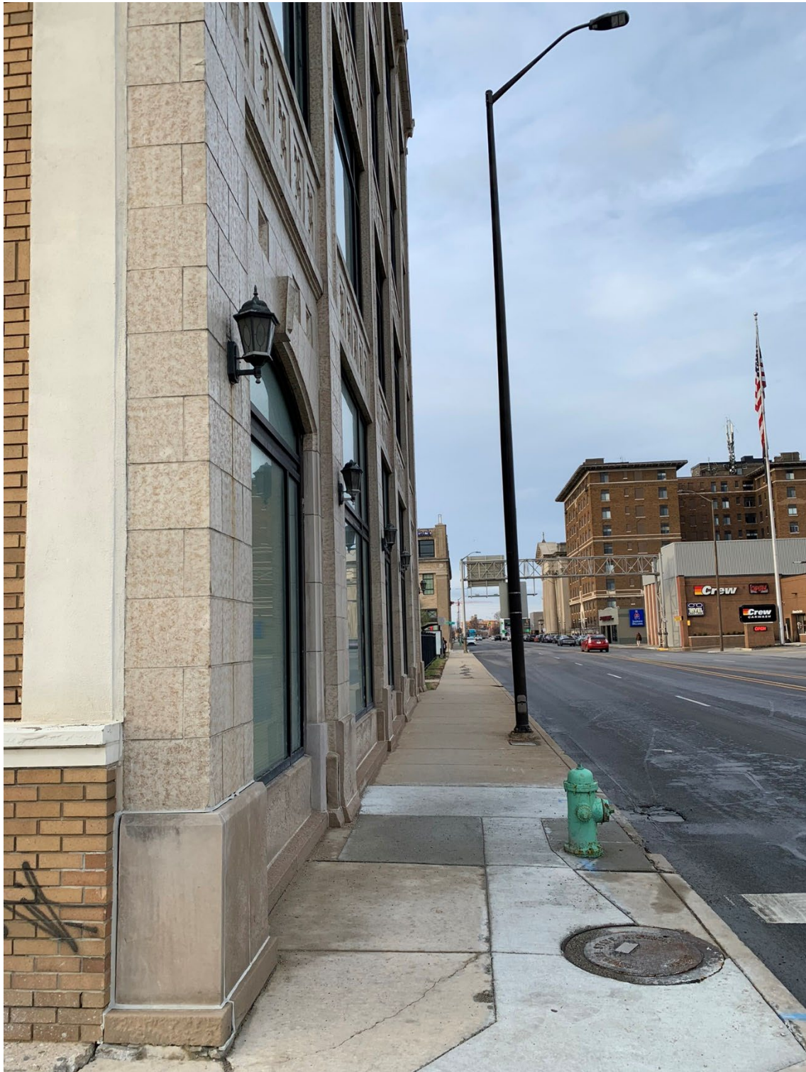
View along Meridian Street looking north
