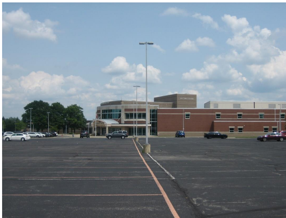
Subject site public high school, looking east.
