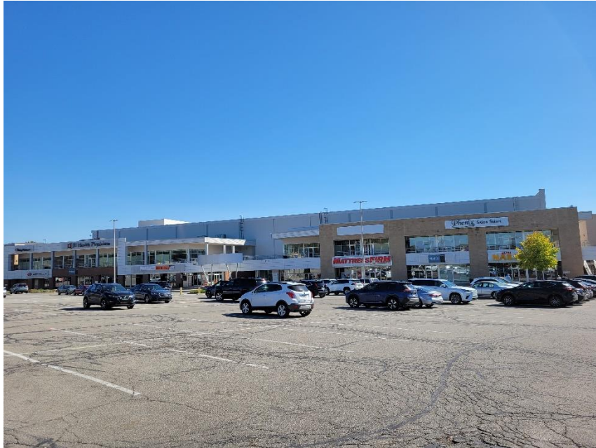
Photo 5: Adjacent Property to Southeast
