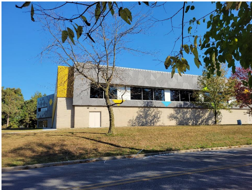
Photo 4: Adjacent Property to North
