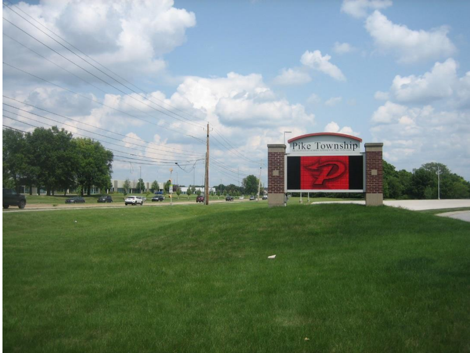
Existing subject site sign with electronic variable message center, looking east.
