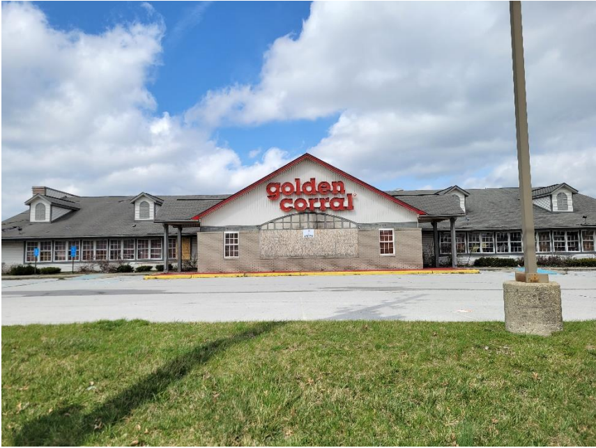
Photo 2: Property Currently Occupying Block A
