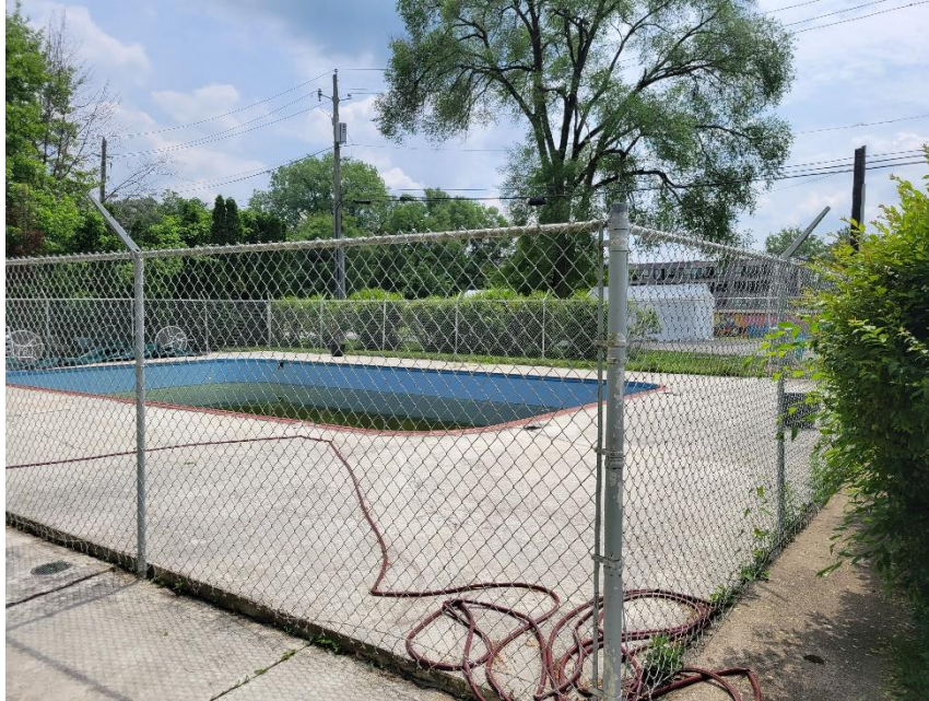
Photo 3: Pool from Northwest
