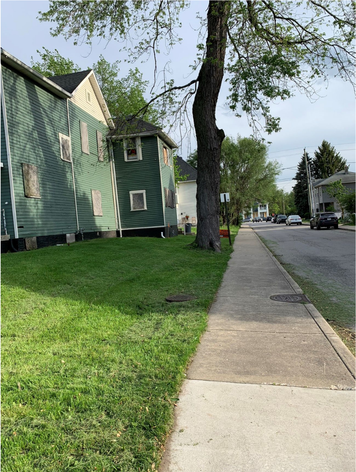
View of existing dwelling and sidewalk along Laurel Street
