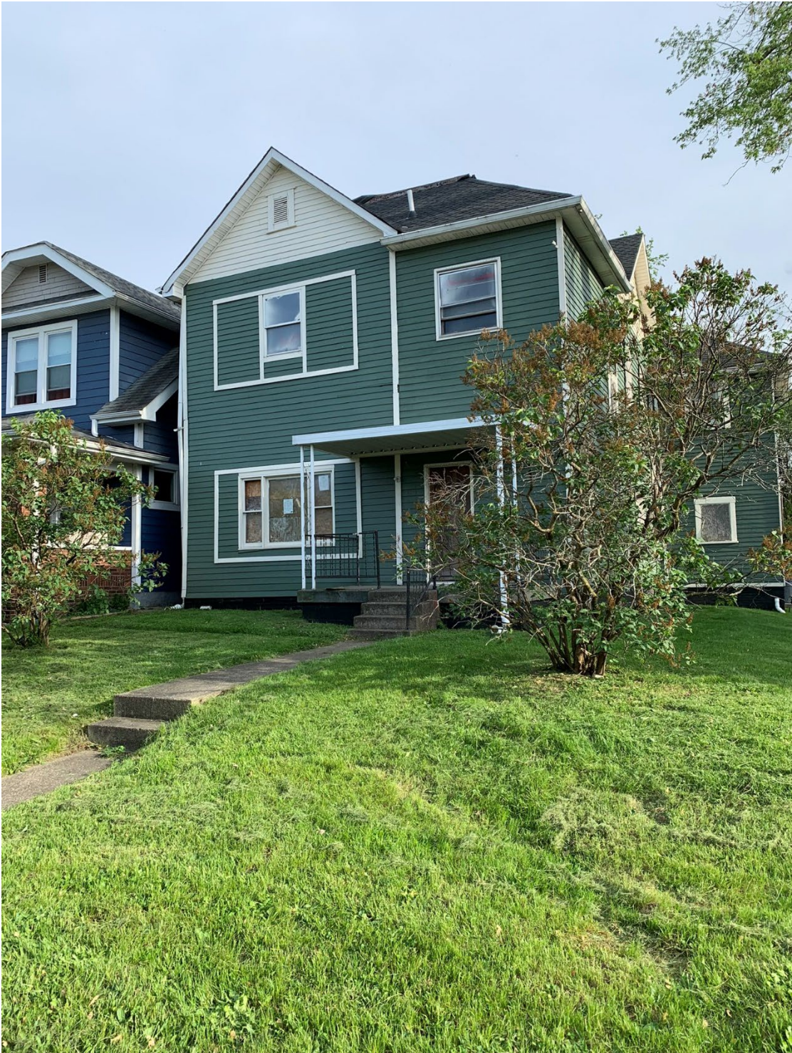
View of existing dwelling along Woodlawn Avenue
