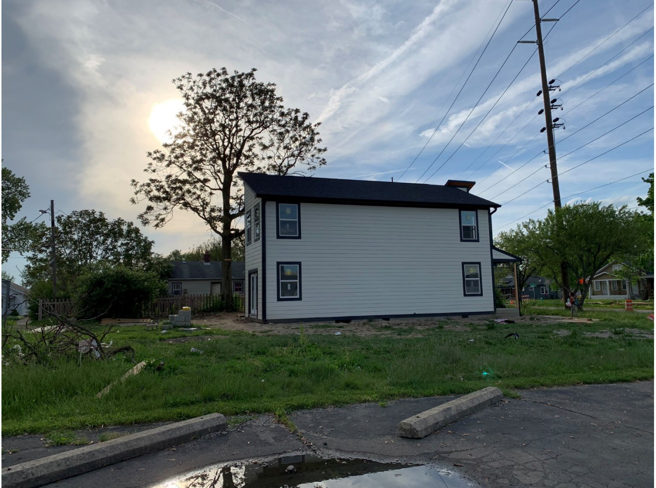
View of existing two-family dwelling from the east
