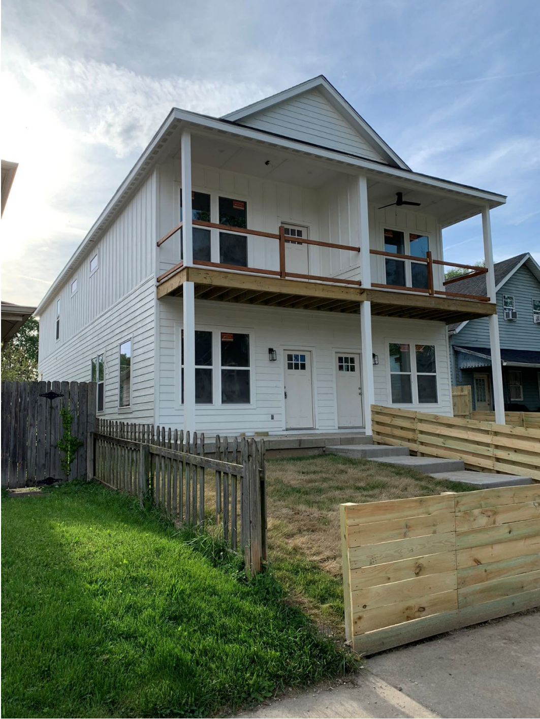
View of existing dwelling
