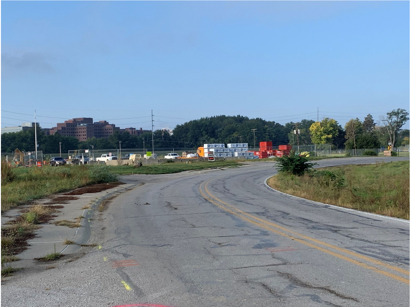
Proposed vacation area – construction material storage in background for bridge construction
