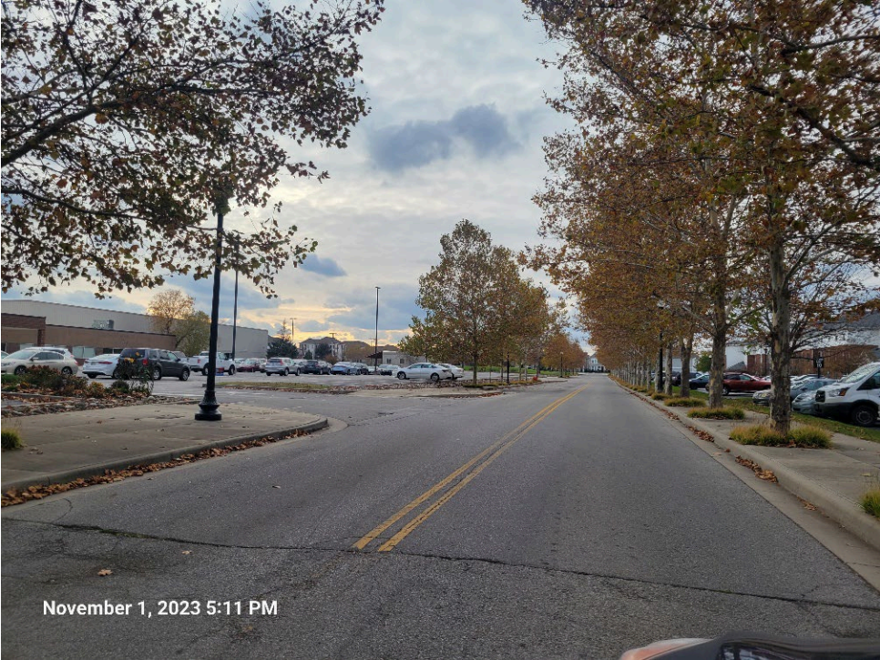
Figure 2 - Hawkins Road looking west
