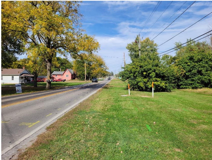
Photo 4: Shelby Frontage Looking North from Lot 2 Southern Edge
