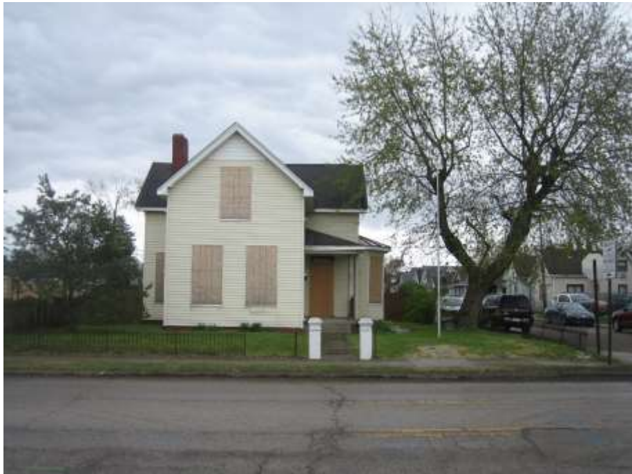
Adjacent single family dwelling use to the east, zoned C-3
