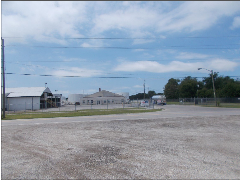
Looking west across Raceway Road at the neighbor to the west.
