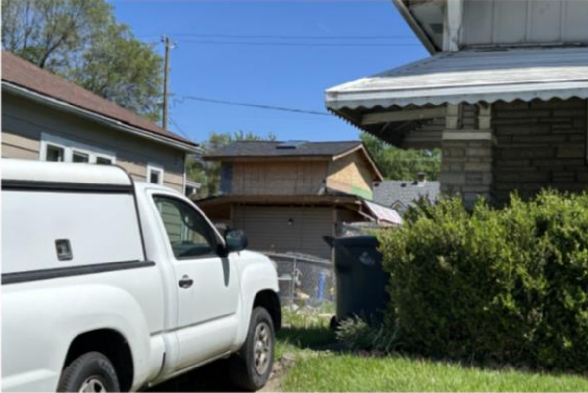
Photo 2: A BNS inspector's photo of a play structure seemingly encroaching into the side yard setback. Play structures are permitted to encroach into side yard setbacks.
