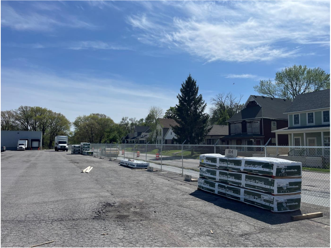
Photo 5: Showing additional material stored along fence line. Materials in far back will need to be stepped down remain below fence height.
