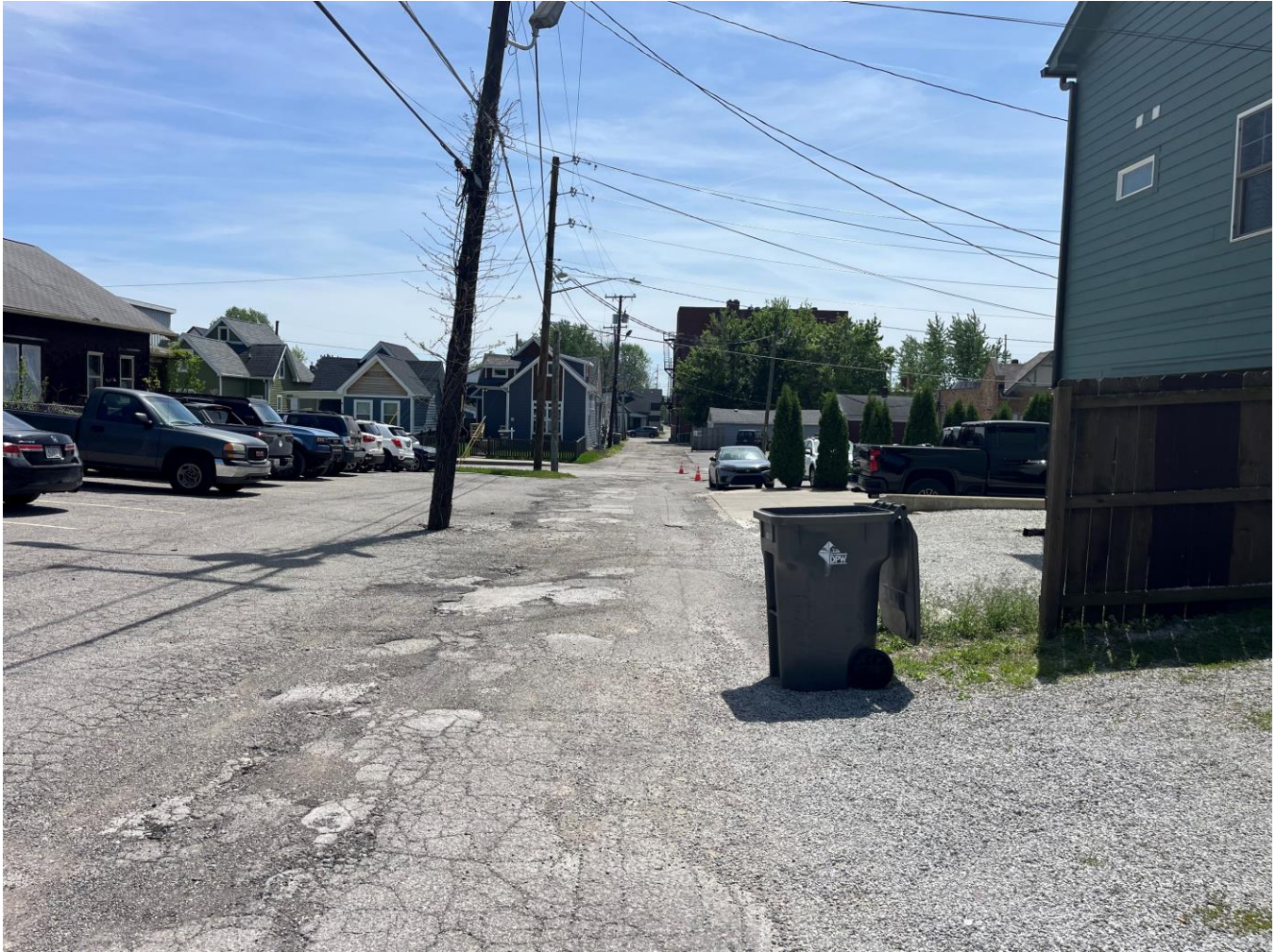
Photo 8: View from alley looking south
