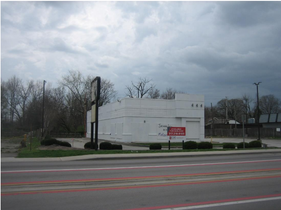
Adjacent vacant commercial restaurant to the west, looking south.
