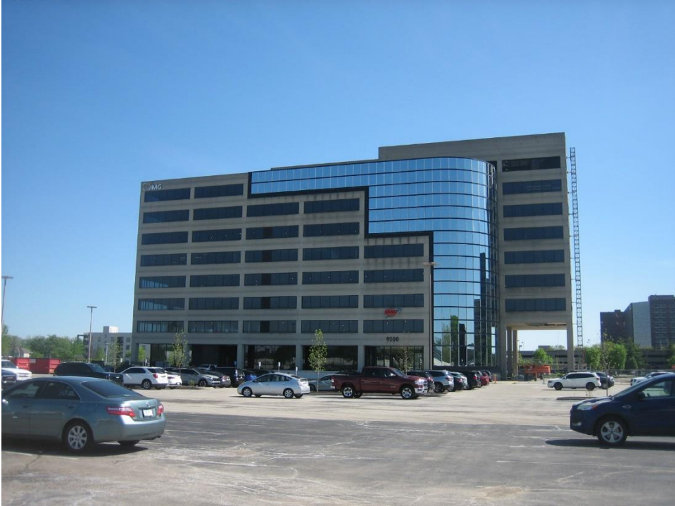
8888 Keystone Crossing building north facade, looking south (proposed sign façade).
