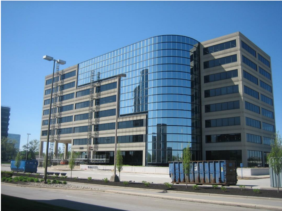
8888 Keystone Crossing building south façade, looking north.
