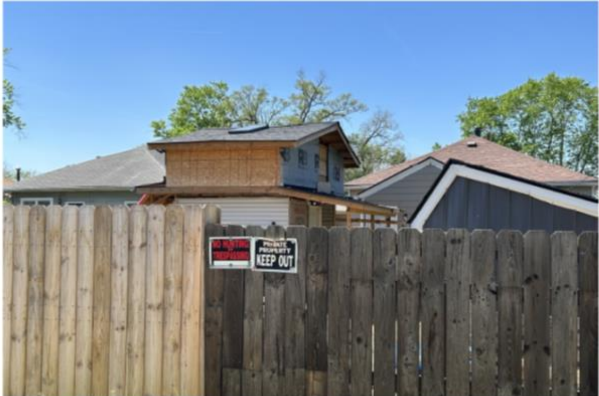
Photo 3: A BNS inspector's photo of the parcel from the rear alley.
