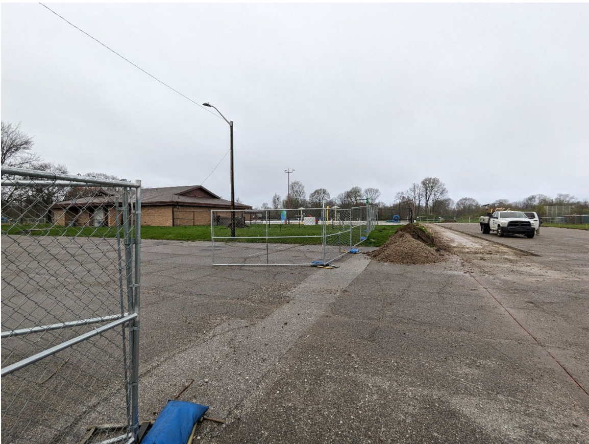
View of area of ongoing 'Basketball Project' (NE area of park)
