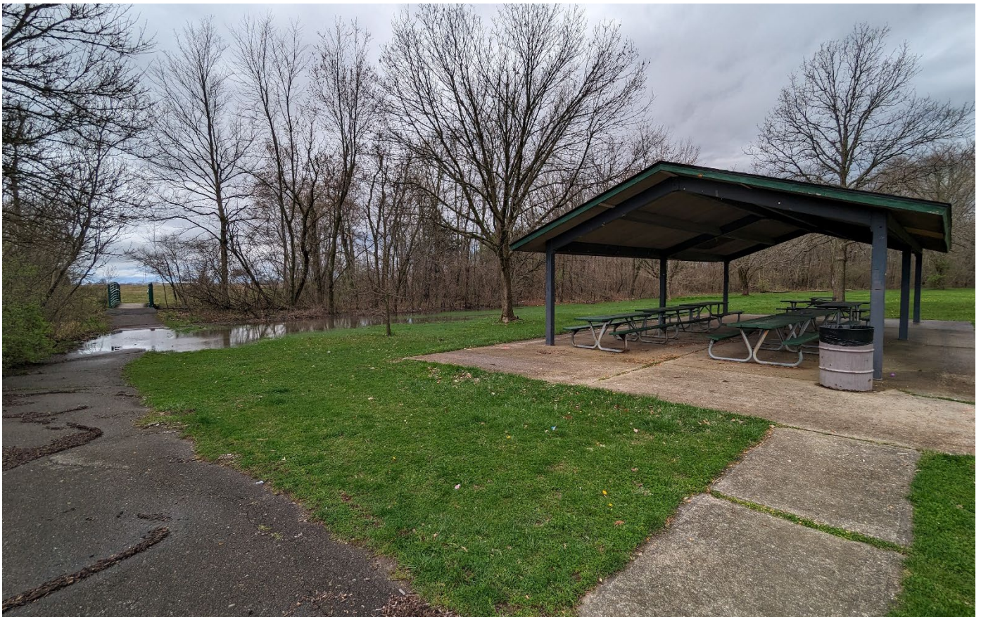
Site photo: View of existing pavilion and foot bridge over Wildcat Brook
