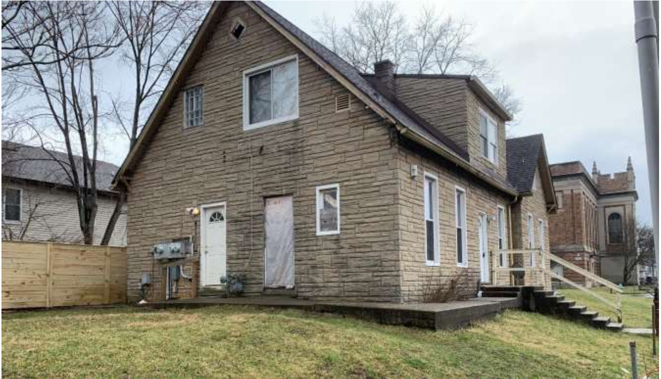
Photo of the rear building façade.
