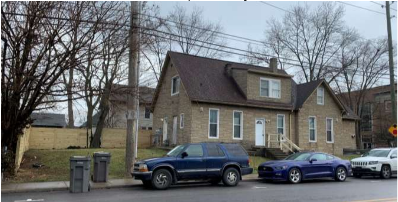
Photo of the subject site looking east.
