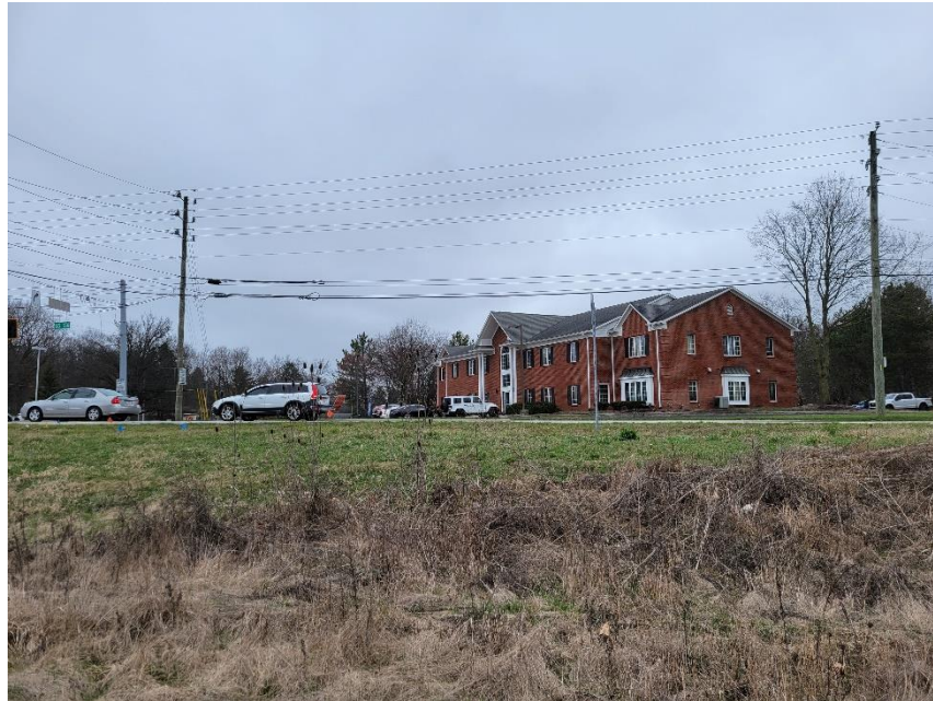
Photo 3: Adjacent Property to North of Subject Site
