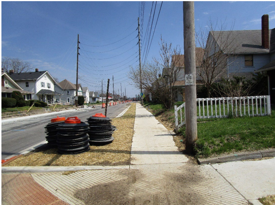
View looking east along West Morris Street
