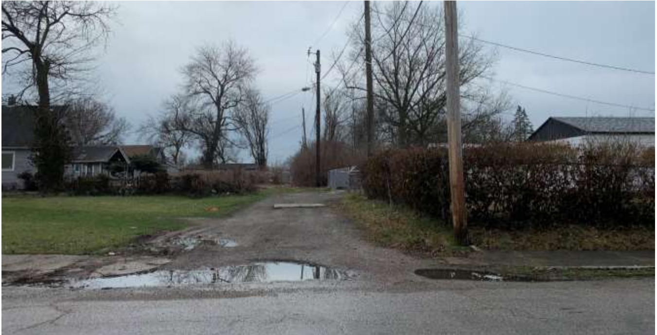
Photo of the alley east of the site looking south from 25 th Street.
