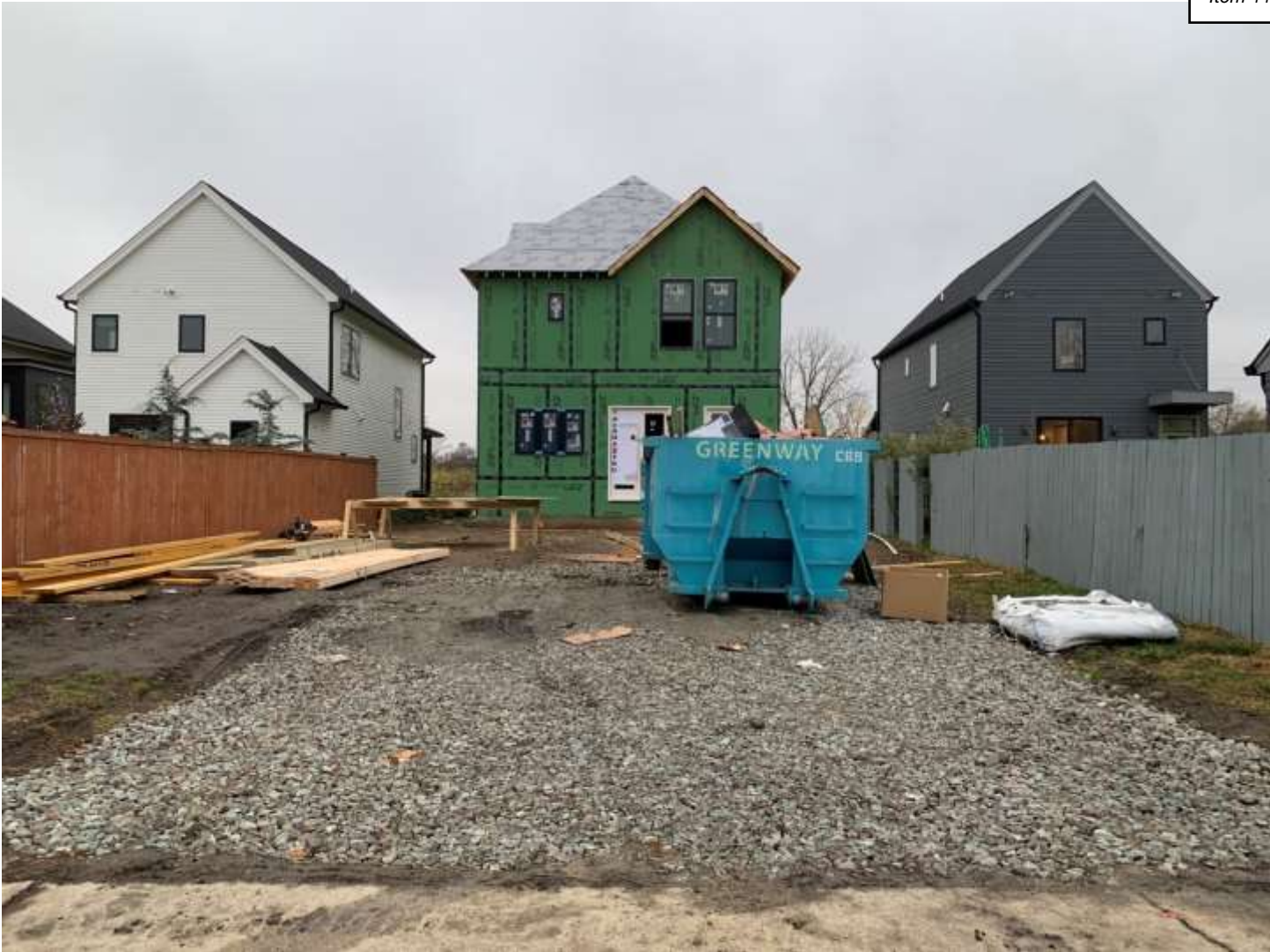
Subject site rear yard viewed from the alley
